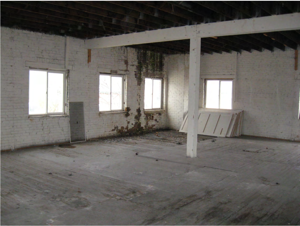
Floor 3 North current view
