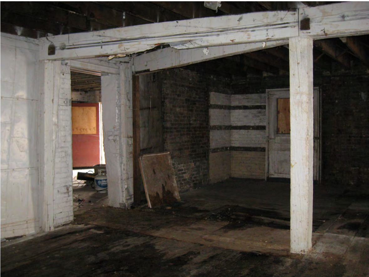
Floor 1 South current view
