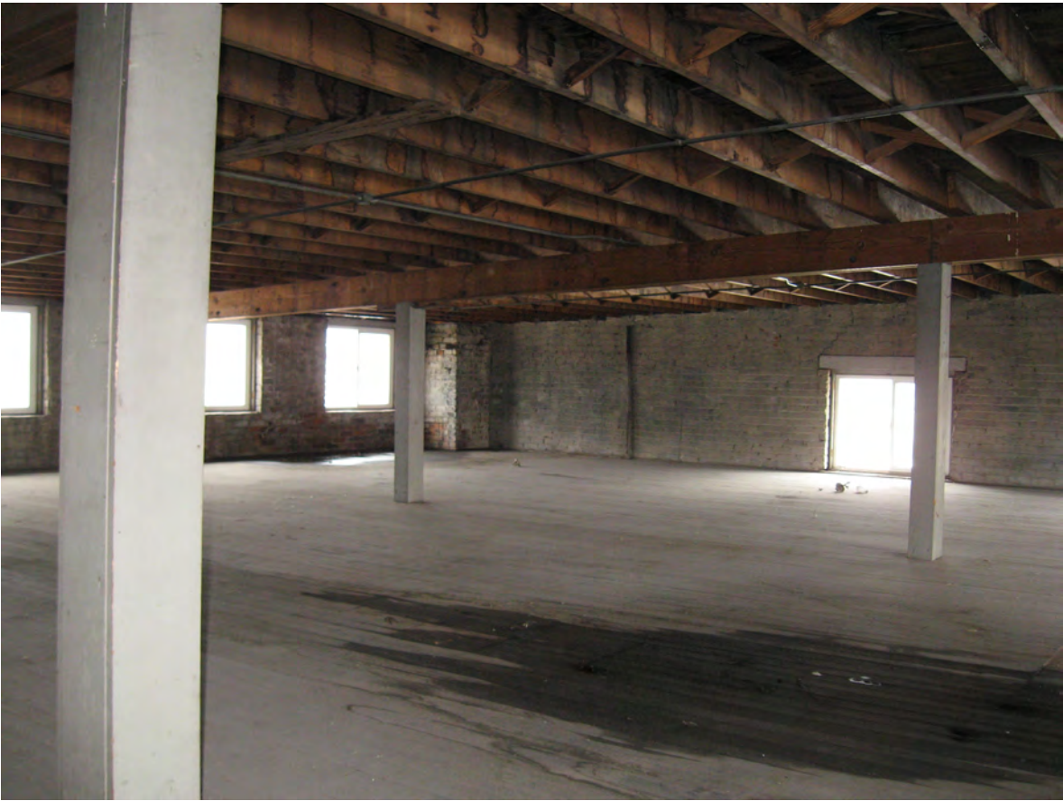
Floor 4 North current view
