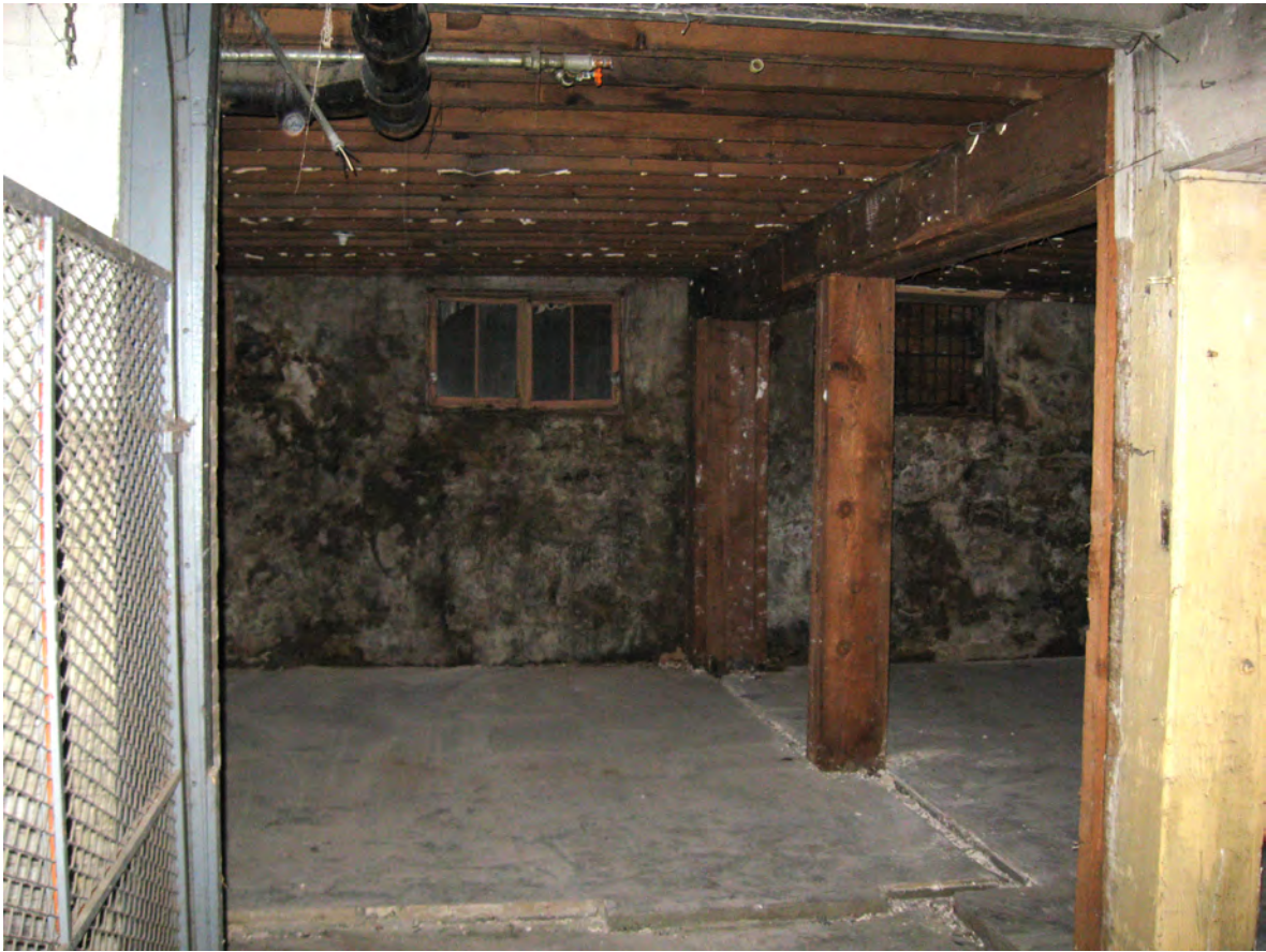
Basement North current view
