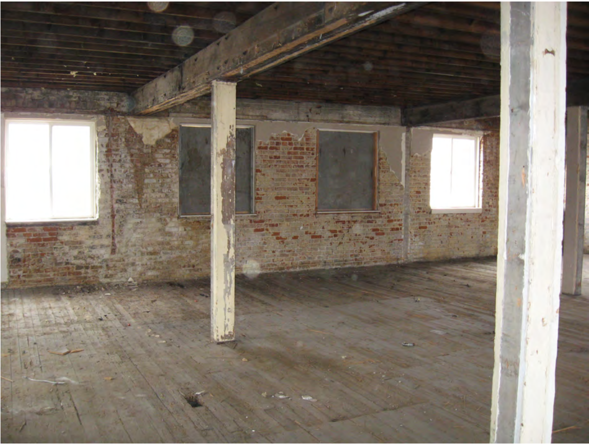
Floor 2 North current view
