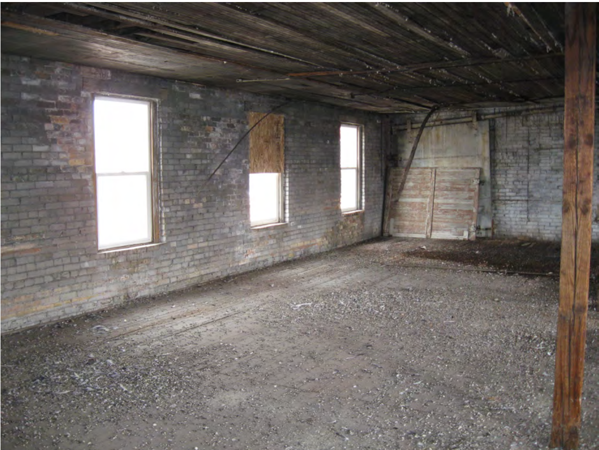
Floor 3 South current view
