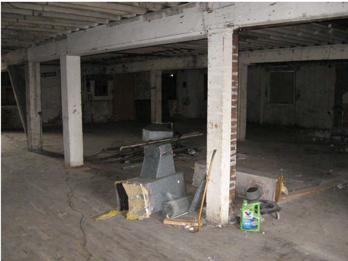
Floor 1 North current view
