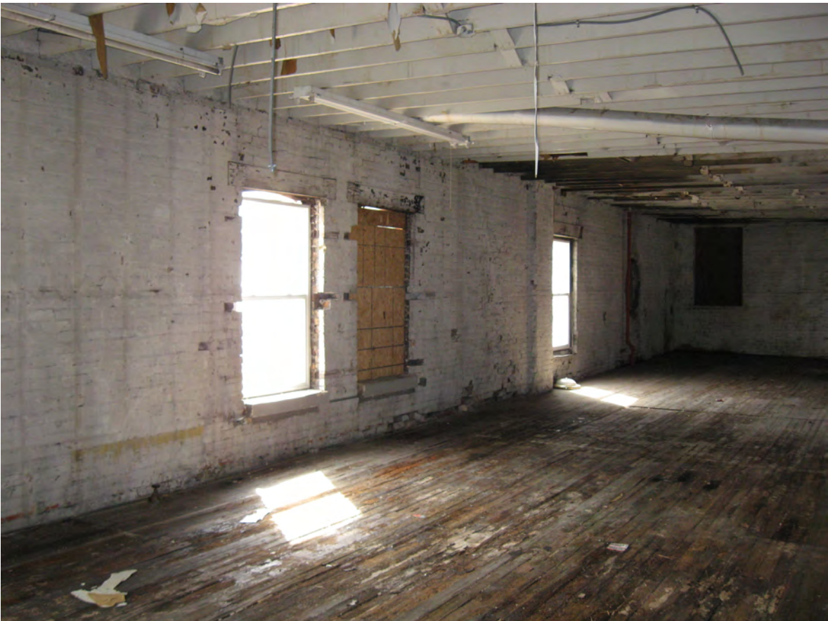
Floor 2 South current view
