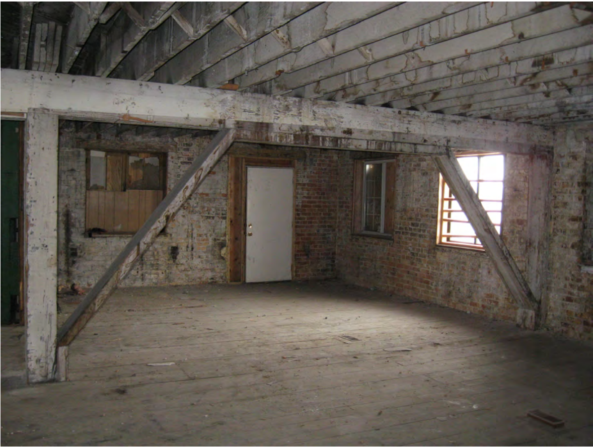
Floor 1 North historic press location current view
