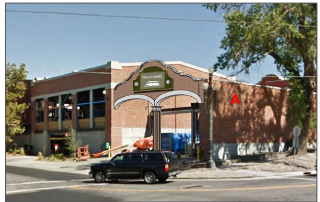
An arched wall would need to be constructed to connect the wall along 600 South with the building on 600 East to house the proposed sign. A final determination on the sign type would need to be made by the zoning administrator.
