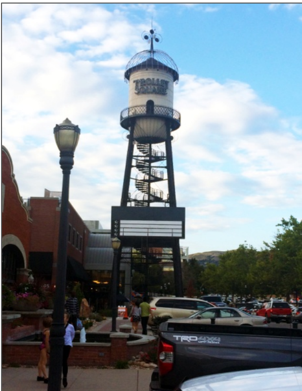
Existing Non Conforming Internally Illuminated Changeable Copy
