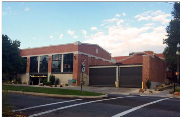
Photo above shows the existing conditions near the loading dock on the corner of 600 East and 600 South.
