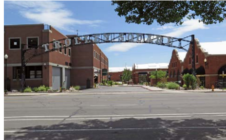
pole sign (pad site A)
