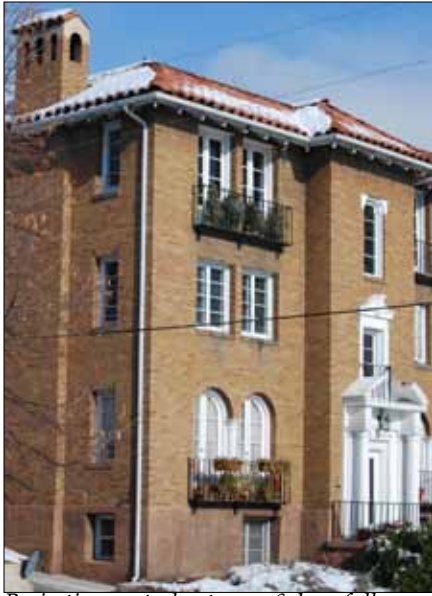
Projecting central entrance & bay, full height chimney & vertically proportioned & window sequence create strong verticality.
