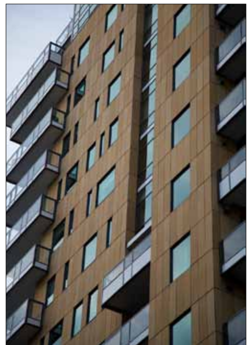
Projecting balcony arrangements, a varied fenestration pattern and window reveals embellish a terracotta panelled facade, helping to reduce apparent scale and creating architectural interest.
