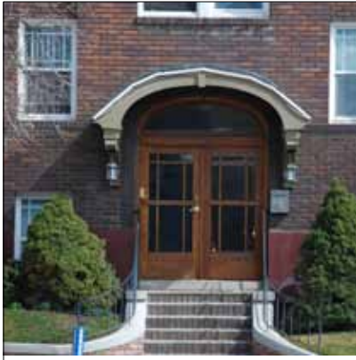
The public entrance designed as the focal point of this street frontage.
