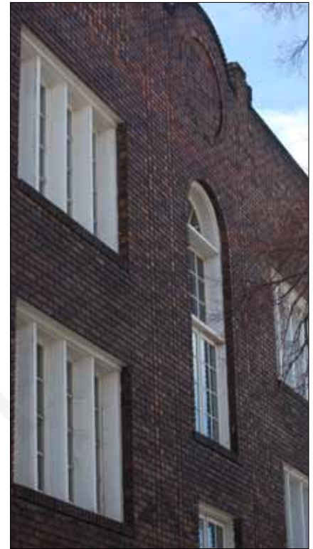
Window reveals and subdivision contrast with the dark brickwork of the facade wall.
