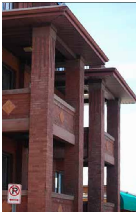
Well defined and detailed projecting balconies help to establish building form and scale.
