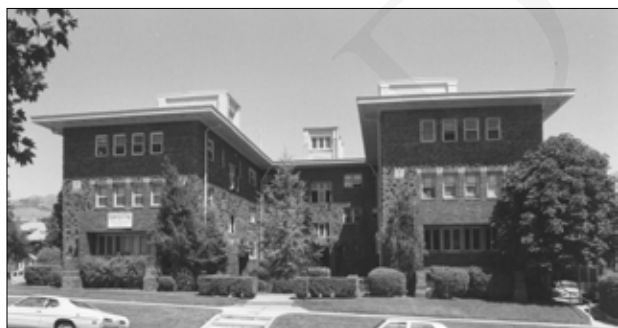
Caithness Apartments, 1908, Ware and Treganza, Architects, Salt Lake City, Salt Lake County. A “U” court design influenced by the Arts and Crafts and Prairie School styles, it originally featured an extensive roof garden.
