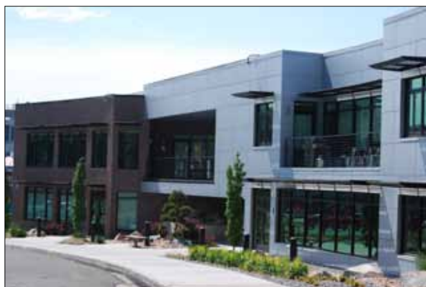
A contrast in facade design and materials, and the modeling of the facade can help to break down lateral scale while enhancing visual interest and presence of the building.
