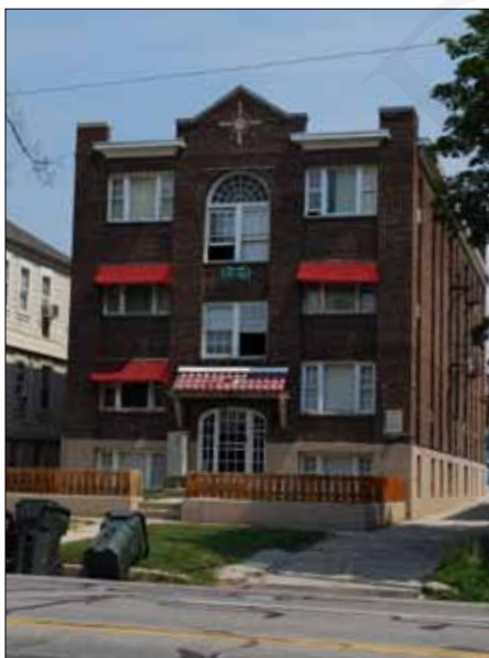
Central approach, entrance and axial 'pedimented' bay help to enhance the focused contribution to the street.
