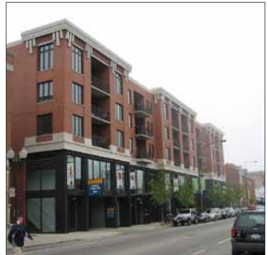
The primary modeling of the street facade to create a symmetrical arrangement of three projecting bays, is supplemented by alternating recessed and projecting tiers of balconies.
