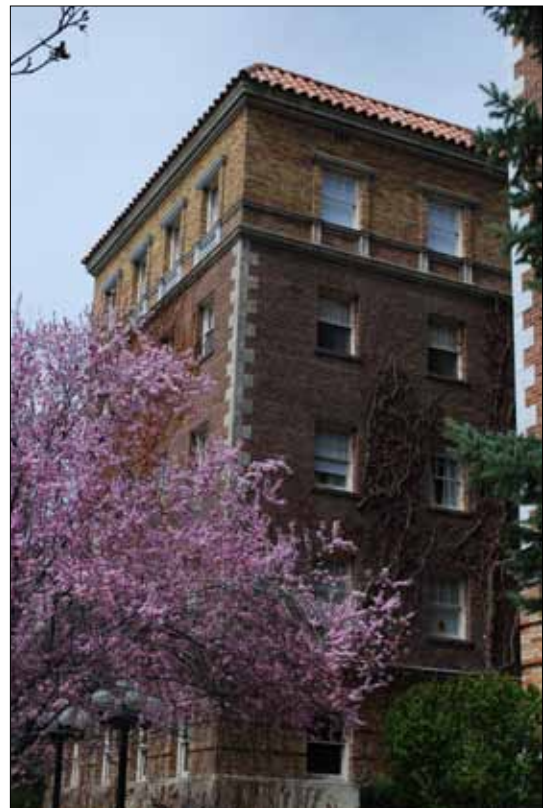
A recessed front courtyard can enhance both building character and public streetscape.
