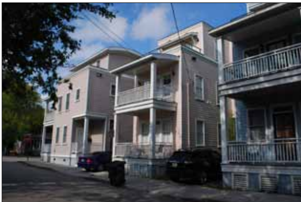
Limiting street facade sheer height and the projecting balconies reinforce a sense of human scale.
