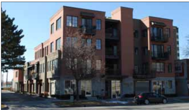
The vertical elements of the primary facade are echoed in the modeling of the secondary facade.
