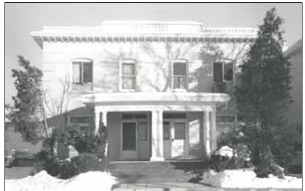
Four-Unit block, c. 1905, Salt Lake City, Salt Lake County. This elegantly proportioned, four-unit block of brick masonry has brick quoins and cornice with dentils below a short parapet. A portico of paired Tuscan columns projects the double entry to the building.
