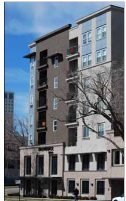
A recessed or projecting balcony sequence can be employed to help articulate the facade design.
