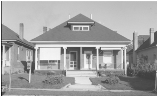
Double-House bungalow, c. 1910, Salt Lake City, Salt Lake County. In this example the privacy of the two units is reinforced by a brick wall that projects onto the front porch, which is supported by under-scaled columns of the Ionic order.
