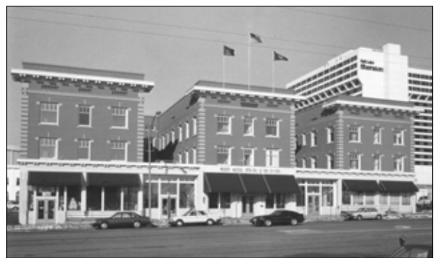
Peery Hotel, c. 1910, Charles Onderdonck, architect, Salt Lake City, Salt Lake County. This example of the “E” or Double Court was built for Ogden Businessmen David and Joseph Peery.
