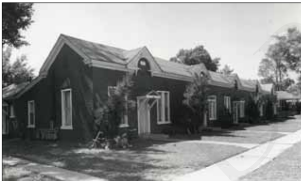
Silver Row, c. 1890, Provo, Utah County. This brick row house, highlighted by a decorative gable over each entry, was owned and rented out by David Felt, a Provo publisher and printer.
