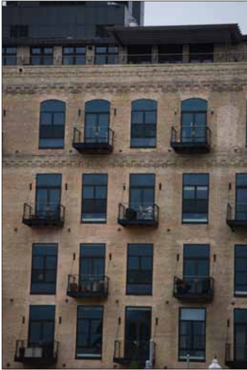
The recent addition of individual alternating projecting balconies has been used effectively to redefine and articulate the character and interest of the facade.
