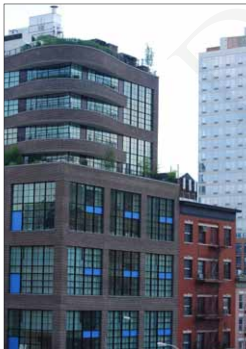
Window design can provide both unity and architectural detail.
