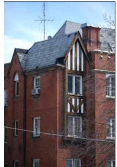
A vertical, gabled corner accent framed by projecting front facade, secondary side gable and rising chimney stack.
