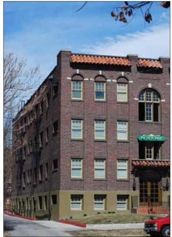
The street facade is designed around a central entrance and stairway, while placement allows access to parking to the rear.
