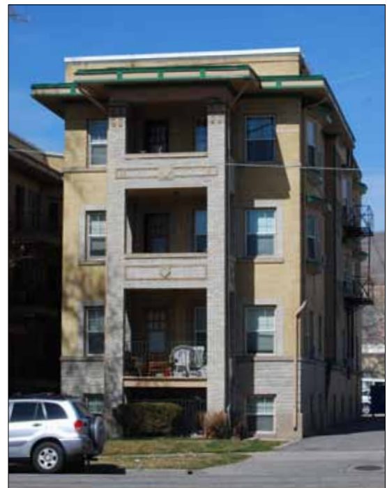
A principal projecting wing of the street facade, combined with projecting balconies, can effectively maintain a distinct human scale in a much larger building.
