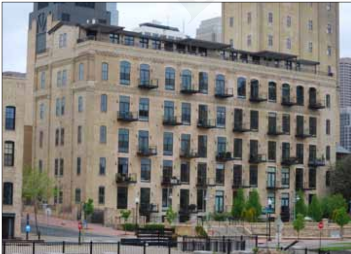
The addition of the alternating projecting steel balconies introduces an intricate horizontality which in turn helps to reduce the apparent scale of the building.
