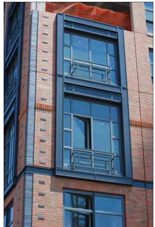
New construction using dark metal framed vertical window bays set within a complimentary decorative brickwork detail.
