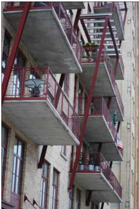
Window proportion and detailing are accentuated by rising, projecting balcony tiers and their decorative structural ironwork.
