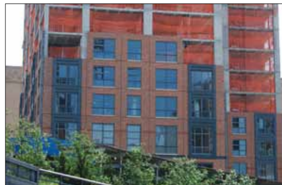
Contrasting dark vertical window bays frame subtly vertical fenestration pattern in this brick facade.
