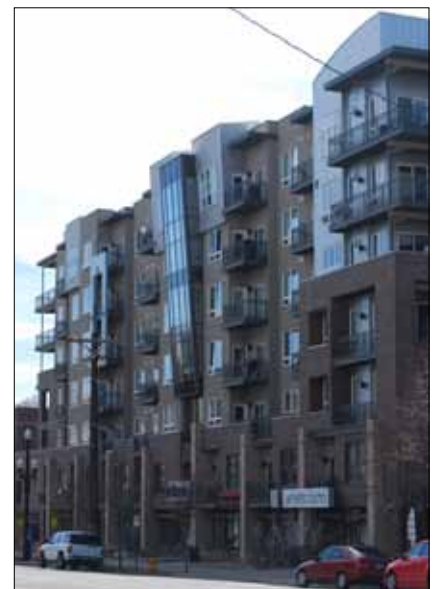
Facade articulation in a series of vertical projecting bays and balconies help to soften and reduce the visual scale of the building.
