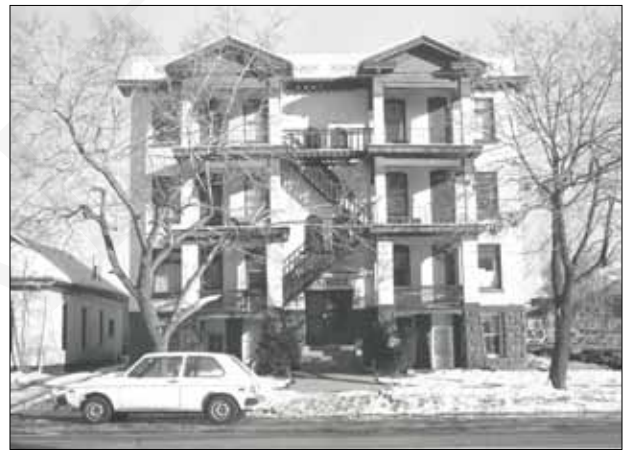
Rainer Apartments, c. 1900, Salt Lake City, Salt Lake County. The raised basement of this building helps create a sense of vertically characteristic of this apartment type.
