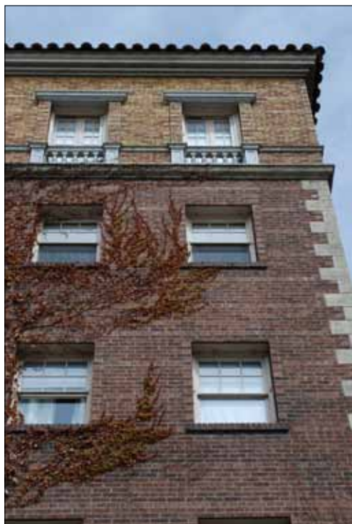
A palette of brick, stone, tile and wood are chosen and detailed to establish both architectural stature and elegance.
