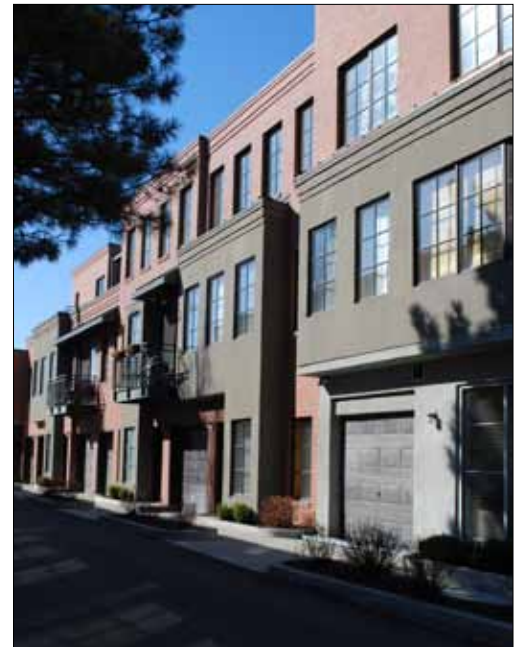
Design articulations, fenestration patterns, materials and their detailing, frame balcony spaces, doors and garage entries in a varied and interesting street facade sequence.
