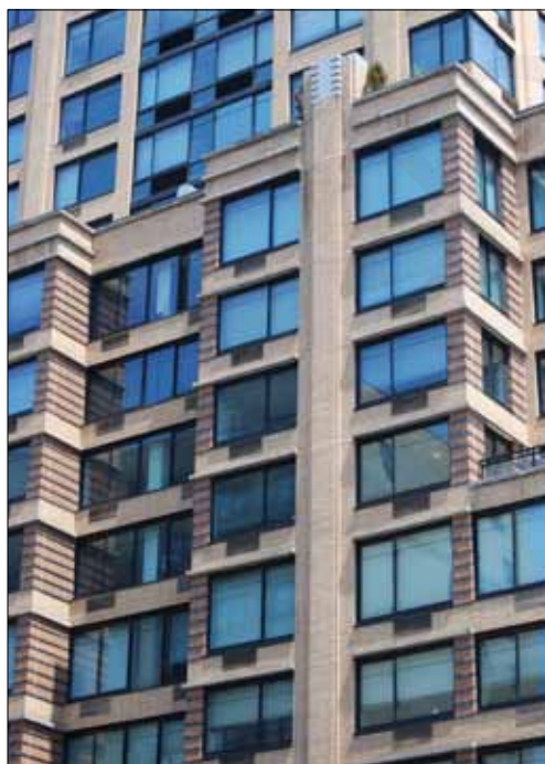
Brickwork employed as a decorative expression of architectural style, and effectively conveying a sense of human scale within a very tall building.
