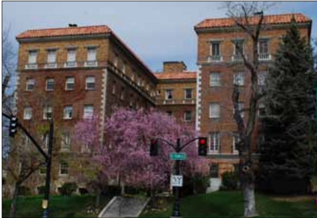
Classic historic apartment plan with two wings to frame a deep recessed and landscaped courtyard.
