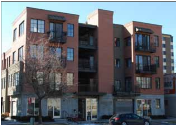
Primary street facade composed of two individual projecting bays framing a central projecting elevator tower and two recessed bays, enriched by rising projecting balcony sequence and varied fenestration an intricate, rather 'organic' relationship.
