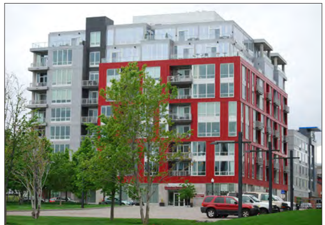
Balconies, modelling, varied fenestration, stepped back upper floors and color, employed in composition to reduce the apparent scale.
