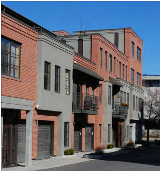
The sequence of small garage doors woven into the intricate articulation of this secondary facade creates a more pedestrian-friendly character.
