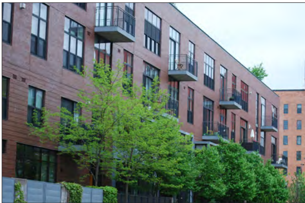
The solid to void ratio and a repeating fenestration pattern create a sense of human scale and visual interest in an otherwise relatively simple brick facade.
