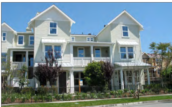
Gabled full height wings frame recessed floors and balcony space creating a strong sense of human scale and visual interest.
