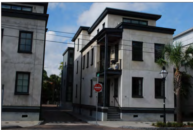
Fenestration pattern and proportions compliment the proportion of the street facades.
