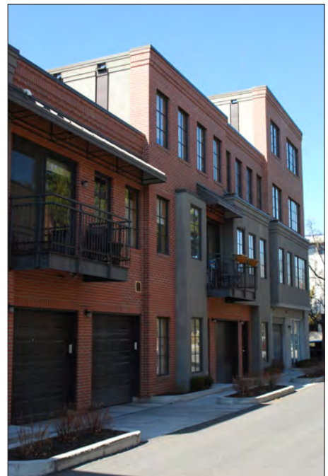
Stepping down the height of the street facade introduces a more intimate scale and terraced private space to the rear.
