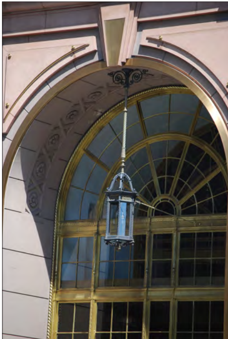
A single decorative pendant light fitting can enhance architectural character when not in use.
