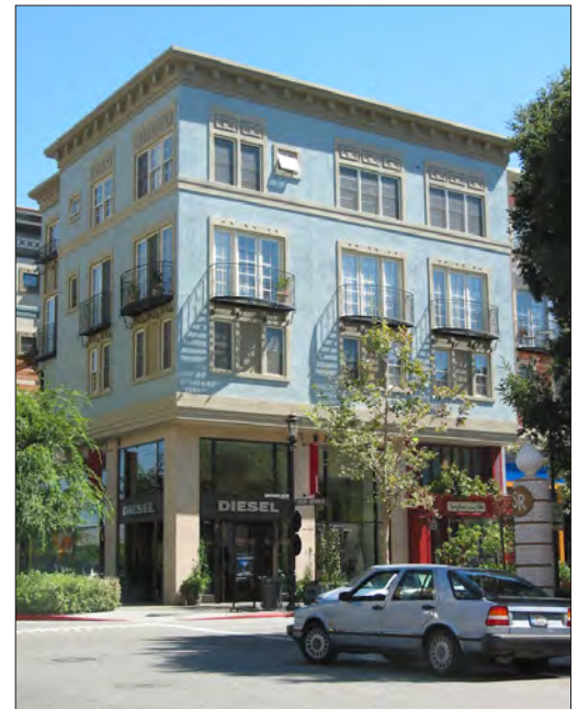
Window design and detailing here helps to identify the building's primary entrance on the corner.
