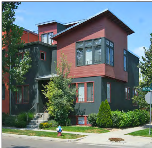
The interplay of architectural forms and varied massing can retain a sense of human scale and achieve a visual strength on the corner.
