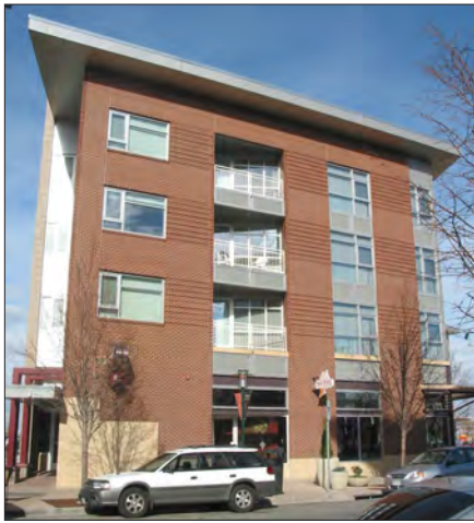
Vertical bays capped by a strong projecting cornice and deep eaves.
