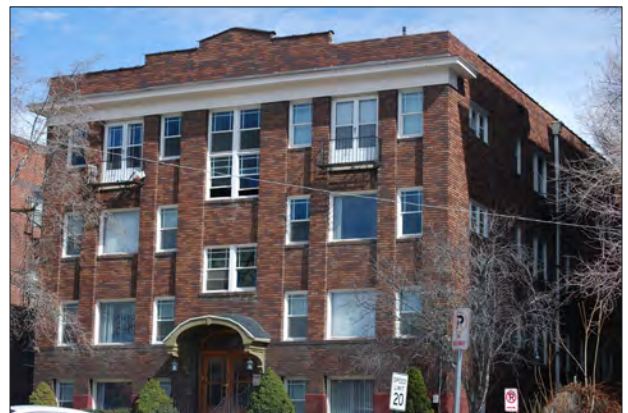
Symmetrical facade composition around a central entrance helps to reduce the sense of scale.
