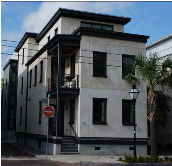
Massing of the building stepping back the street and the side facades, with corner balcony and fenestration, creates a vertical proportion and a human scale street facade.
