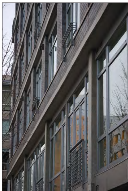
Window design can provide both unity and architectural detail.
