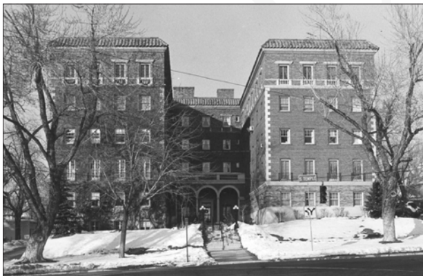
Mayflower Apartments, 1927, Slack Winburn, architect, Salt Lake City, Salt Lake County. A vertical “H” apartment block complete with attached parking structure, the Mayflower was built by and for the Bowers Building Company
