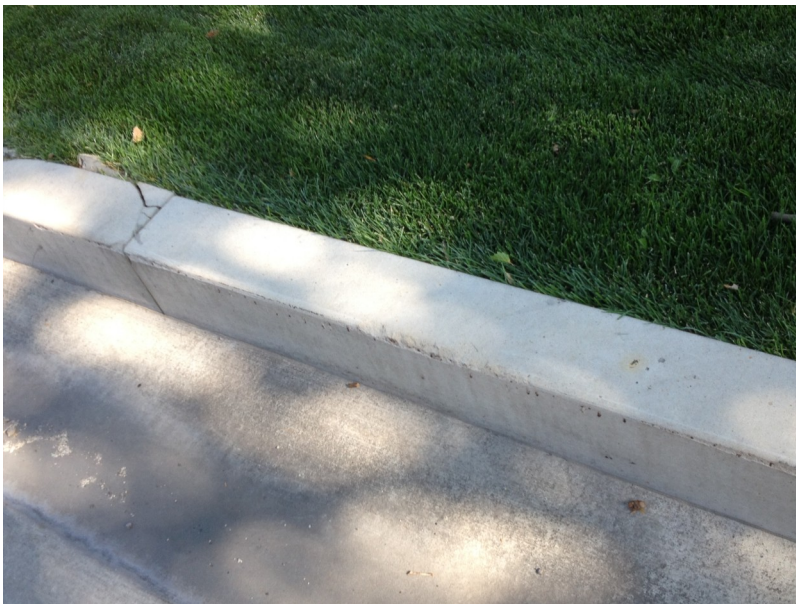
Limestone curb mostly intact
