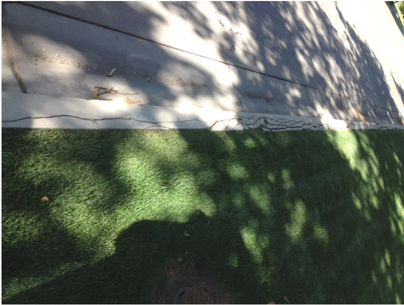
Limestone curb in front of 550 East South Temple
