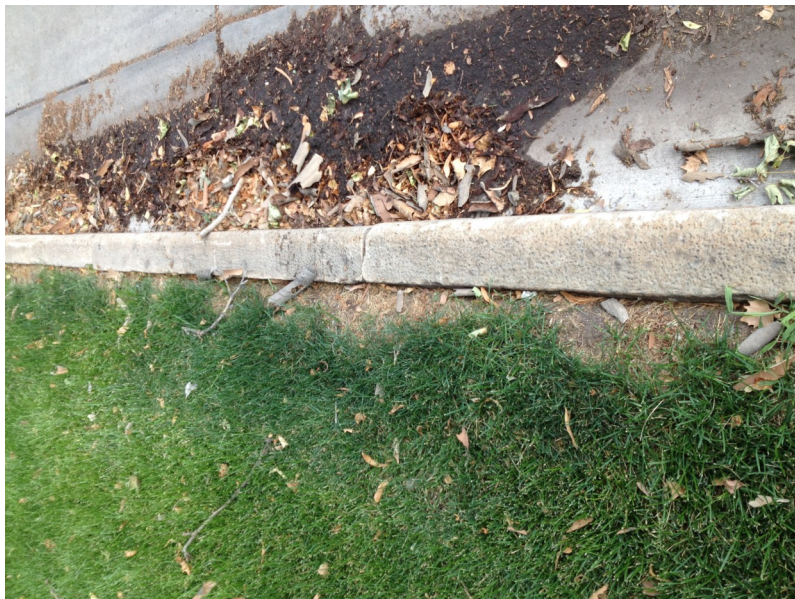
Original sandstone curb
