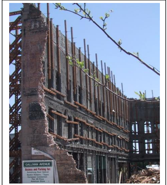
Photos of demolition (only two walls remaining)
