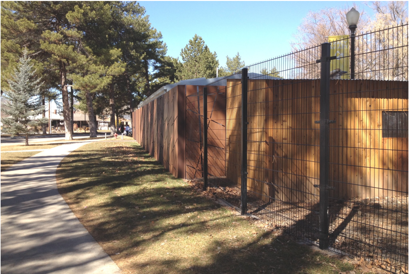
HOLDINGS BUILDING - View looking West
