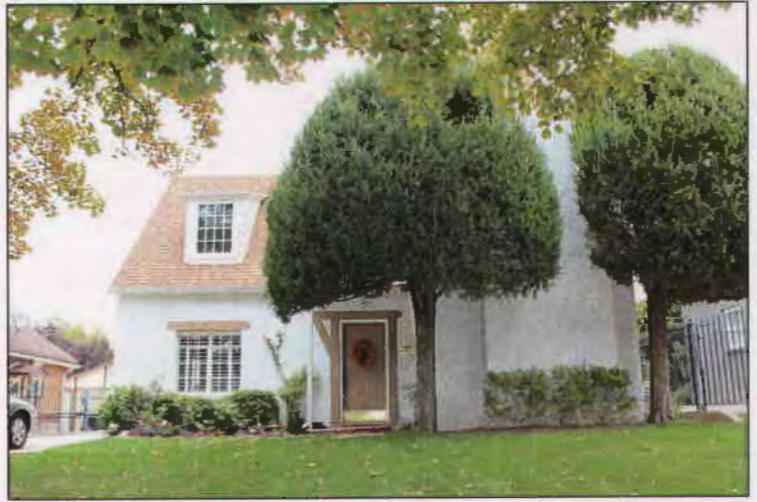
1775 Herbert Ave. Built 1936 Regular brick English Cottage
