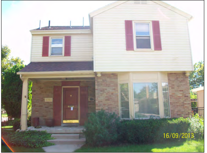
1786 E. Princeton Ave. Colonial Revival c. 1940
