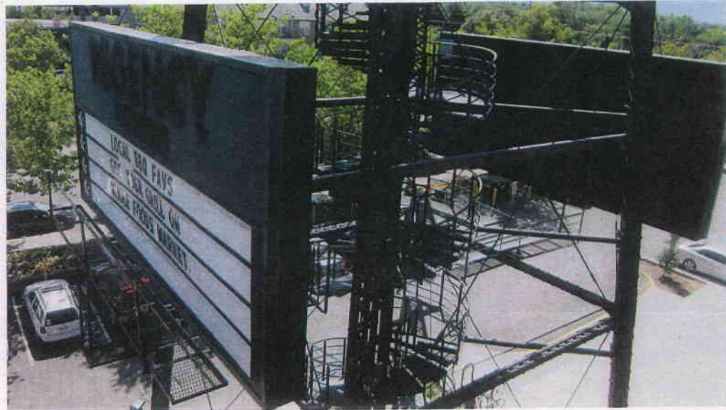
2014 Damaged and Disfigured Signs
