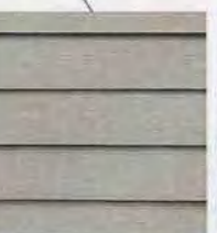
LAP SIDING Material: Fiber Cement 'Smooth' Color: 2844 ROYAL ROY MUST GRAY SHERWIN-WILLIAMS
