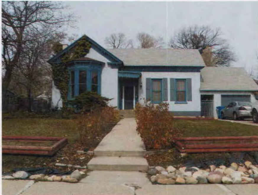
Front of 323 E. 2 nd Avenue prior to modifications
