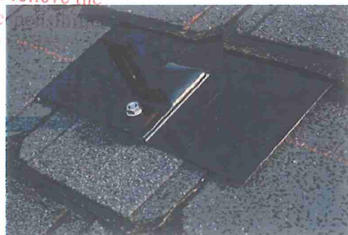
FLASHING DETAIL
