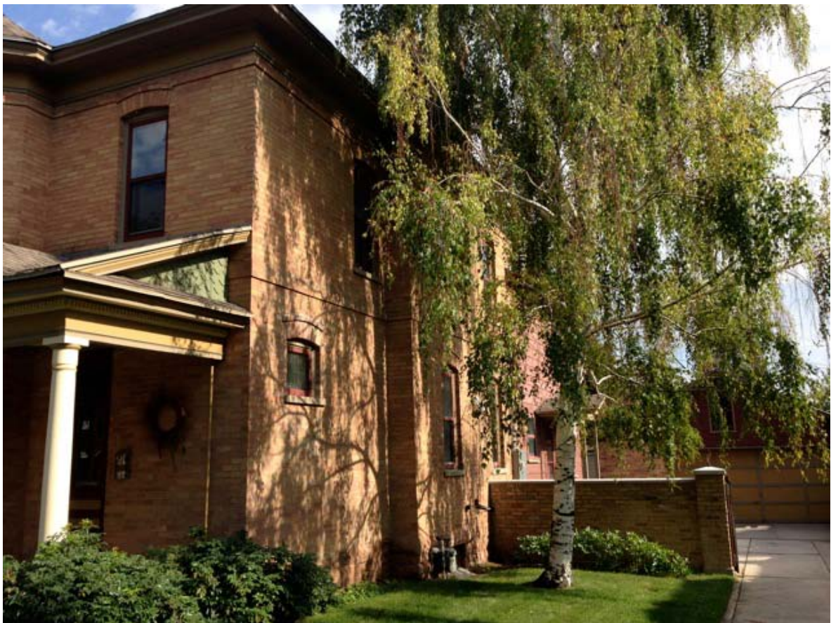
Area of porch expansion
