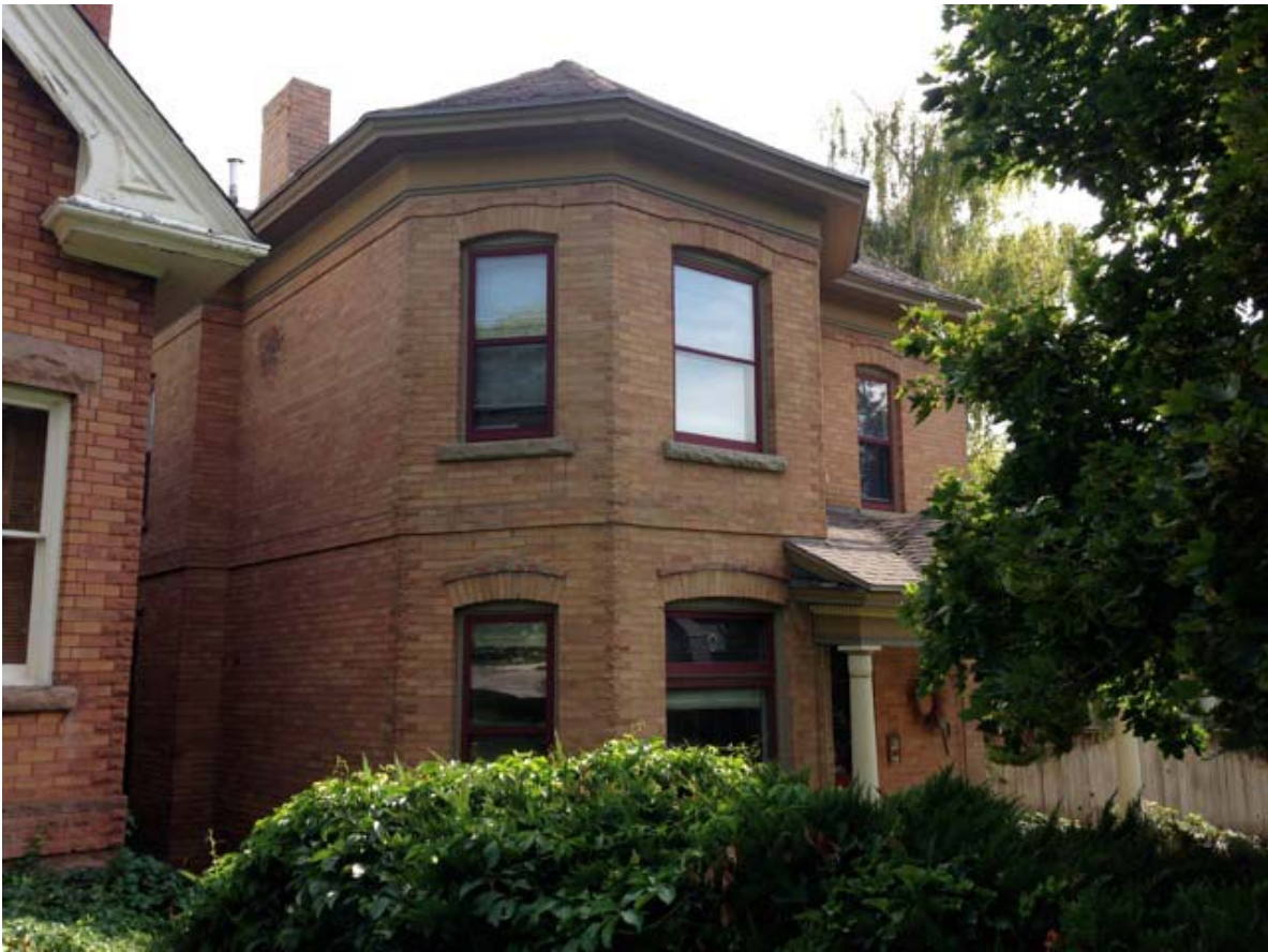
East side view of front of residence
