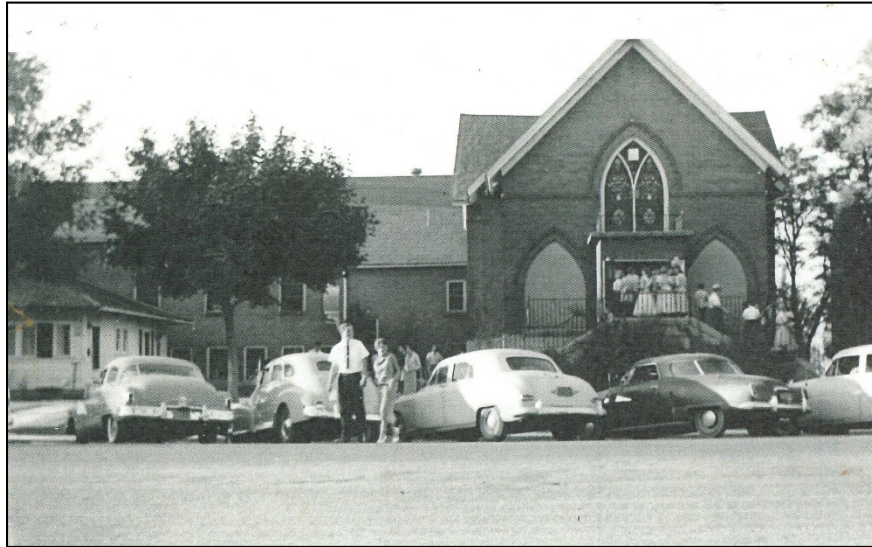
Figure 3 Twenty-Ninth Ward LDS Meetinghouse, circa 1959. Camera facing north.
