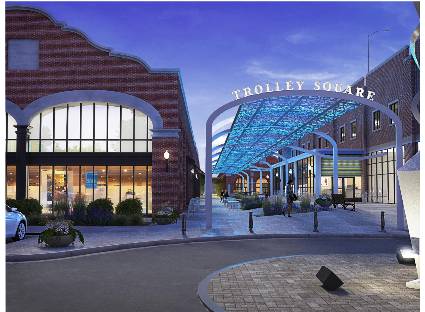
RENDERING OF DROP OFF AREA AND CANOPY BETWEEN BUILDING D AND BUILDING C
