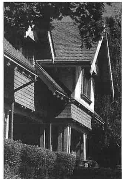
Gables, deep eave profiles & rafter tails are key elements of the design.
