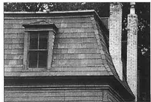
Natural slate is rare in the city and is the most durable of traditional roof materials, usually requiring only piecemeal replacement of damaged individual slates.
