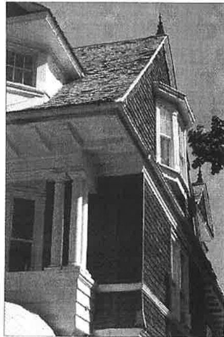
Wood shingles help to unify both walls and roofscape, creating visual texture as a background to Classical detail.
