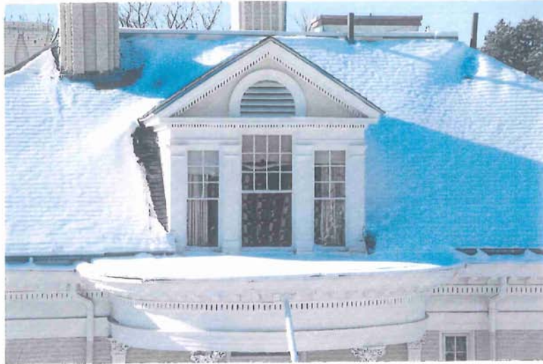
EAST ATTIC DORMER
