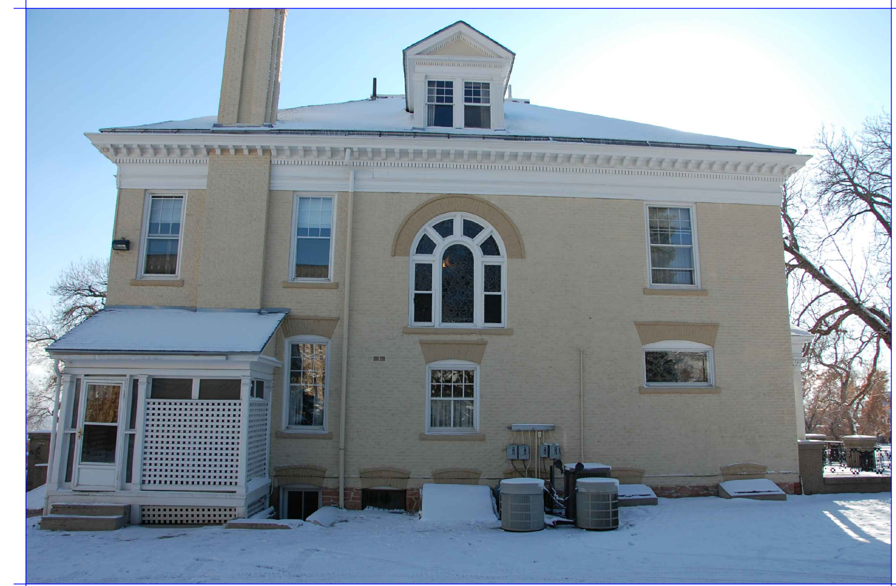
259 Seventh Avenue 'North Elevation'
