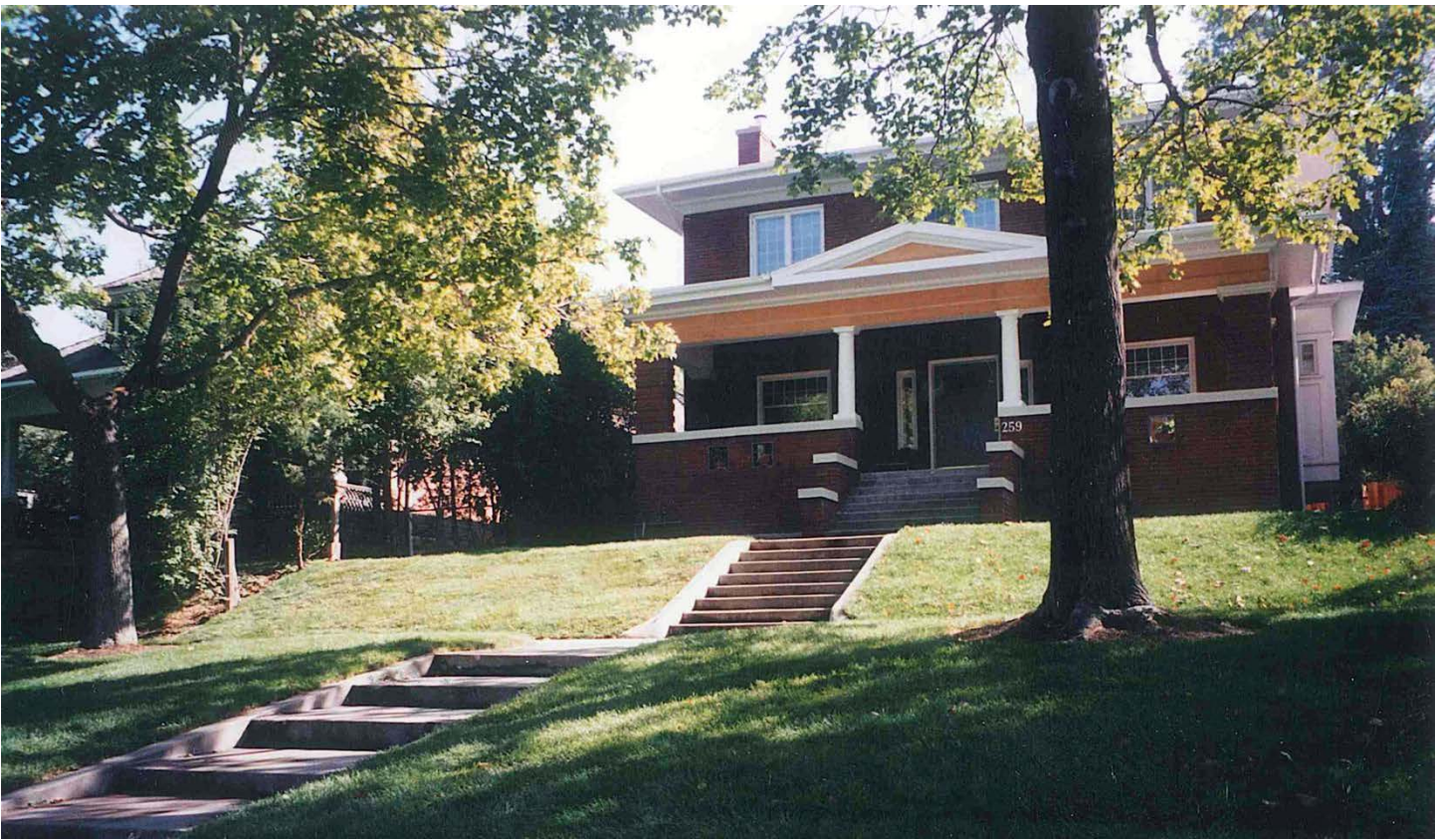
East View of the subject property from 1200 East. Photo submitted with the application prior to unauthorized grading of the front yard. Proposed terraced retaining wall would be located in the front yard area at the base of the stairs and step up to a point in line with the top of the staircase. Two pillars with cement caps are proposed to match the design of the front porch as closely as possible.
