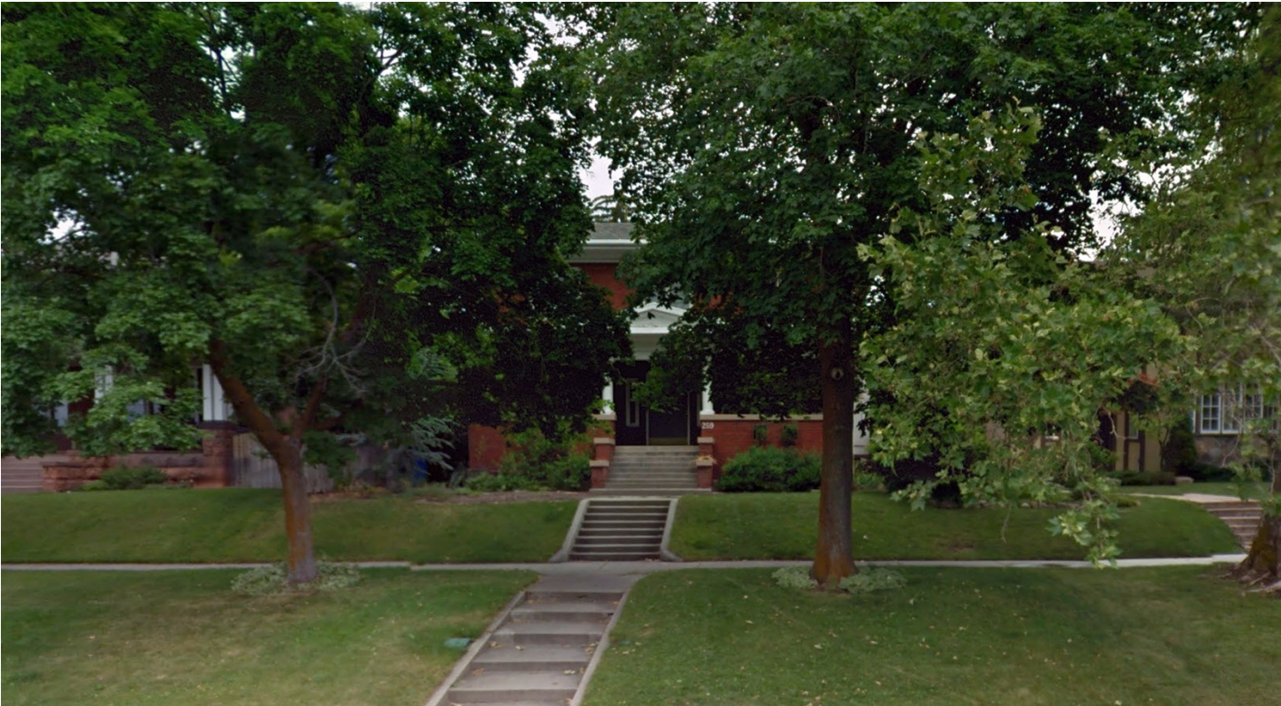
East View of the subject property from 1200 East.
