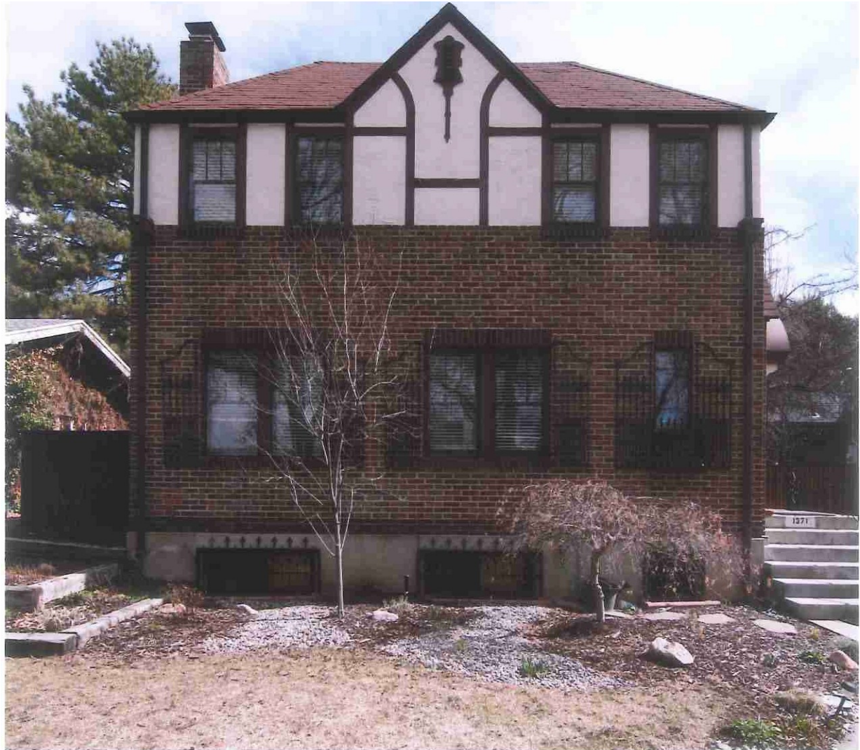
Existing West Façade (Block View)
