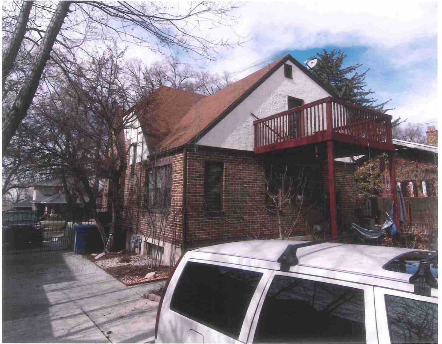
Existing South East Façade
