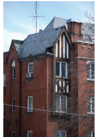
A vertical, gabled corner accent framed by projecting front facade, secondary side gable and rising chimney stack.
