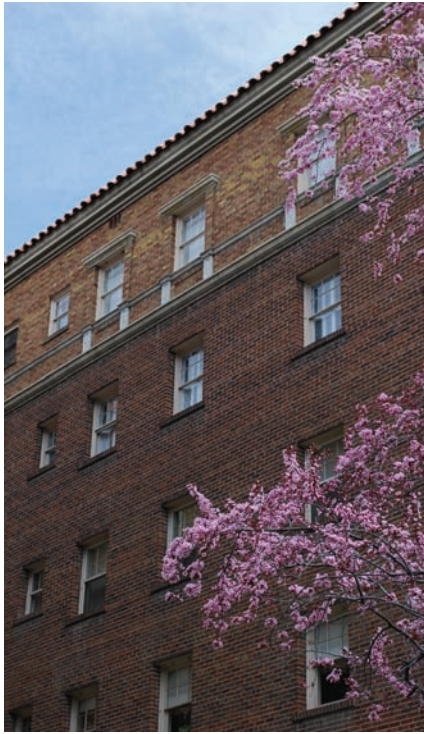
Window proportion and grouping in this brick and stone facade create subtle pattern and relationship.
