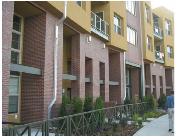
Deeply recessed windows and doors on lower floors create a strong sculptural base for the articulation of the facade above.
