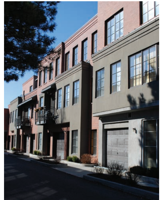
Design articulations, fenestration patterns, materials and their detailing, frame balcony spaces, doors and garage entries in a varied and interesting street facade sequence.
