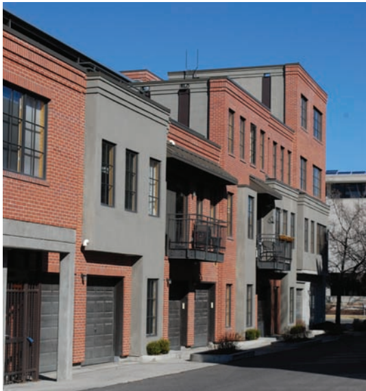
The sequence of small garage doors woven into the intricate articulation of this secondary facade creates a pedestrian-friendly character.
