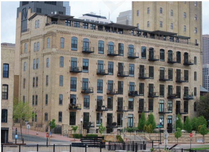
The addition of the alternating projecting steel balconies introduces an intricate horizontality which helps to reduce apparent scale.
