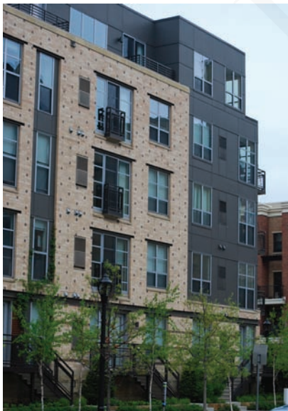
Fenestration pattern in light colored brickwork framed by dark panelling organized around vertical proportion.
