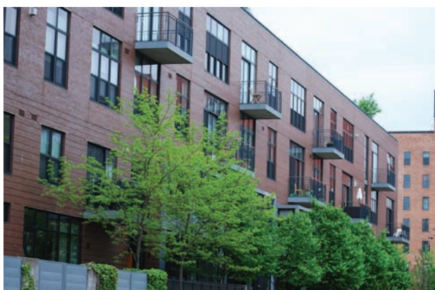
The solid to void ratio and a repeating fenestration pattern create a sense of human scale and visual interest in an otherwise relatively simple brick facade.
