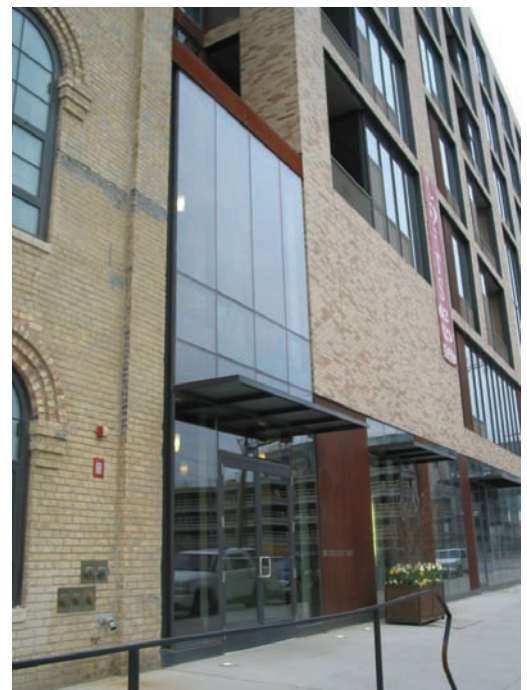
Historic brickwork provides the inspiration for the use of complimentary brick as the principal material for recent construction.
