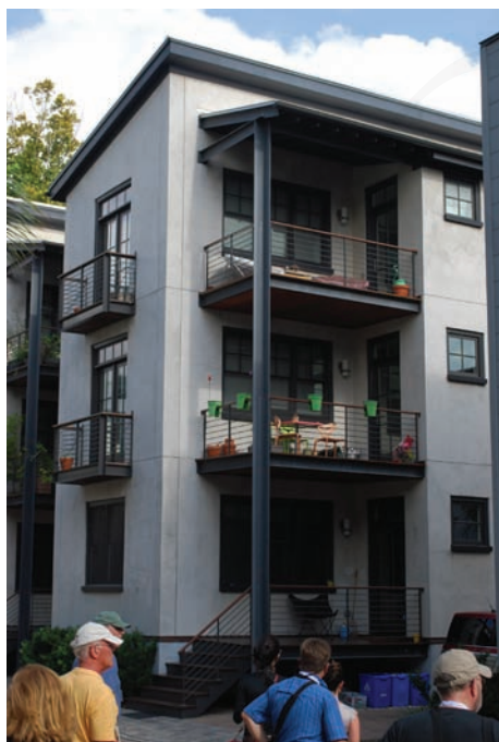
The design of a projecting balcony arrangement should still provide the opportunity for architectural creativity.
