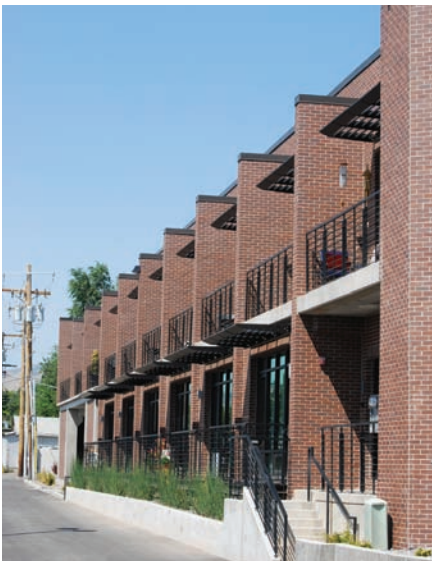
A linear sequence of units stepping back to create strongly framed private balcony space above.
