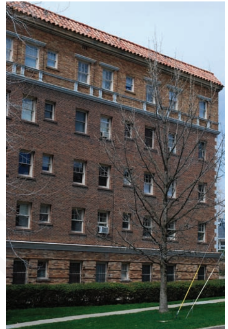
Differentiation in the design of the first floor and the top floor and tiled roof helps to reduce perceived height.
