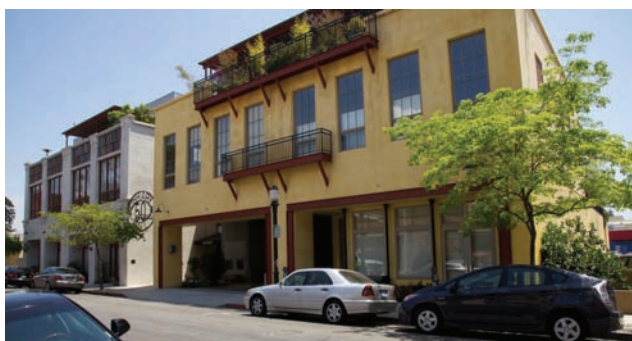
Building scale and the alignment and proportion of openings create an affinity in different facade designs.
