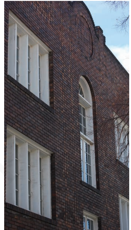
Window reveals and subdivision contrast with the dark brickwork of the facade wall.
