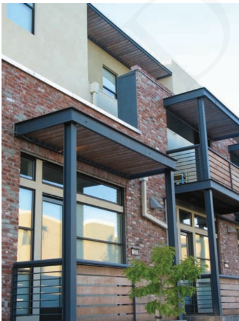
Porch and balcony design and detailing can play a major role in the articulation of the facade and in defining private outdoor space.
