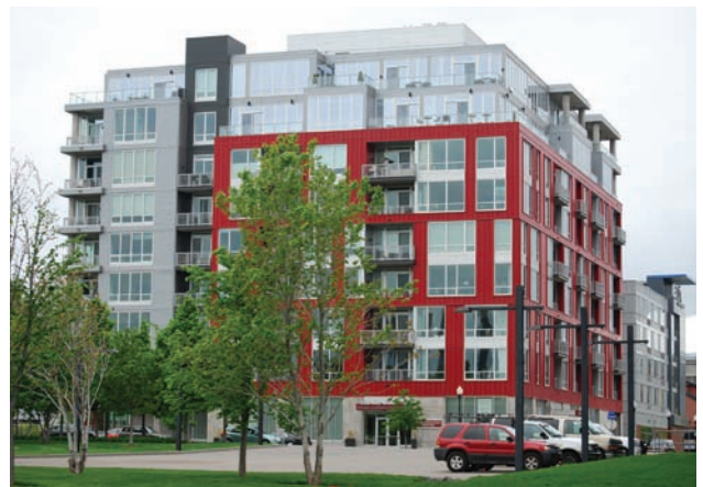
Balconies, modelling, varied fenestration, stepped back upper floors and color, employed to reduce apparent scale.
