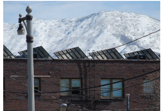
Building utility locations can have unanticipated consequences.
