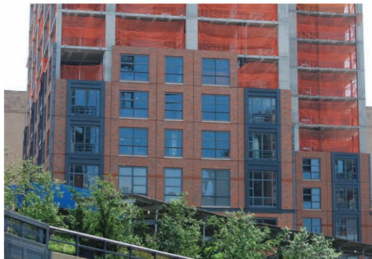
Contrasting dark vertical window bays frame subtly vertical fenestration pattern in this brick facade.
