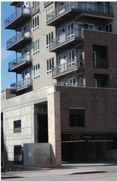
Utility equipment can be discreetly planned and designed.
