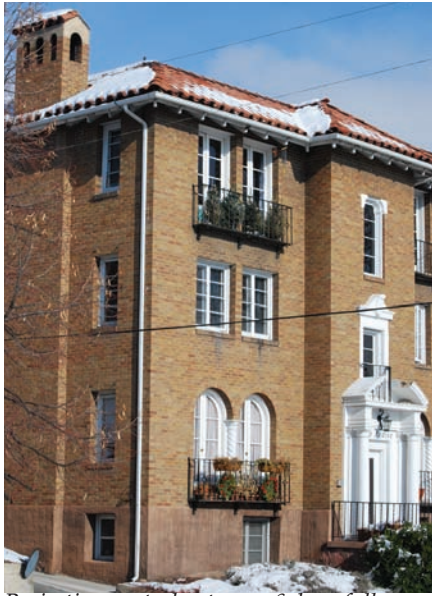
Projecting central entrance & bay, full height chimney & vertically proportioned & window sequence create strong verticality.
