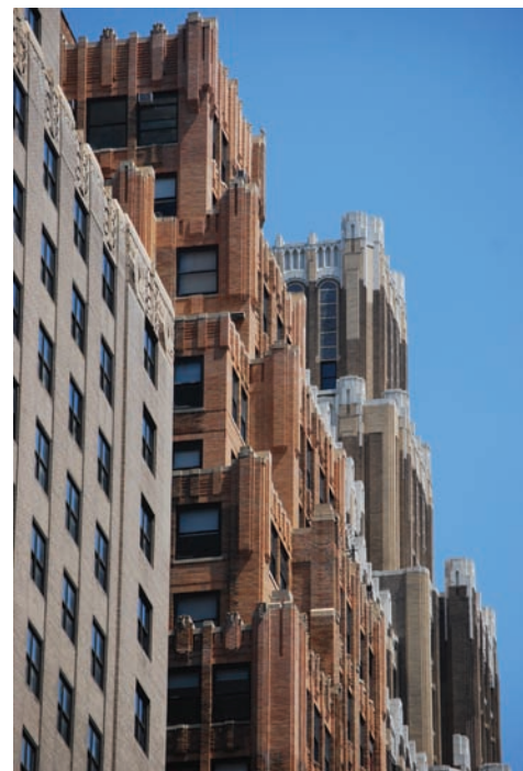
Contrasting fenestration providing 'hole in the wall' definition in one facade, and framed by decorative sculptural brickwork in others.
