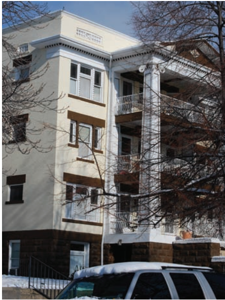
Central balcony portico, cornice, raised first floor and foundation, and fenestration coincide to reduce the apparent height.
