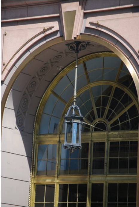
A single decorative pendant light fitting can enhance during daytime.
