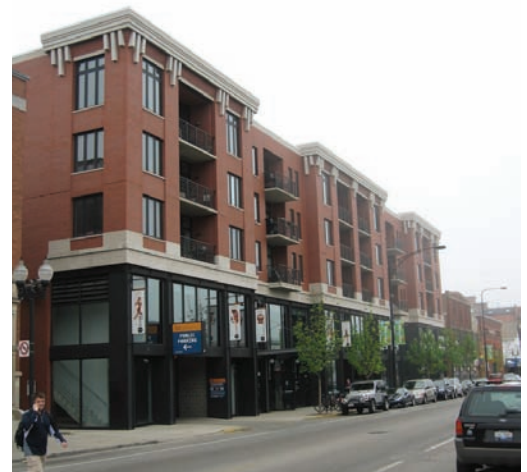
The primary modeling of the street facade to create a symmetrical arrangement of three projecting bays, is supplemented by alternating recessed and projecting tiers of balconies.
