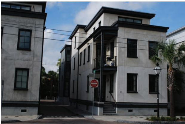
Fenestration pattern and proportions compliment those of the street facades.
