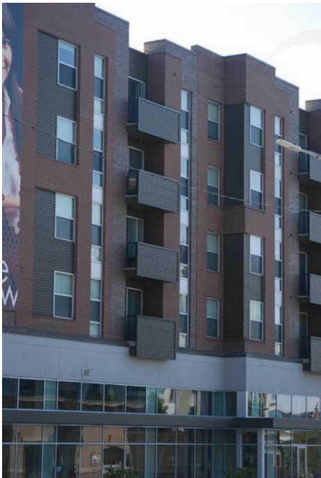
Articulation of the street facade using varied planes, materials and parapet profiles, contrasts strongly with the design of the commercial first floor.
