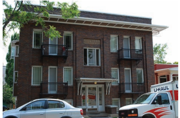
Symmetry and vertical emphasis can effectively enhance a sense of both human scale and architectural stature.
