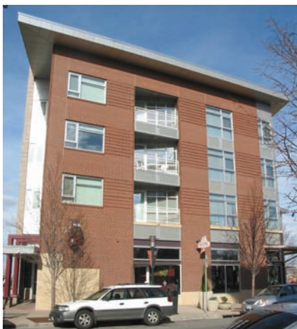
Vertical bays capped by a deep projecting cornice.
