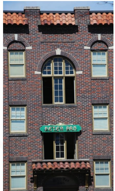
The considered detail inherent in the brick and tile work, as well as the window designs, create a vibrant street facade.
