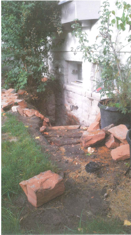
TOP OF STAIRWAY TO BASEMENT
