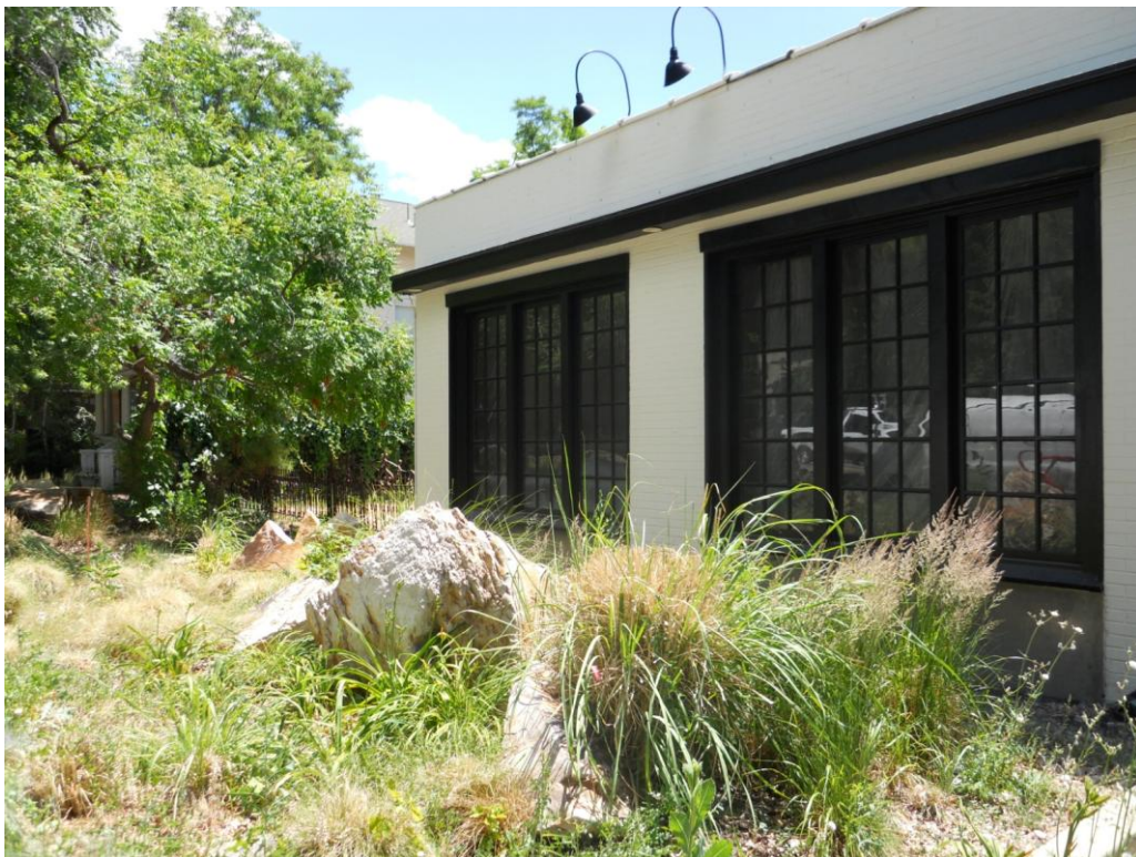
Close up of the front or north face of the building.
