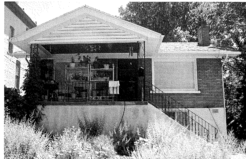
EXAMPLES OF RETAINING WALLS AND CONCRETE
