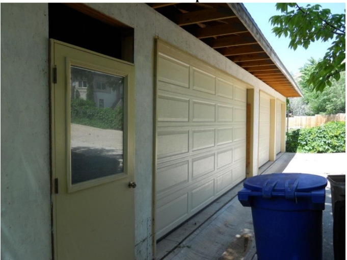
Entryway to Garage
