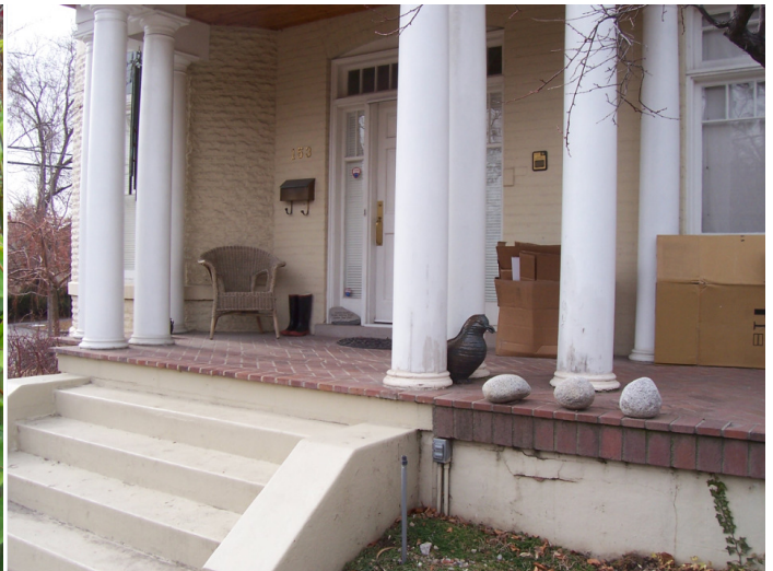
View of Elevated Porch
