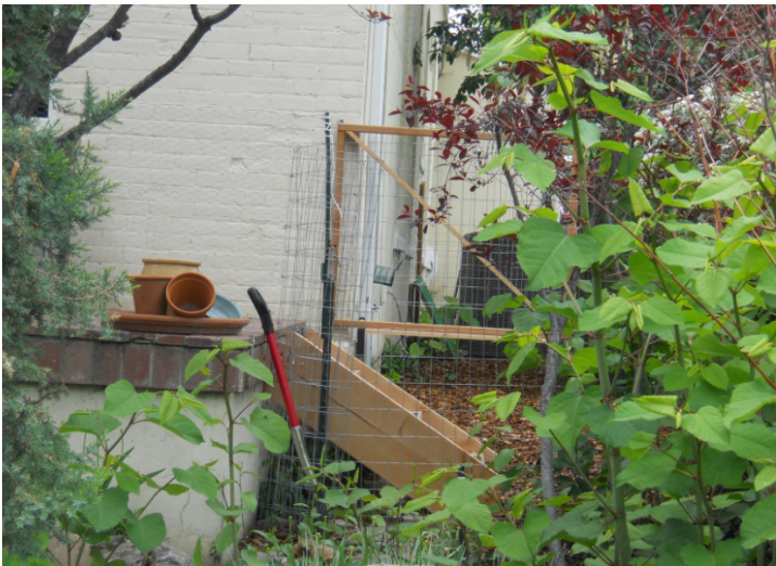
Steps Constructed off of Porch
