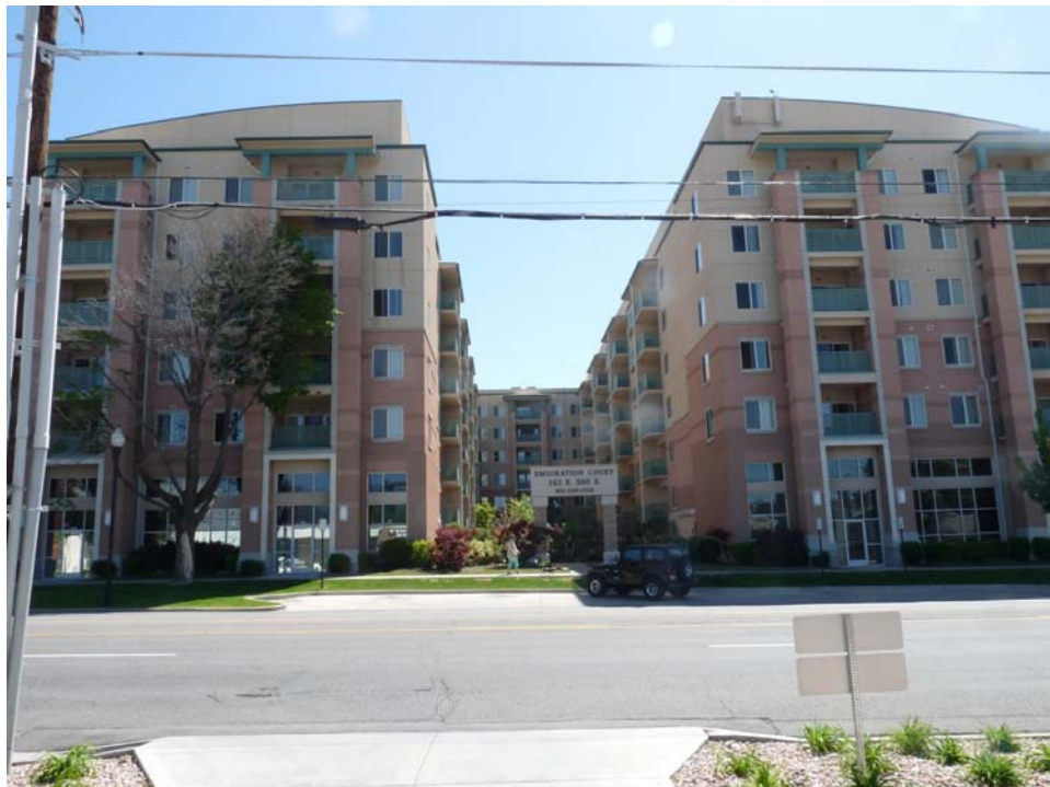
Emigration Court (east side of 500 East) – approximately 80 feet tall along 500 East
