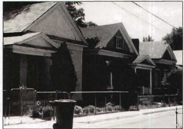
Orienting the entry to the street is preferred. Establishing a "progression" of entry elements, including a walkway, landscaped elements and porch also is encouraged.
