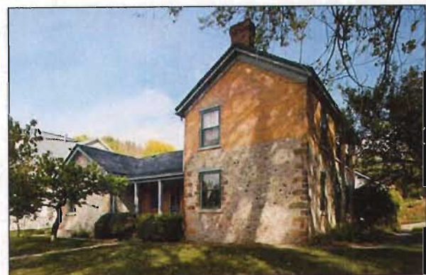
The addition here takes the form of a new single story wing to the left of the two story earlier building, itself with an early addition of the second floor.
