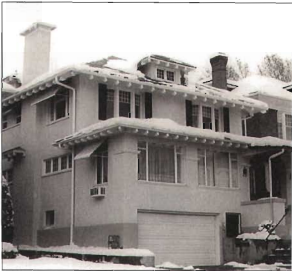
Due to the large size of many of the buildings in the district, roof materials are very important visual features.
