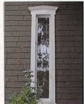
Ornamental trim around historic windows should be preserved.
