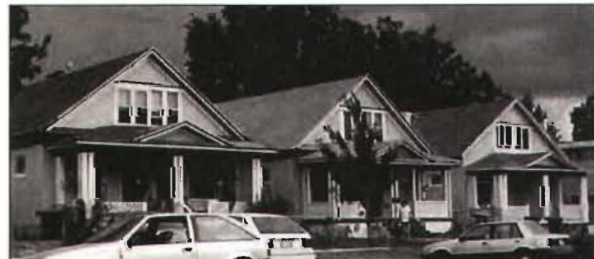
The uniform setback of these vernacular structures provides a sense of alignment and the porches provide a consistent orientation to the street.
