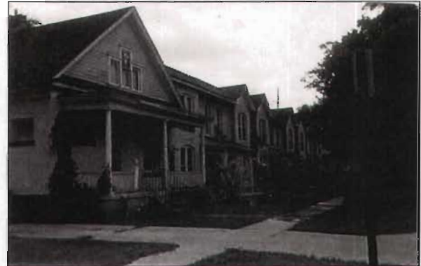
Use building materials that will appear similar to those used historically.
