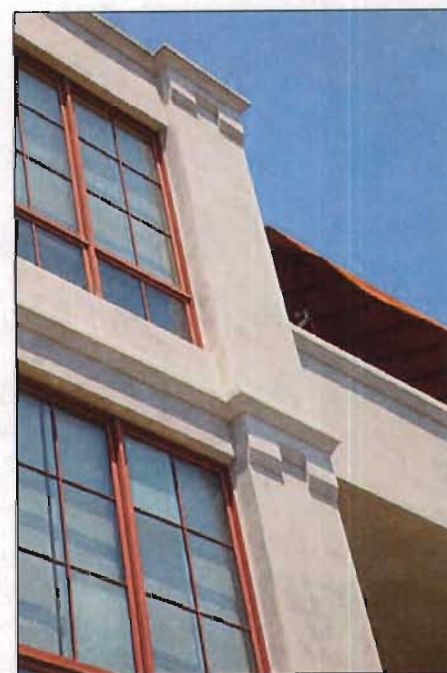
Window proportions, reveals and frame details can add visual strength and decorative embellishment to otherwise plain or sparsely modeled facades.
