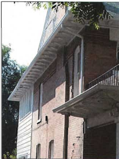
This rear addition respects the principal building by continuation of wall plane, eaves and bracket details, while changing the materials and fenestration.
