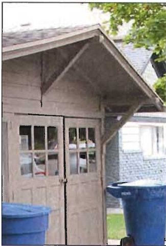
Street facing accessory structure reflecting the house design, and using a pair of side-hinged doors.
