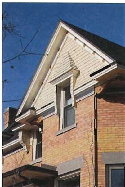
Original materials are essential to the integrity of a building and convey a sense of authenticity and maturity.
