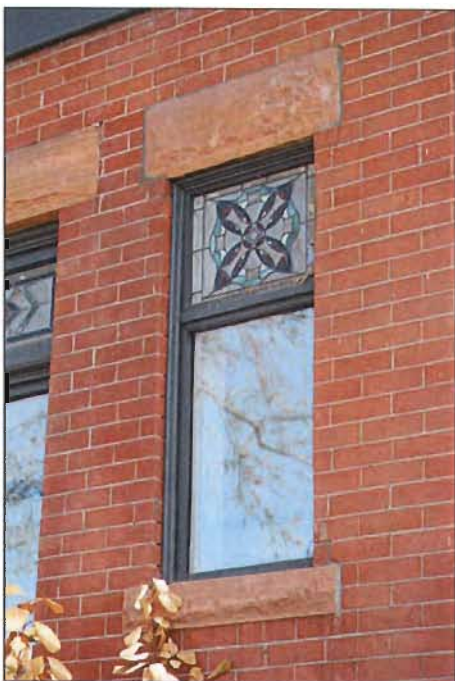
Matching the existing brick pattern or bond and the composition of the mortar mix help to ensure the integrity of the brick and stonework and consequently architectural character.
