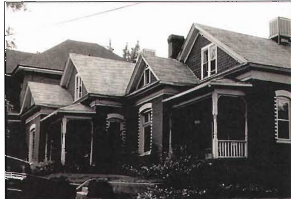
Staggered setbacks in the Marmalade district are due to its diagonal street pattern.
