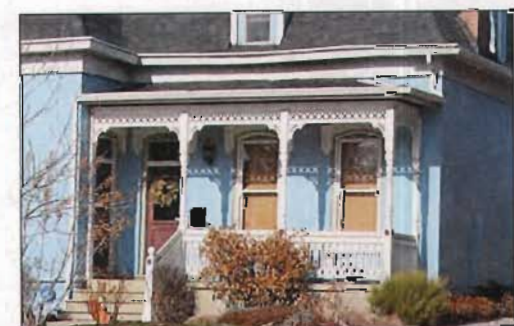
Wood detailing on porches such as this jigsaw ornamentation, or detailed balustrade, should be preserved.
