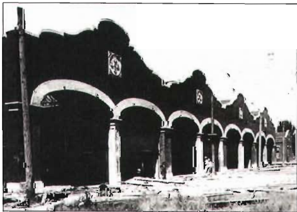
Trolley Square under construction.
