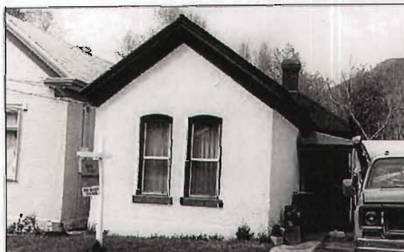
This is an unusual example of a front facing Greek Revival style building in the Capitol Hill Historic District. Despite the rarity of its orientation, its massing, stucco finish, pronounced wood cornices and fascia are clearly in keeping with this style and period.
