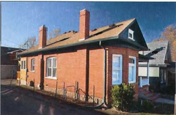
Small staggered rear addition continuing the axis and eavesline of the residence and distinguished by design and materials.
