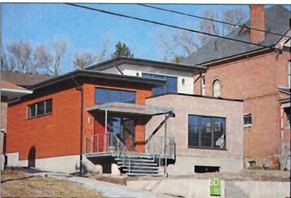
The massing of this building is designed to mediate between adjacent single and two story buildings, increasing in height incrementally as it steps back from the street frontage.
