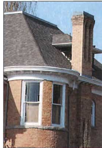
Asphalt shingles are the typical and appropriate roofing material for this style and period of architecture.
