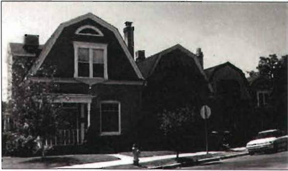
A row of Dutch Colonial structures angled with the street provides a distinct character to the streetscape of this block in the Capitol Hill district.
