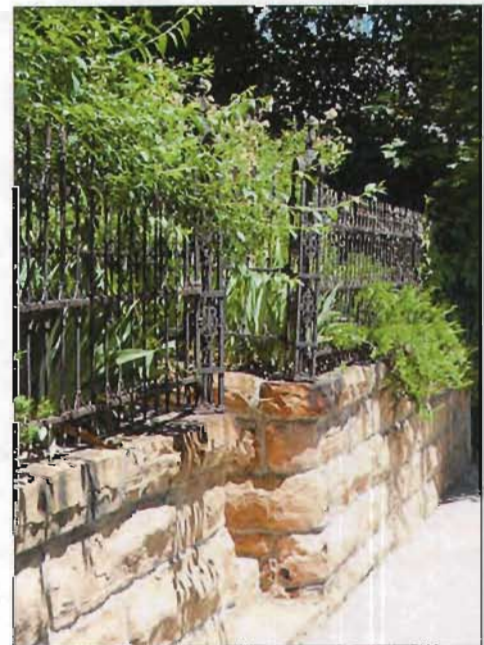
Historic wrought or cast iron fences provide visual richness to the street scene.
