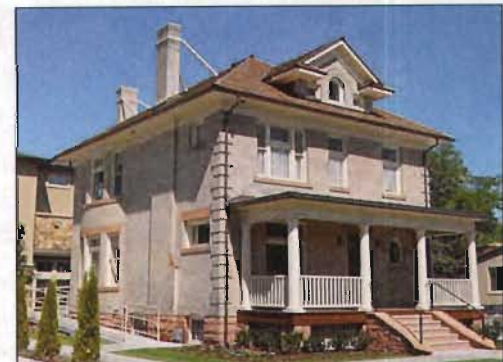
The Stanley F. Taylor building, a residence dating to c. 1906 was recently seismically upgraded as part of an extensive rehabilitation.
