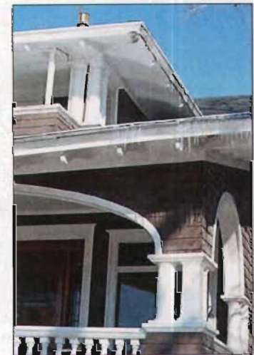
Features such as window hoods, brackets and columns are often associated with particular styles and therefore their preservation is important.
