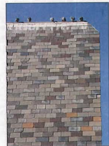
Cedar, clay and slate create special roof texture, color and character.
