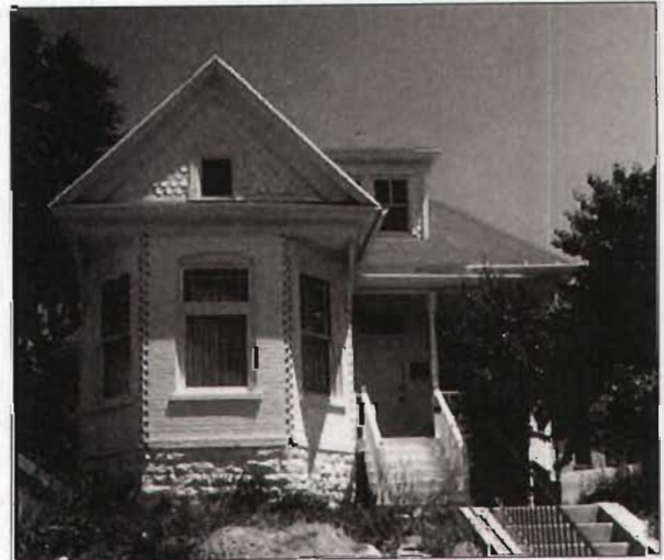
Decorative shingles in the gable, turned posts on the porch and the interlocking brick bay of this house exhibit the high degree of craftsmanship and attention to detail that mark many houses in the neighborhood.
