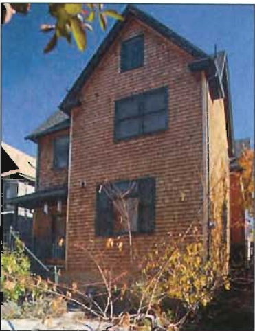
Front and rear views of substantial rear addition adopting original design cues.
