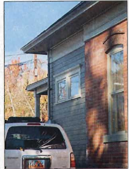
Rear addition reflecting form and scale and distinguished by wall plane, fenestration, detail and materials.
