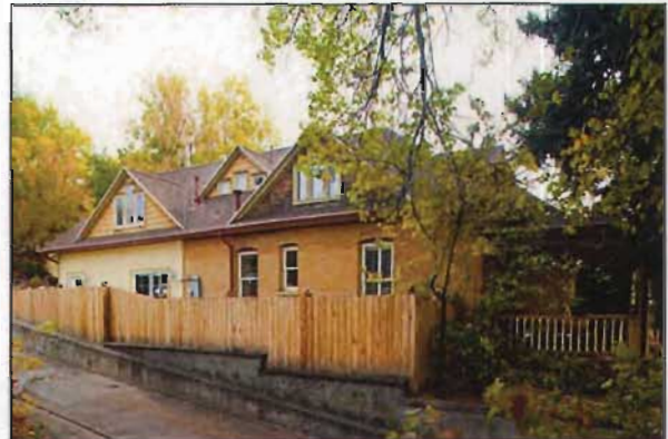
Addition to the rear of this house adopts the scale and design of the original and is clearly identified by a change in materials.
