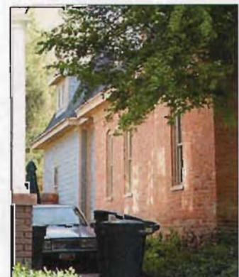
This recent addition reflects the design traditions of the original with a change in material to siding. The change from original to new is emphasized by a break in the wall plane and roof plane.
