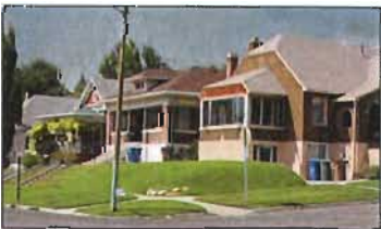
Enclosing a front porch will significantly compromise the architectural integrity of the house.
