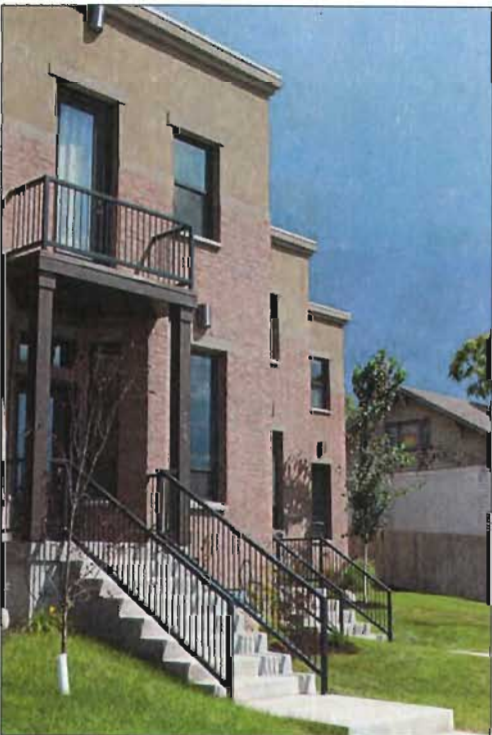
A strong vertical proportion and emphasis are created by the facade modules, tall entrance porchways and the pattern of doors and windows.
