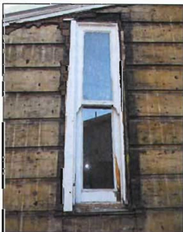
Removing later materials should reveal the original materials, which with care can be successfully repaired.
