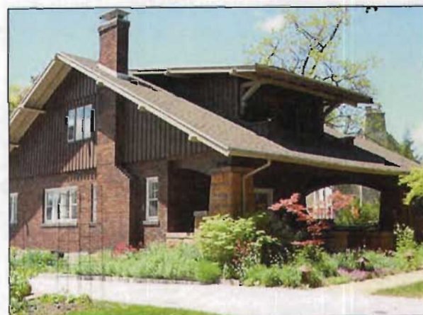
Bungalow porch with battered (tapered) columns.
