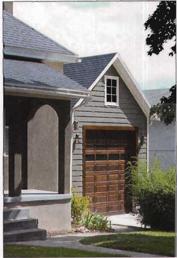
Recent street facing garage addition designed to respect scale & character.
