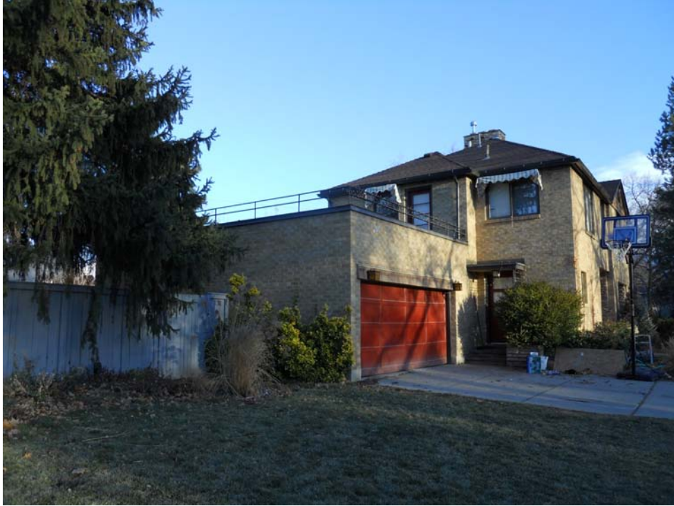
View of Existing Garage from West
