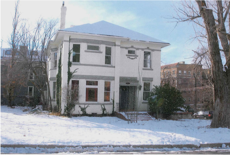
North Elevation Facing First Avenue
