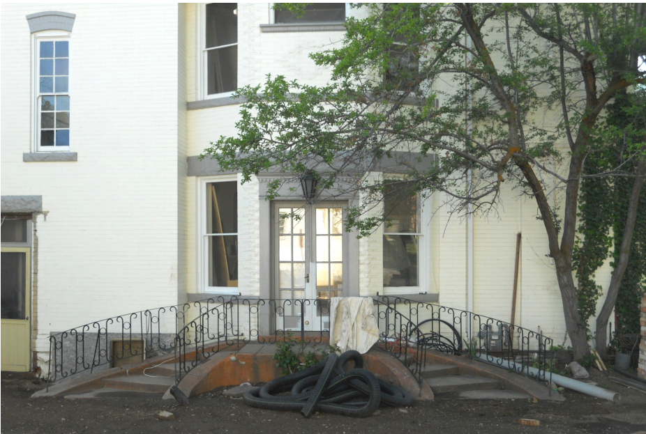
East Elevation Entryway to be partially removed
