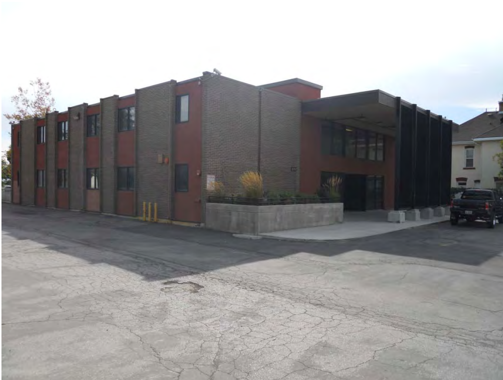
View of Property to the West (530 East 500 South)
