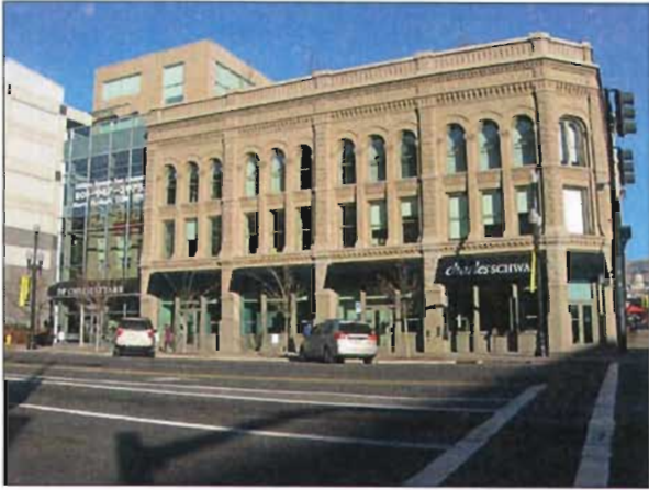
A change in material and a differentiation between historic and more current styles help define the change from old to new construction.
