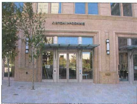
Canopies provide focus as well as shelter of the public, can be used to define an entry and add interest to a building's facade.
