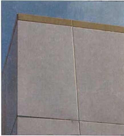
Porcelain panels on the Felt-Buchorn Building at 445 E. South Temple Street.
