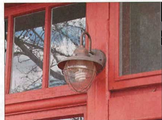
Good lighting choices for historic buildings are simple and unobtrusive, such as this example at 361 N. Main Street.
