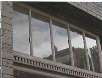
Original transoms contribute to the character of this historic storefront at 271 N. Center Street.
