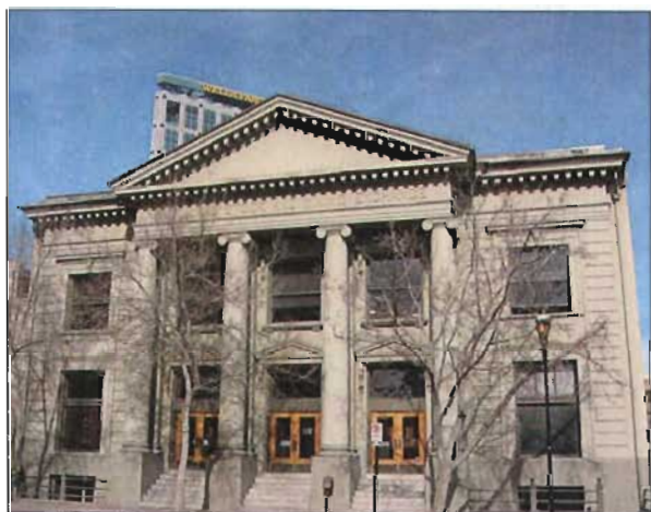
The Salt Lake Stock and Mining Exchange at 39 Exchange Place (1908) retains much of its original design. The building's form is central block with wings while its architectural style is Neoclassical. The projecting central bay displays Ionic columns and a large pediment with modillion blocks.
