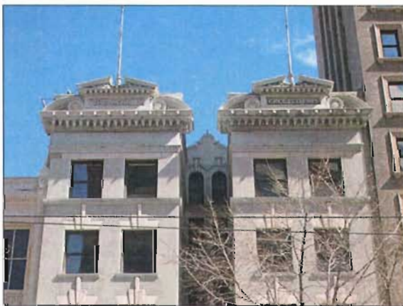
An ornate cornice crowns the Herald Building at 169 S. Main Street.
