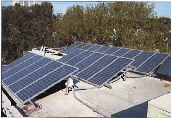
Rooftops may be an appropriate location for solar panels.
