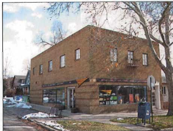
The building at 702 E 3rd Avenue (ca. 1940) was designed with simple detailing and has rectangular steel casement windows and original display windows.
