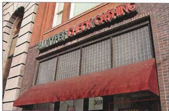
The distinctive Luxfer glass transom on the New Grand Hotel at 369-379 S. Main Street is intact and not concealed by the awning.
