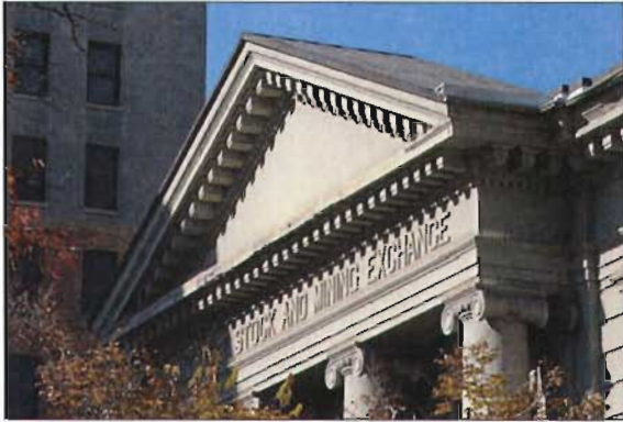
Classical detailing at 39 Exchange Place.
