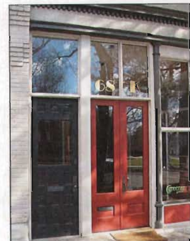
Salt Lake City's commercial buildings have a variety of doors and entrances.
