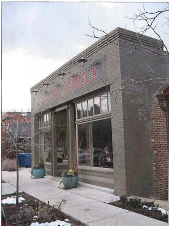
This one story building at 271 N. Center Street (c. 1900) is an example of a one-part commercial block.
