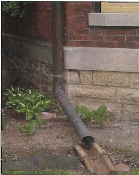
An appropriate downspout and splash block.
