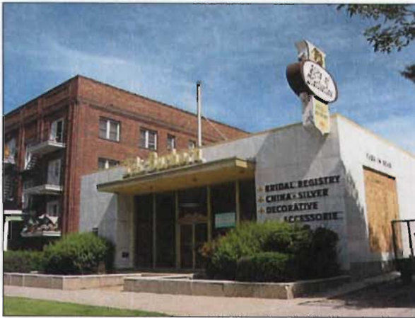
An enframed window wall plan is the Felt-Buchorn Building at 445 E. South Temple Street (1959). It displays a continuous surround of porcelain steel panels which frame the display windows and entrance.
