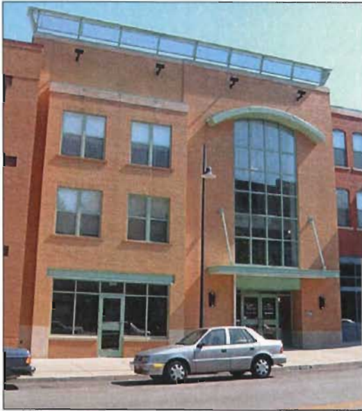
Articulation in facade elements can reduce the apparent mass and scale of a building.
