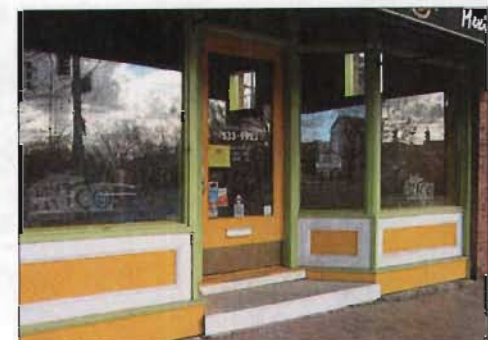
Bulkheads act as a platform for display windows.
