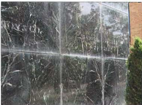
Marble paneled veneer on the main facade at 641-645 E. South Temple Street.
