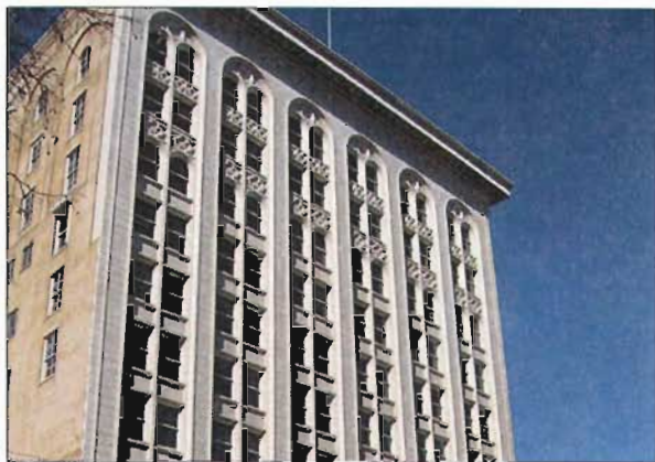
The Kearns Building at 136 S. Main Street is representative of the Sullivan-esque style.
