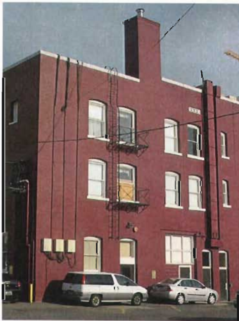
This chimney is incorporated into the building facade.
