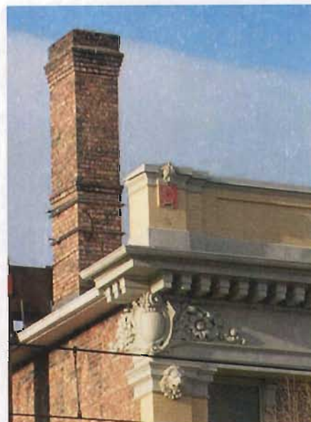
Chimneys can be an integral part of the roof composition.
