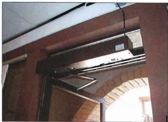
Doors can be modified with pressurized door openers to allow for ease of access.
