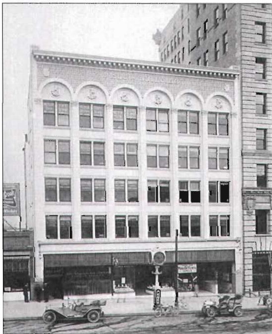
The Felt Building (1910) at 339 S. Main Street displays early use of terra-cotta as a decorative element. (Courtesy Utah State Historical Society)
