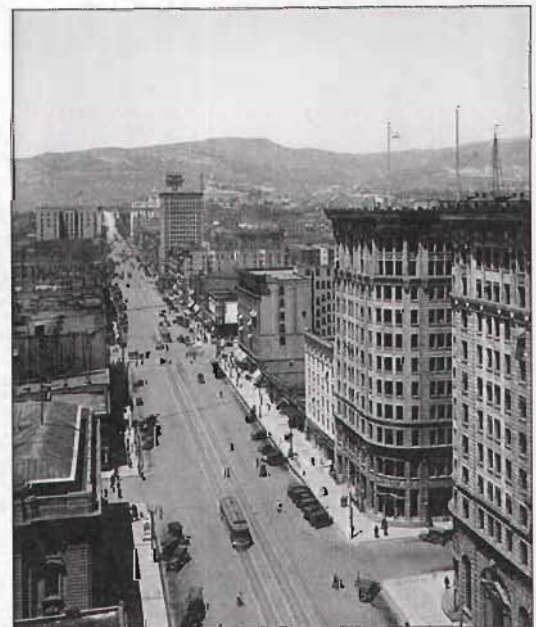
Skyscrapers, like the 11-story Boston Building (1909), at Exchange Place and Main Street, became more common with the development of a lucrative mining economy.
