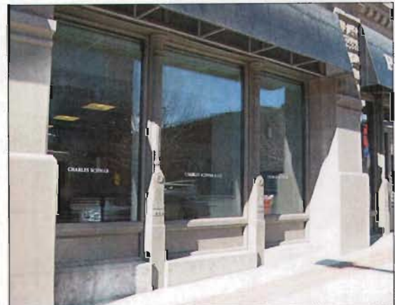
Cast iron columns embellish the window frame on the Brooks Arcade at 268 S. State Street.
