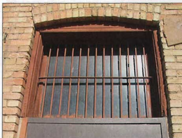
Security bars are more appropriate on side or rear facades.
