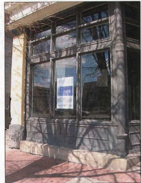
An original tile bulkhead at 422-426 North 300 West.
