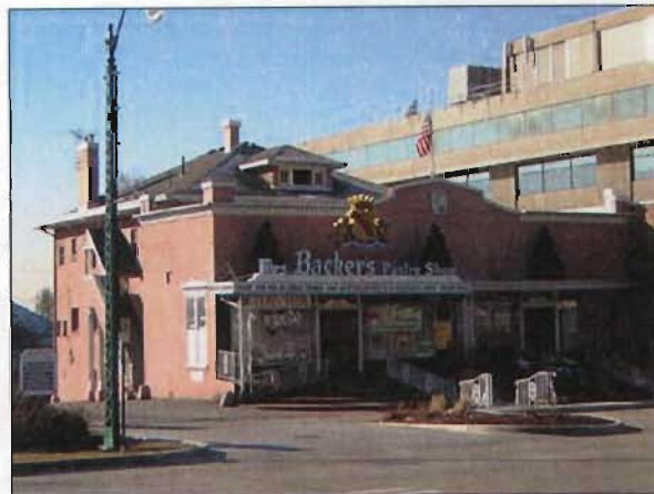
The storefront was an early addition to the building at 434 E South Temple Street.
