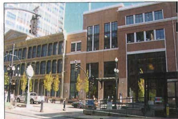
A step back provides a transition between the historic ZCMI storefront and the infill construction.
