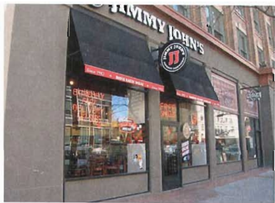
Awnings are generally simple in design, angled and fit within the window opening.
