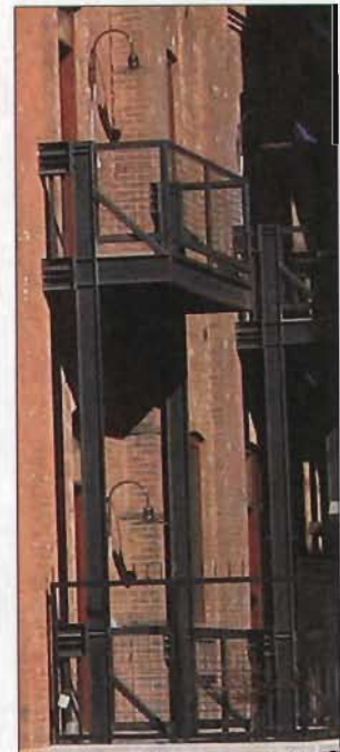
This metal fire escape has been appropriately added to the side facade of the building.
