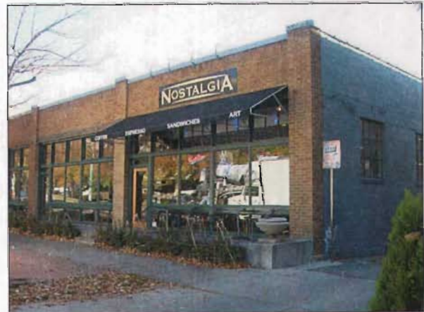
Most historic commercial buildings were designed with flat or gently sloping roofs.
