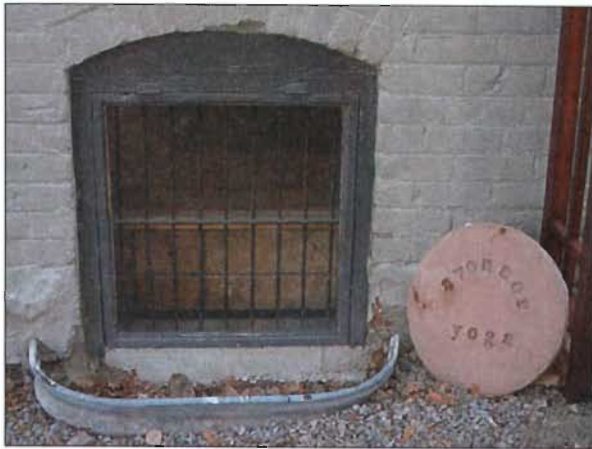
Installing security bars on the inside of windows is a solution that accommodates both design and security considerations.
