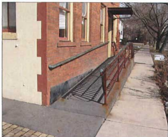
This accessibility ramp is successfully integrated with the historic building both in scale and materials.
