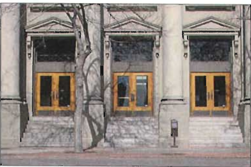
These three center bays are framed by four freestanding Ionic columns. Salt Lake Stock and Mining Exchange, 39 Exchange Place.
