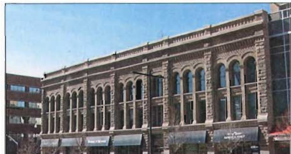
Rounded arches and textured masonry are common features of the Richardsonian Romanesque style.
