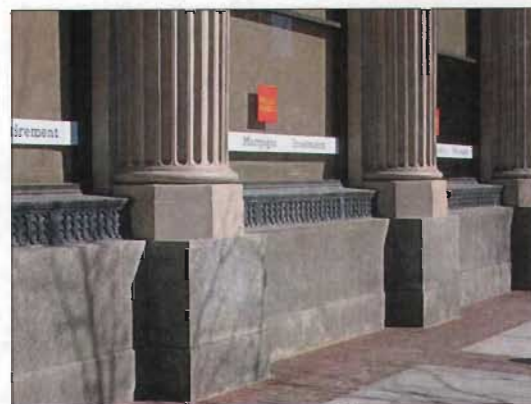
Foundation walls with high quality materials and intricate detailing are important in establishing the architectural character of a historic building.
