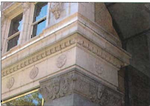
Molded terra-cotta rosettes adorn the facade of the Kearns Building at 136 S. Main Street.
