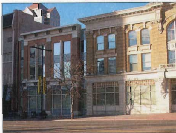
The design of the addition reflects the historic alignments and rhythms that exist on the primary facade of the historic building.
