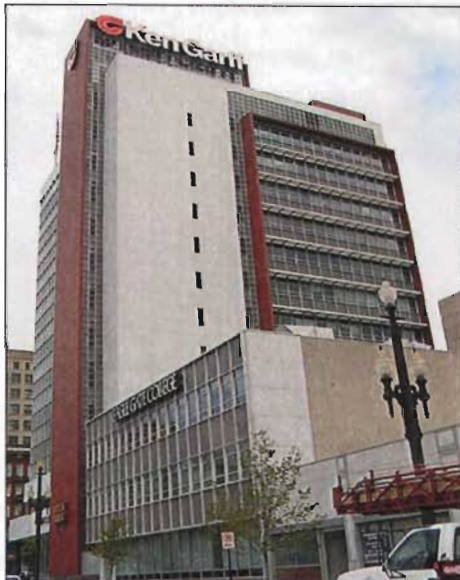
The First Security Bank Building at 405 S. Main Street (1955) features an exterior curtain wall of glass, aluminum, and enameled porcelain panels.
