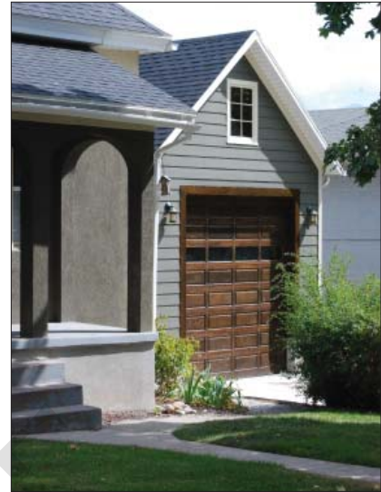
Recent street facing garage addition designed to respect scale & character.
