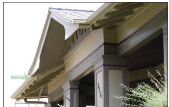
Eave profiles & rafter tails are key parts of the design.
