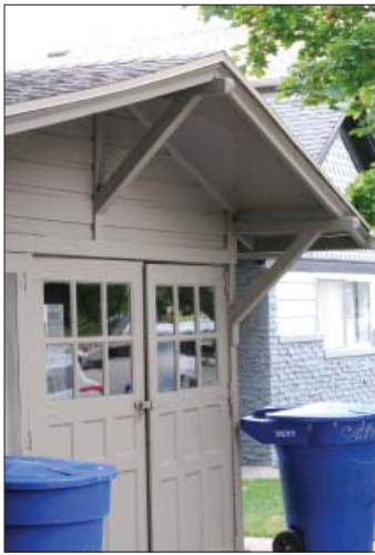
Street facing accessory structure reflecting the house design.
