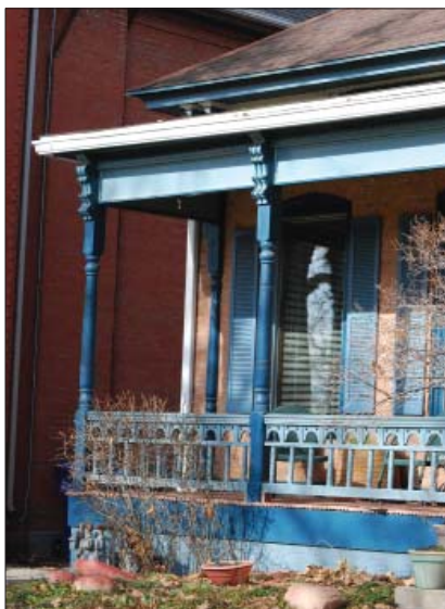
Intricate porch detailing is reflected elsewhere on the building.
