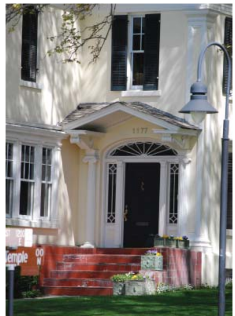
The doorway, the proportions of opening and framework, sidelights and transom/fan lights, finer intricate details, and the design of the door itself, combine to celebrate the entrance.
