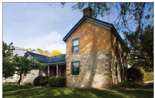
Second story addition to a historic plan form, closely reflecting the original design and identified by a change in materials
