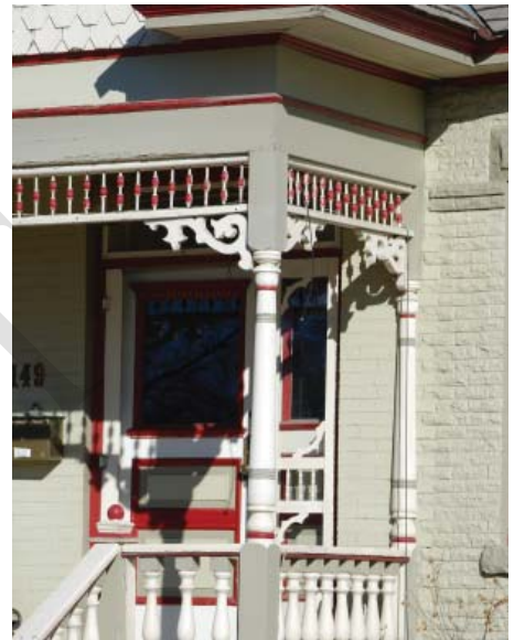
Ornamental trim on historic doors contribute significantly to the character of the building frontage and porchway
