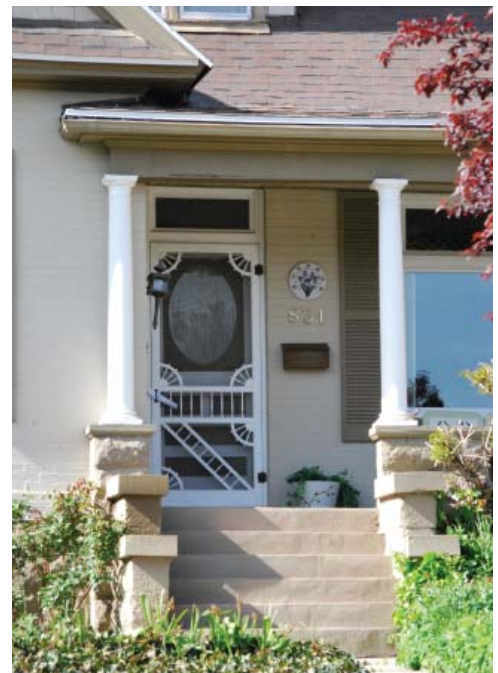
In this case the storm door and screen provide a decorative addition to the original design and detail of the door.
