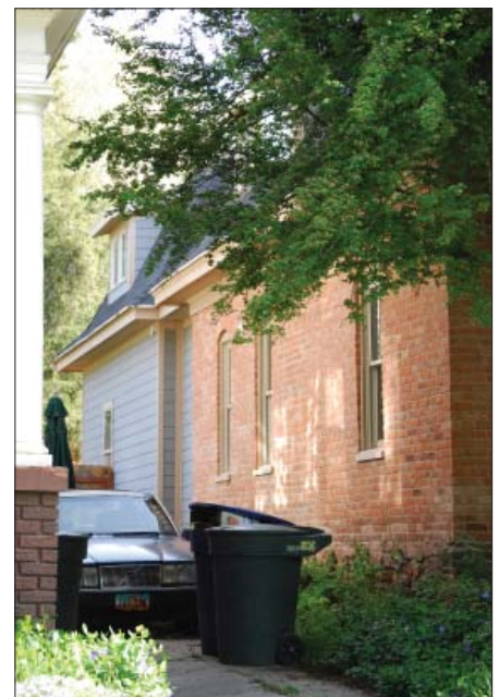
This recent addition reflects the design traditions of the original with a change in material to siding. The change from original to new is emphasized by a break in the wall plane and roof pitch.
