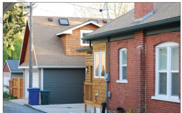
Small rear addition of contrasting style continuing the eavesline, with additional separate garage with accommodation above
