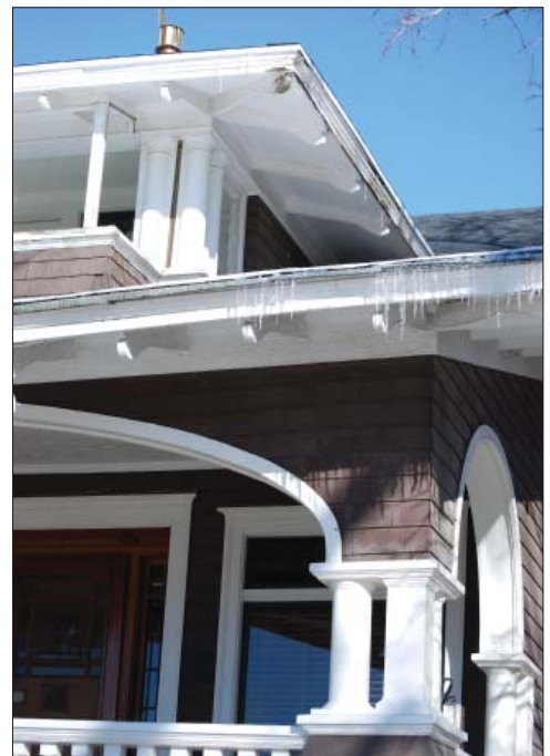
Features such as window hoods, brackets and columns are often associated with particular styles and therefore their preservation is important.
