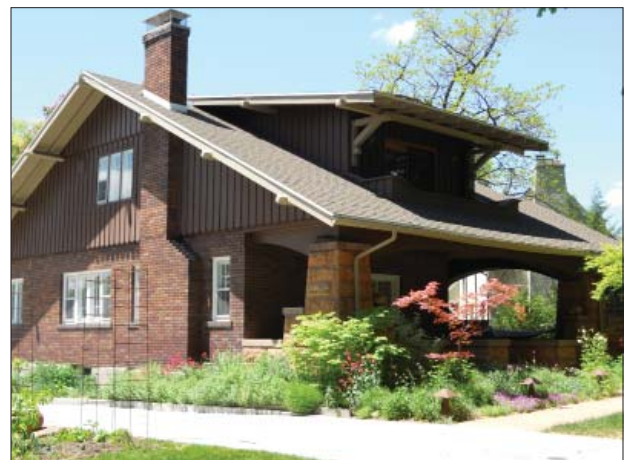
Bungalow porch with battered (tapered) columns.
