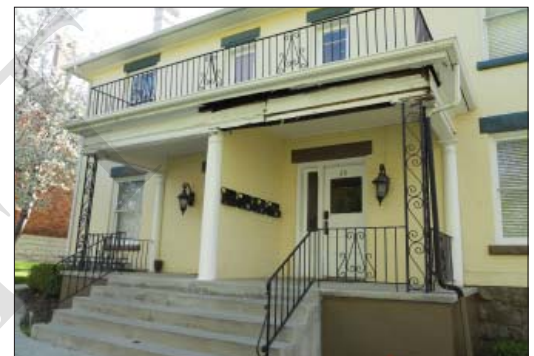
Repair original elements of the porch and consider reinstating original features which have been lost.
