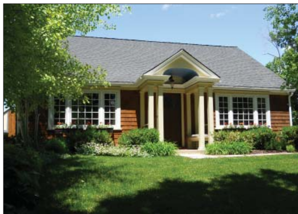
Asphalt shingles are the typical and appropriate roofing material.
