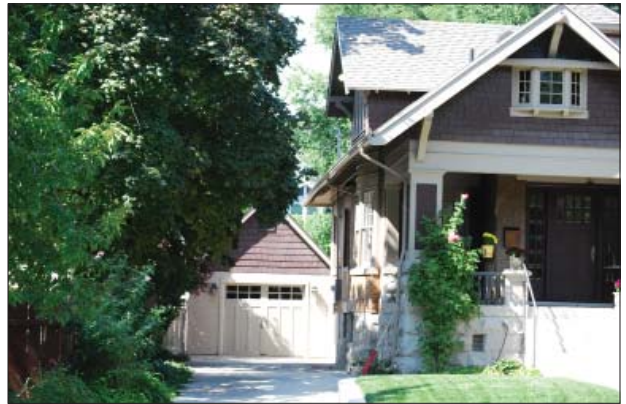
This garage reflects the design of the house in form, details and materials.
