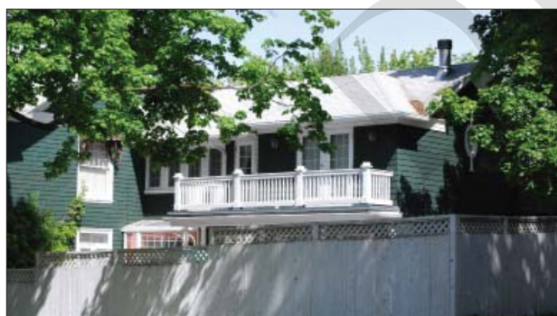
New roof forms can compliment the original.
