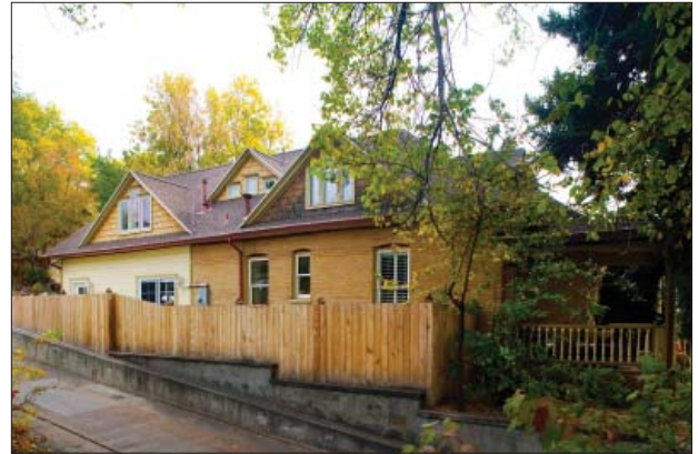
Addition to the rear of this house adopts the scale and design of the original and is clearly identified by a change in materials
