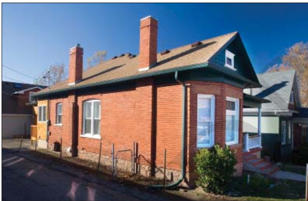
Small staggered rear addition continuing the axis and eavesline of the residence and distinguished in design and materials
