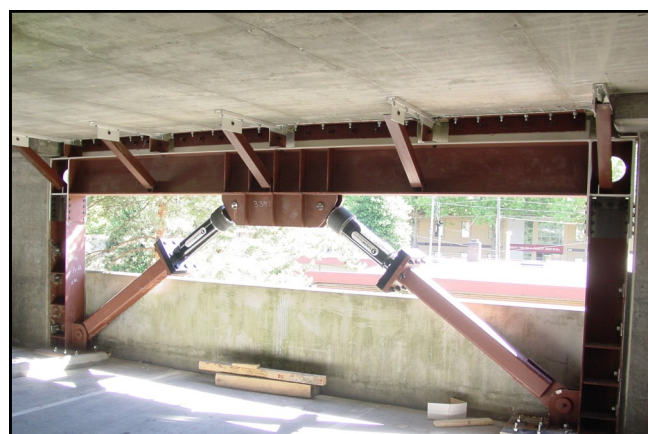
Seismic retrofitting can include adding steel frames and dampers in basement and parking areas of commercial buildings.
