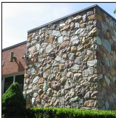
This stone veneer corner bay is at 633 E South Temple Street and built in 1960.
