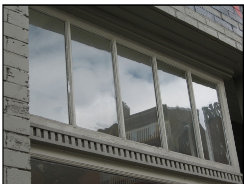
Original transoms enhance historic character and are important elements of storefronts.
