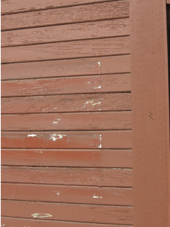
Preserve and maintain original wood siding
