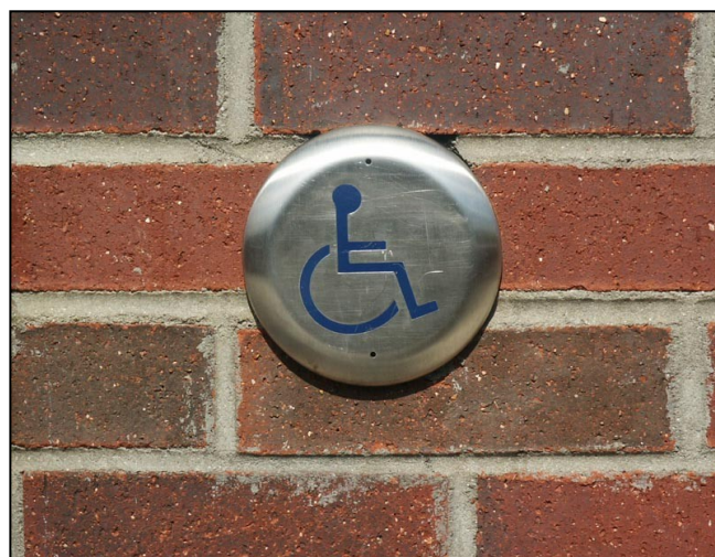
Push plates for ADA access are appropriate solutions for access into commercial buildings.
