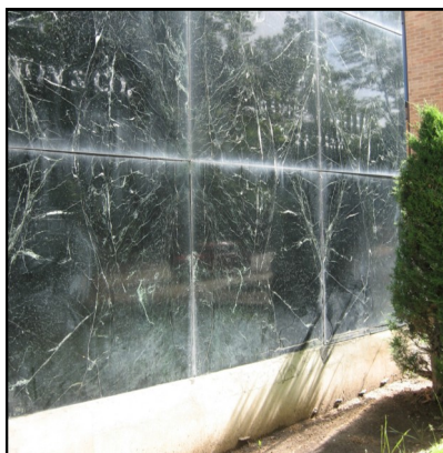
Marble paneled veneer on the main façade at 641-645 E South Temple Street, which was built in 1957.
