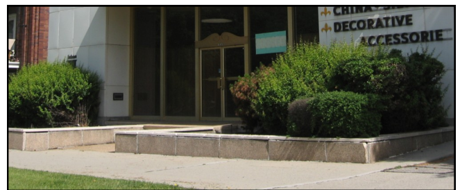
Retaining walls in front of commercial buildings such as this example at 445 E South Temple Street provide interest to the streetscape.
