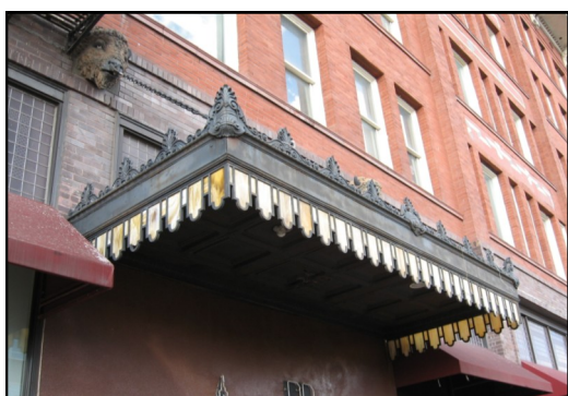
An example of a metal awning on the New Grand Hotel at 369-379 S Main Street.
