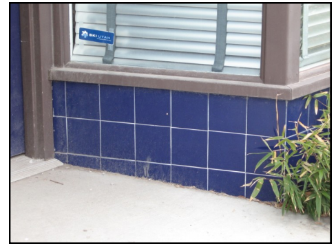
An original tile bulkhead at 422-426 N
