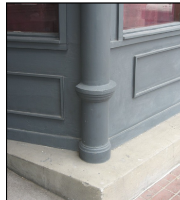
Preserve and maintain original cast iron features such as those at 68 N 'K' Street (above) and (below).
