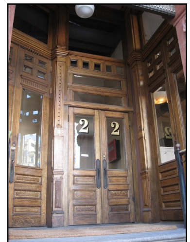
Wood doors on Utah Commercial & Savings Bank Building at 22 E 100 South.
