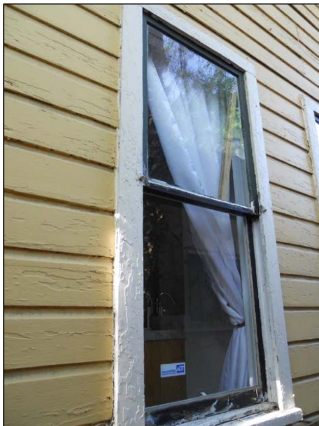
Subject Window #5 (Westernmost Window)
