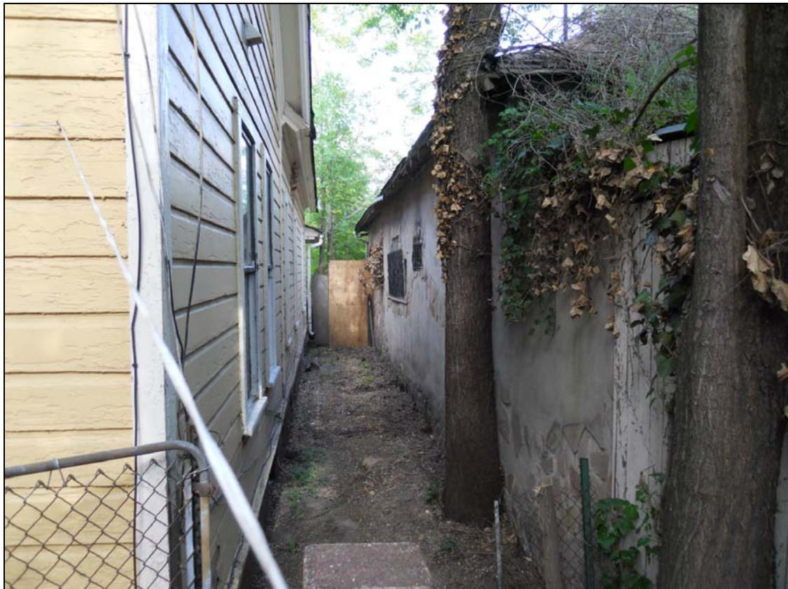
View of Subject Windows from Rear
