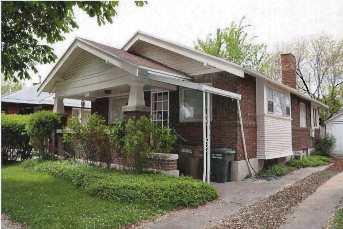
Photograph 5. 147 E. Harvard Ave., facing northwest.
