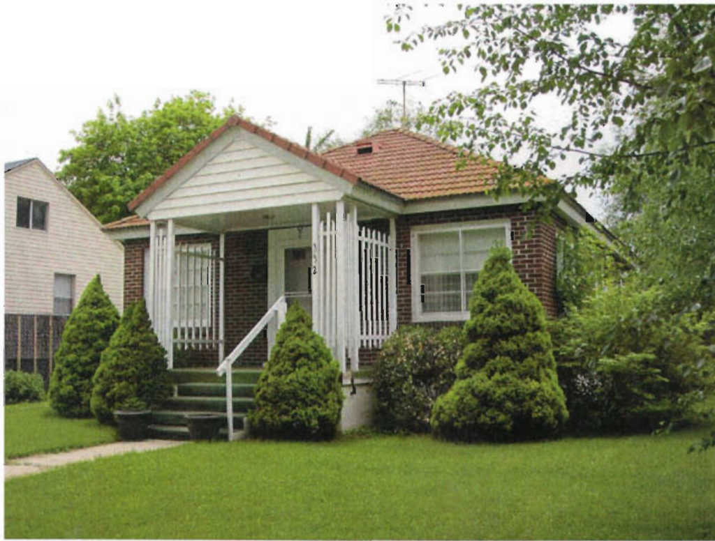
Photograph 20. 332 E. Williams Ave., facing south-southeast.
