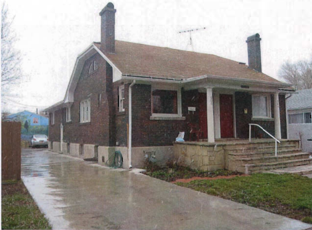
Photograph 11. 964 S. Denver St., facing southwest.
