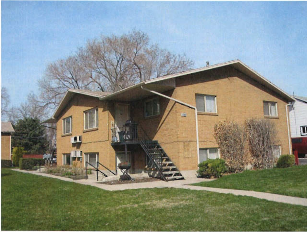
Photograph 22. 1140 S. 500 E., facing west-northwest.
