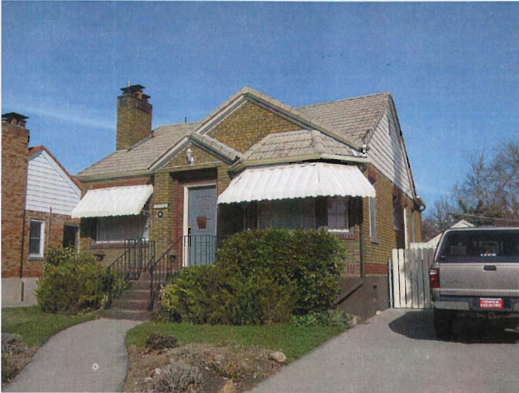
Photograph 13. 1123 S. 400 East, facing northeast.
