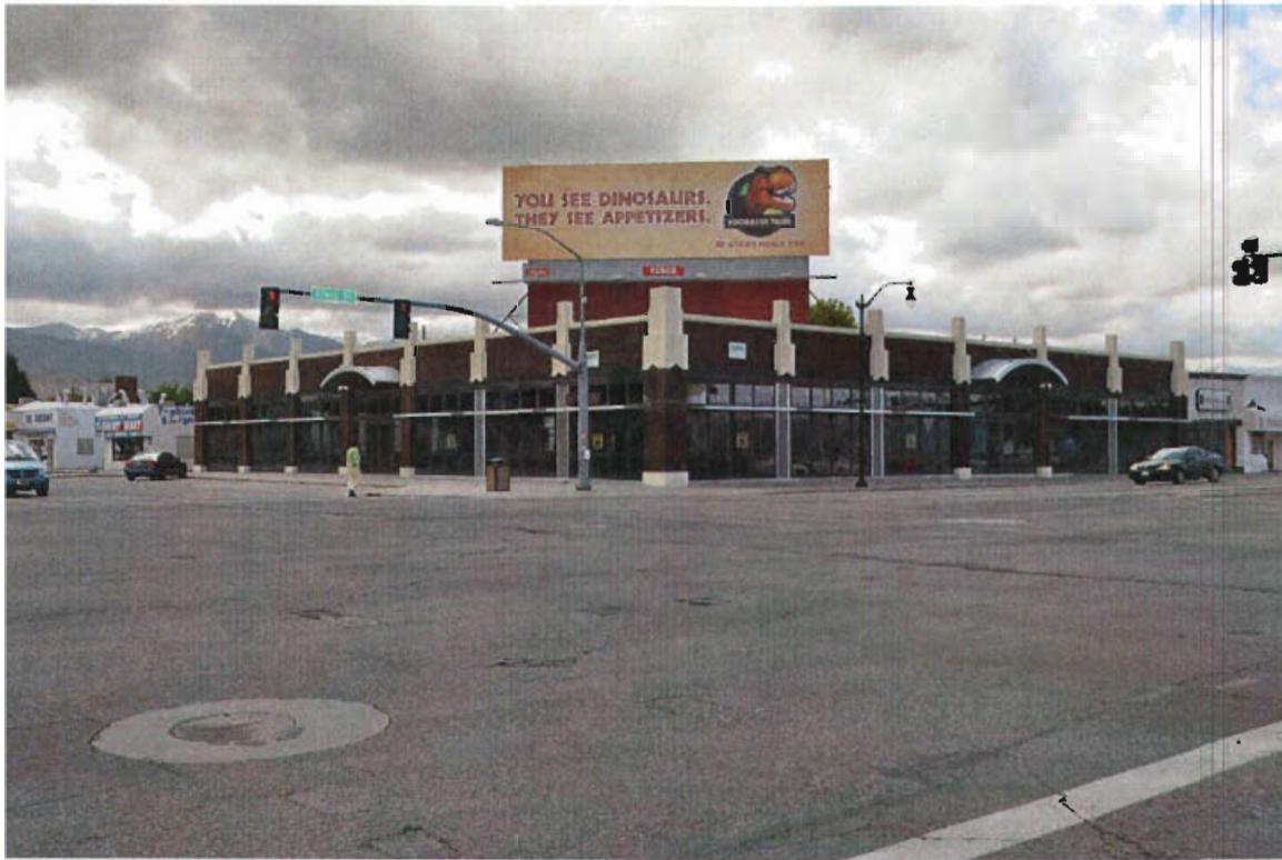
Photograph 18. 905 S. State St., facing southeast.
