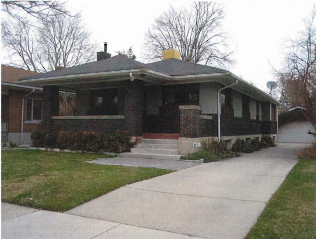
Photograph 6. 457 E. Edith Ave., facing northeast.
