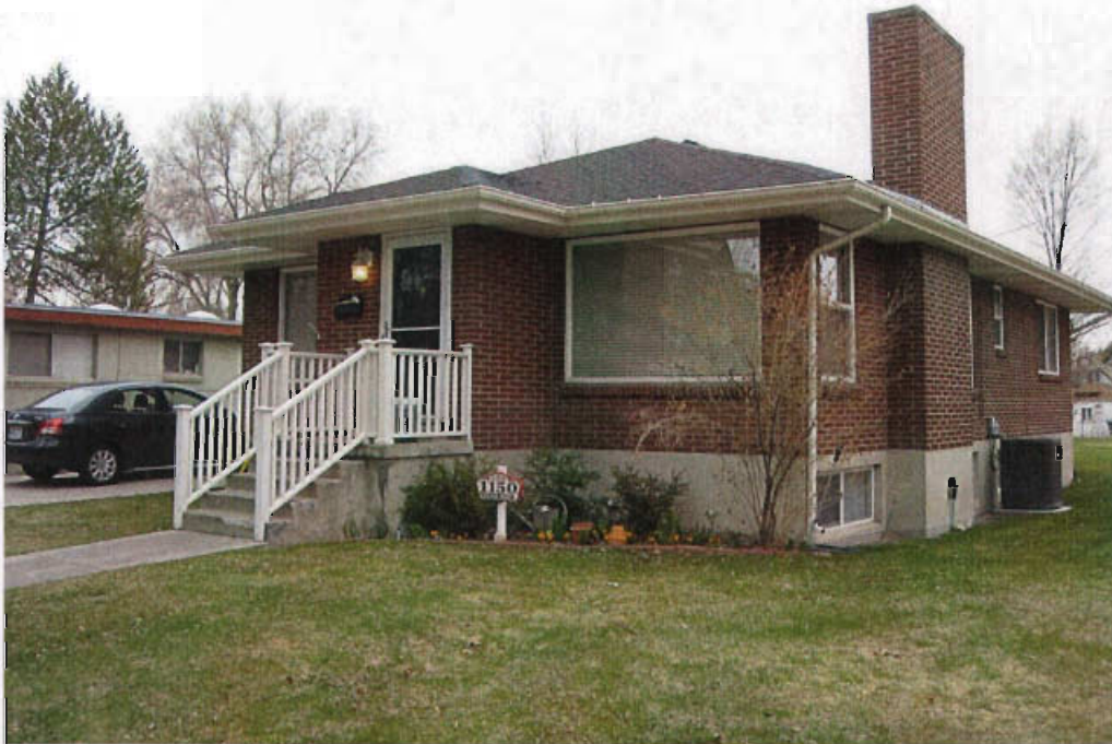
Photograph 21. 1150 S. Denver St., facing southwest.
