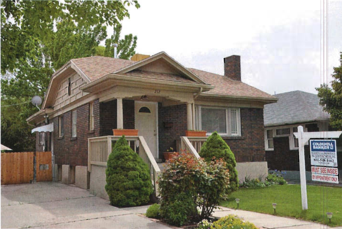
Photograph 8. 252 E. Belmont Ave., facing southwest.
