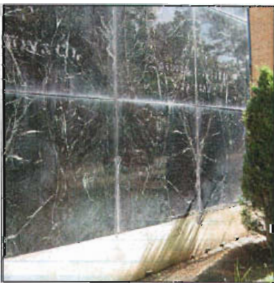
Marble paneled veneer on the main façade at 641-645 E South Temple Street, which was built in 1957.
