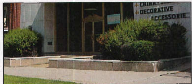
Retaining walls in front of commercial buildings such as this example at 445 E South Temple Street provide interest to the streetscape.
