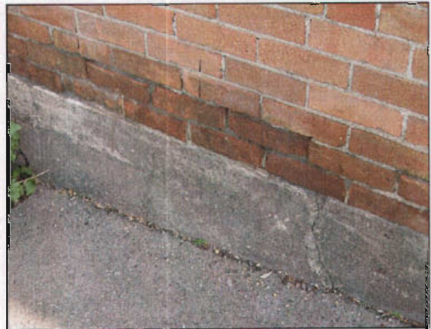
A concrete foundation at 422-426 N 300 West.
