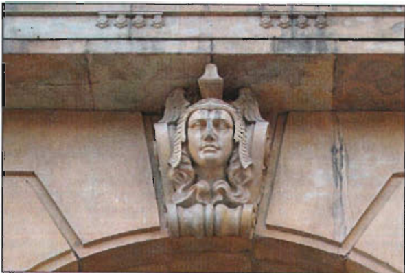
Preserve and maintain details such as this decorative keystone at 32 Exchange Place.
