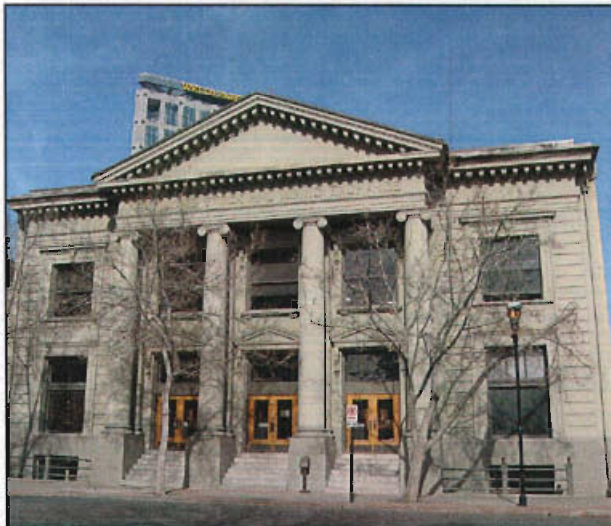
The Salt Lake Stock and Mining Exchange at 39 Exchange Place demonstrate the Neoclassical style with prominent classical columns and accentuated entrances.
