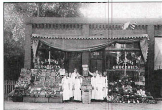
In addition to downtown, neighborhood commercial buildings were constructed in the early 20th century such as F. J. Lucas Grocery at 267-269 W 200 South, shown in 1909. (Courtesy Utah State Historical Society)
