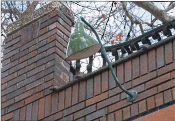
Swan- or goose-neck fixtures in dark metals are appropriate new light fixtures for commercial buildings, as at 82 N 'Q' Street (left) and 422-426 N 300 West (right).
