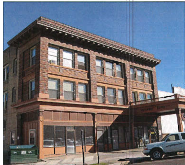
Pilasters divide the upper façade at 222 W 300 South and present a balanced and symmetrical appearance.
