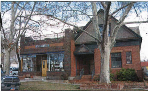
This building at 82 N 'Q' Street (1898) features an original storefront in the commercial section.
