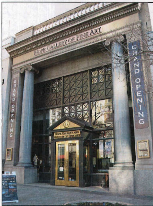
The Tracy Loan Trust Company (1916) was constructed at 151 S Main Street. This vault design features a large central bay with a pedimented entrance flanked by Ionic columns. In addition to the entrance, the central bay is composed of a large window wall.
