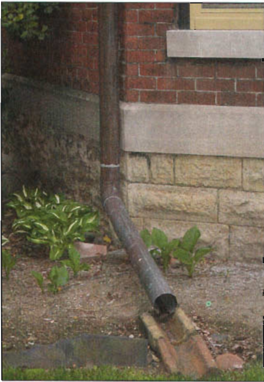
Appropriate downspout and splash block.
