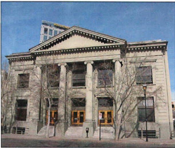
The Salt Lake Stock and Mining Exchange at 39 Exchange Place (1908) retains much of its original design. The building's form is central block with wings while its architectural style is Neo-classical. The projecting central bay displays Ionic columns and a large pediment with modillion blocks.
