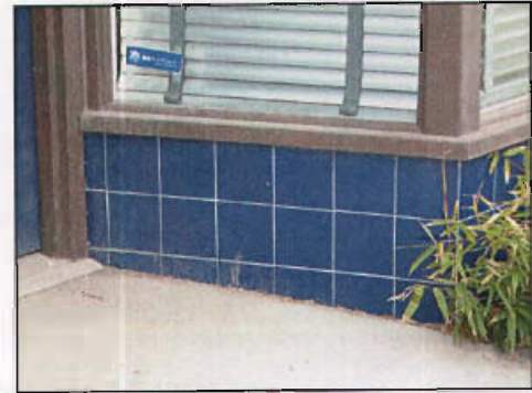
An original tile bulkhead at 422-426 N
