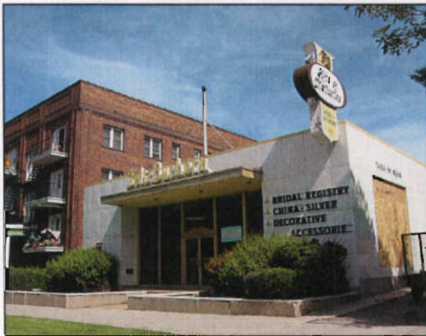
An enframed window wall plan is the Felt-Buchorn Building at 445 E South Temple Street (1959). It displays a continuous surround of porcelain steel panels which frame the display windows and entrance.
