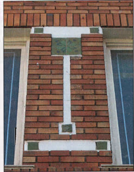
Architectural details at 145 S State Street.
