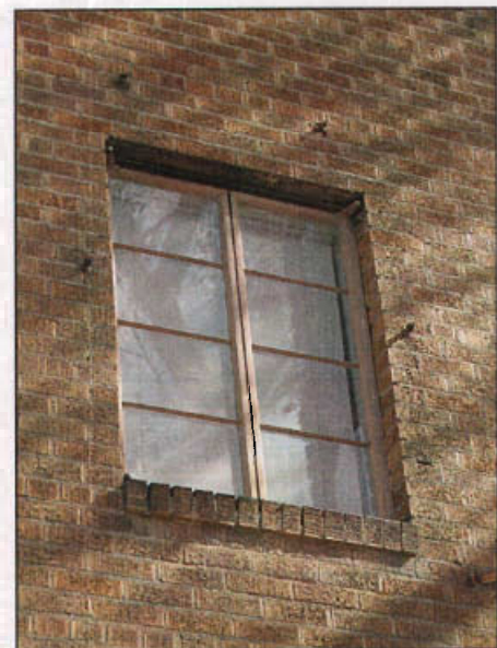
Traditional steel casement frames are durable as well as characteristic.
