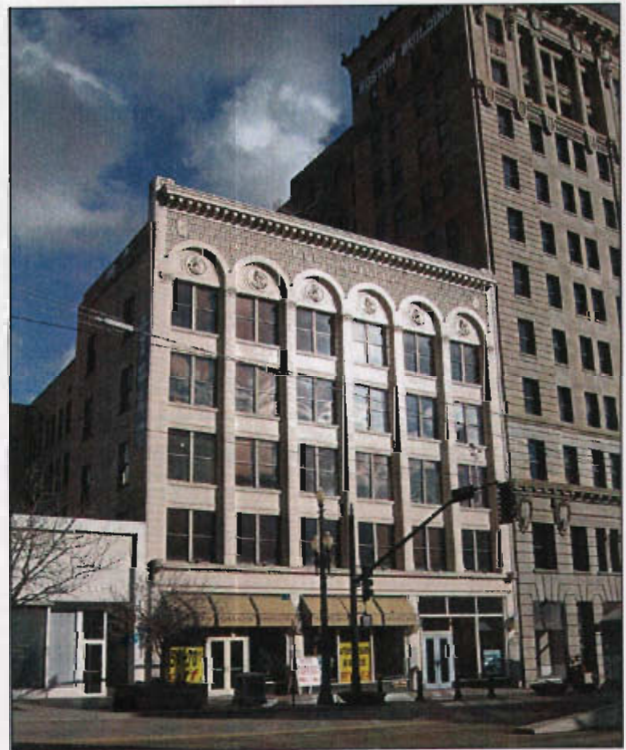
The Felt Building at 335-339 S Main Street (1909) has a separate storefront zone and unified upper façade. The building is distinguished by its glazed terra-cotta and arched panels below the cornice.
