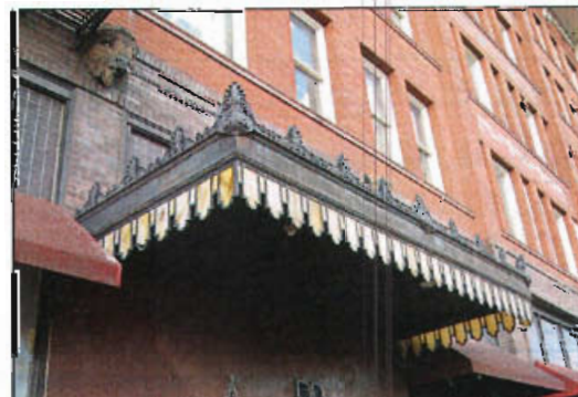
An example of a metal awning on the New Grand Hotel at 369-379 S Main Street.
