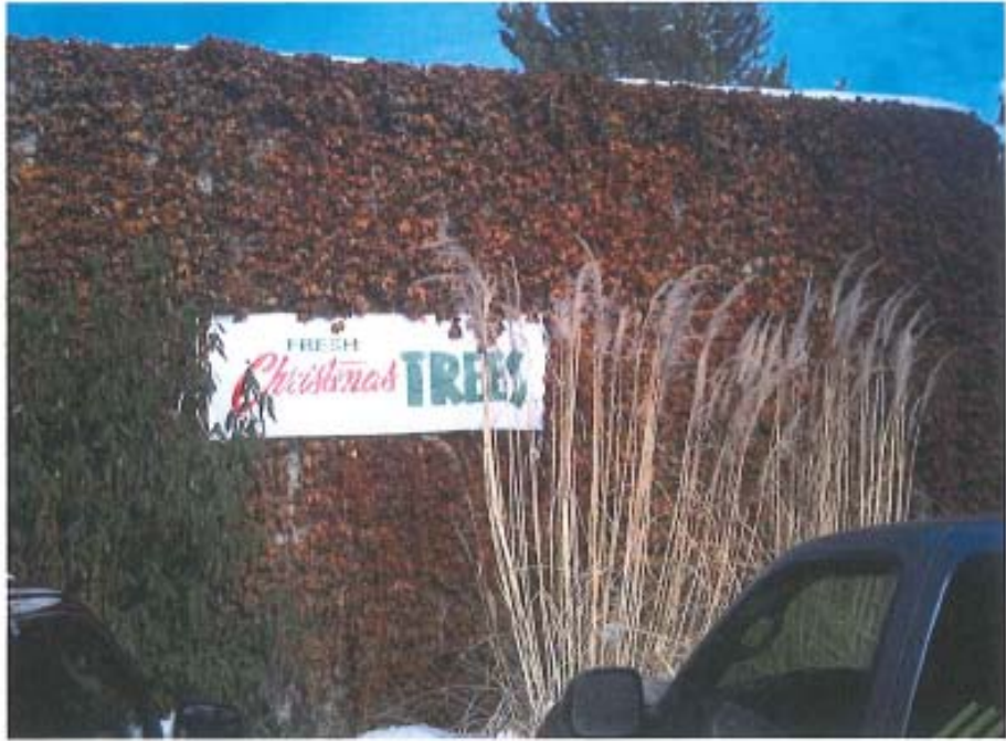
South Elevation Designated as "Reception Center"
