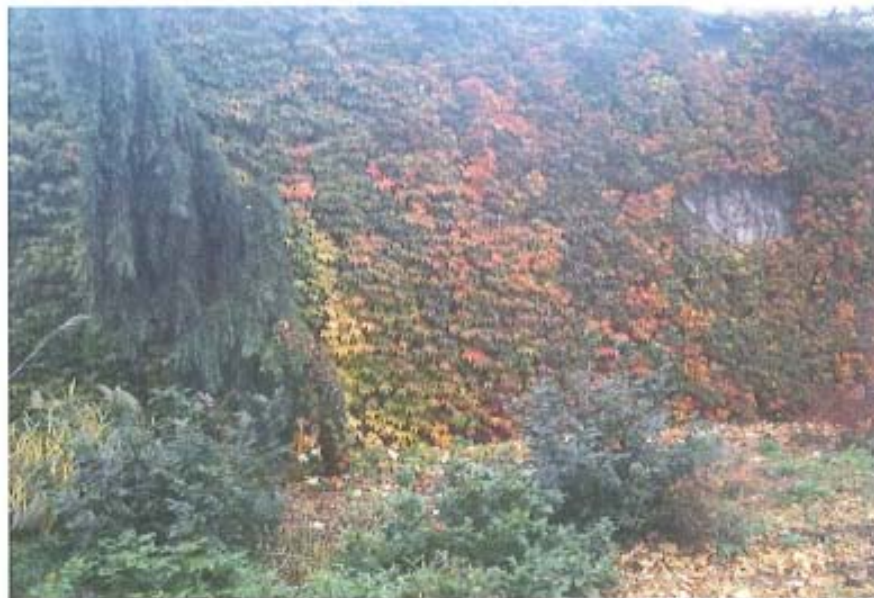
East Elevation Designated as Reception Center
