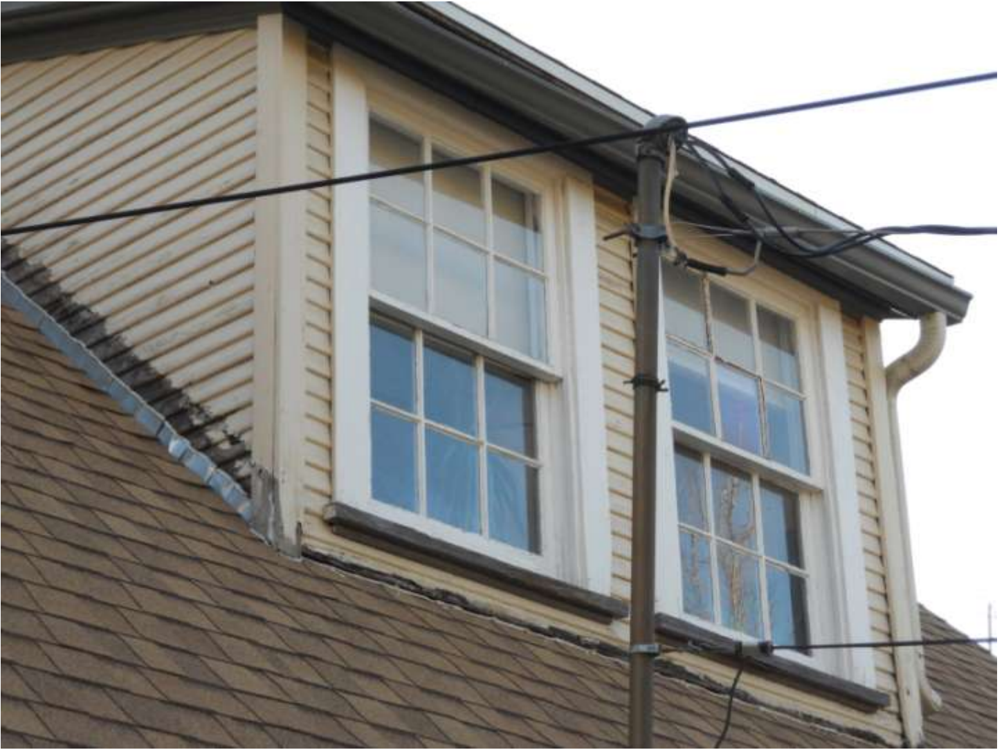
Rear Façade: Dormer Windows to be Replaced
