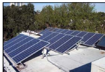
Rooftops are the preferred location for solar panels.
