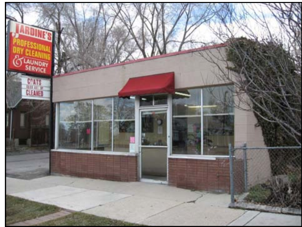
Neighborhood shopping center commercial buildings continued to be constructed into the 1940s in many residential areas of the City (442 N 300 West).
