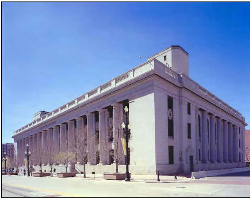
The Federal Building and Post Office at 350 S Main Street was completed in 1906 and is an example of an enframed block designed in the Neo-classical style. The building is distinguished by its long row of engaged Doric columns on each elevation.
