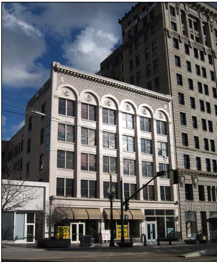
The Felt Building at 335-339 S Main Street was constructed in 1909 and has a separate storefront zone and unified upper façade. The building is distinguished by its glazed terra cotta and arched panels below the cornice.
