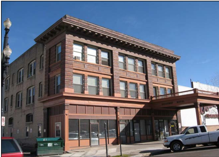
Pilasters divide the upper façade at 222 W 300 South and present a balanced and symmetrical appearance.
