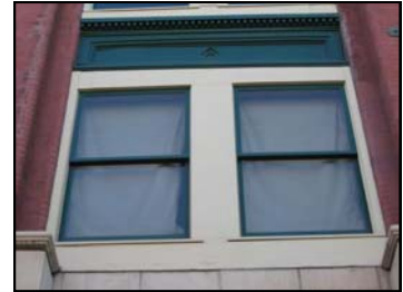
These one-over-one sash windows are a good example of replacement windows. They match the historical design and configuration of the original windows.
