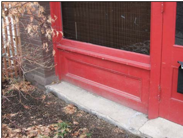
Original wood bulkheads such as those at 361 N Main Street (left) and 779 S 500 East (right) are significant parts of historic storefronts.
