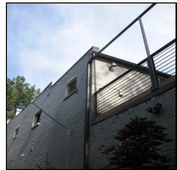
Decks such as this second floor addition at 68 N 'K' Street are appropriate as long as they are not readily visible from the street and are located at rear elevations.
