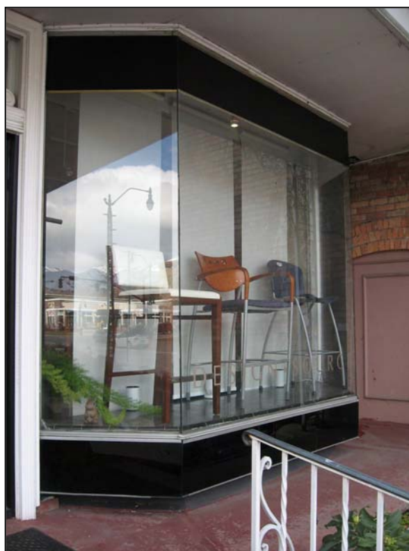
Few historic commercial buildings are located along South Temple but at 432-434 E South Temple Street is a building with an intact ca. 1930s Carrara glass storefront.
