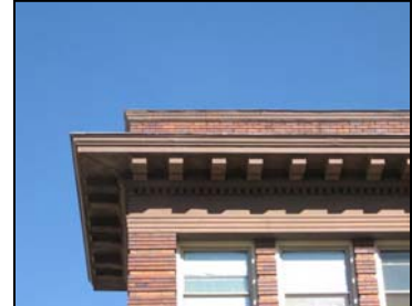
Preserve and maintain historic cornices (Broadway Hotel, 222 W 300 South).
