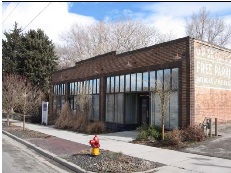
The building at 422-426 N 300 West is a one-story example of an enframed window wall plan with a simple brick surround around the storefront.
