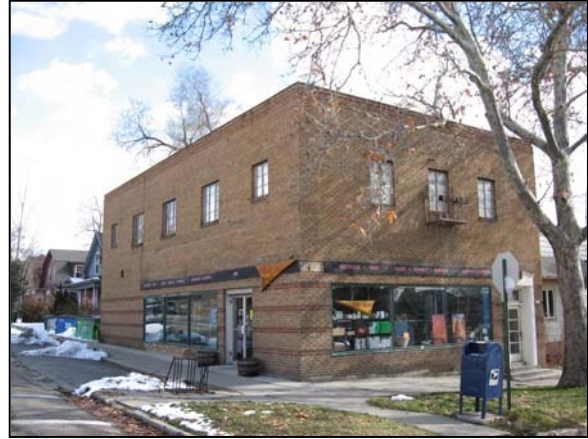
This building was designed with simple detailing ca. 1930 and has rectangular steel casement windows and original display windows (702 E 3rd Avenue).
