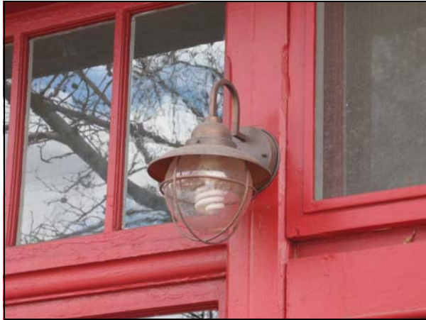
Good lighting choices for historic buildings are simple and unobtrusive, such as the example shown above at 361 N Main Street.
