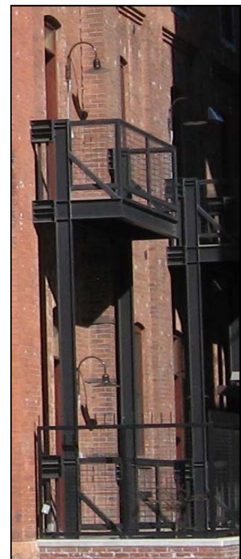
This metal fire escape has been appropriately added to the side elevation.
