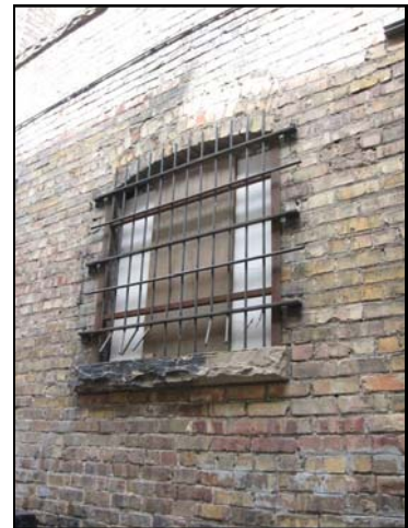
Security bars are more appropriate on side or rear elevations.
