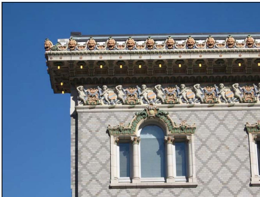
Architectural details of the Capitol Theatre include an ornate cornice and decorative window hoods and surrounds.
