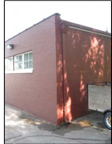
Appropriate rear gutter and downspout at 784 N 300 West.
