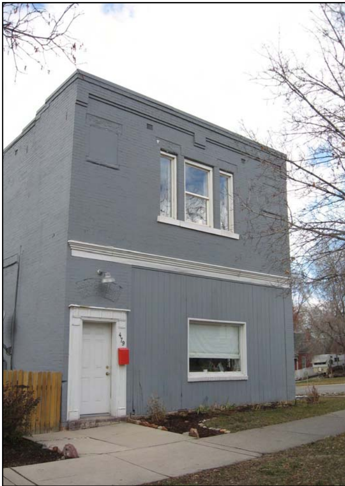
A number of neighborhood commercial buildings were converted into residences in late 20th century. This building at 479 N 200 West lost its original storefront and entrance when it was redesigned for residential use.
