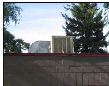
This roof mechanical system is set back so that it is not readily visible from the street.
