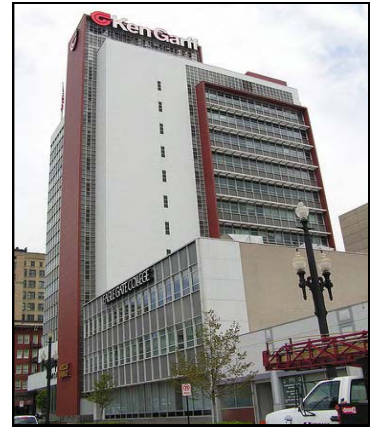
The First Security Bank Building at 405 S Main Street was the City's first modern skyscraper.
