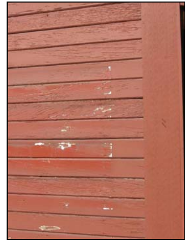
Original wood siding, 271 N Center Street.
