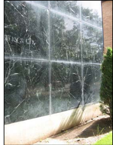
Marble paneled veneer on the main façade at 641-645 E South Temple Street, which was built in 1957.
