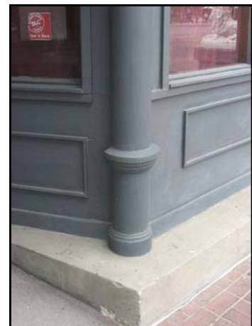
Preserve and maintain original cast iron features such as those at 68 N 'K' Street (above) and (below).
