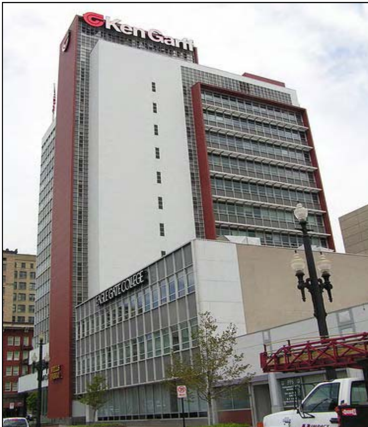
The First Security Bank Building at 405 S Main Street was built in 1955 and features an exterior curtain wall of glass, aluminum, and enameled porcelain panels.
