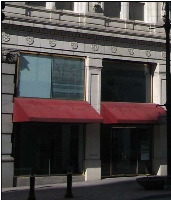
Use traditional awning locations, materials, and designs on new construction as used on historic buildings. Shed canvas awnings that fit storefront openings are recommended (136 S Main Street).
