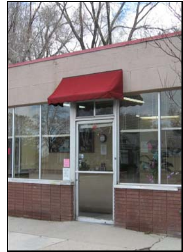
Simple shed roof canvas awnings are also appropriate for entrances such as at 442 N 300 West.
