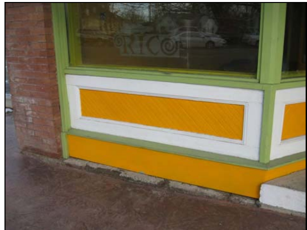
Original wood bulkheads such as those at 361 N Main Street (left) and 779 S 500 East (right) are significant parts of historic storefronts.
