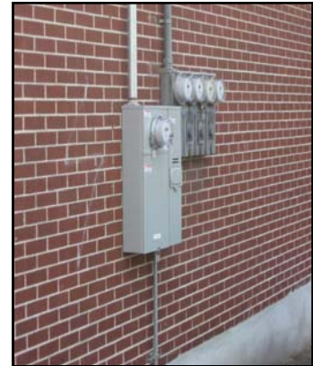
Meters at 39 N 'I' Street are correctly placed on a non-primary elevation.
