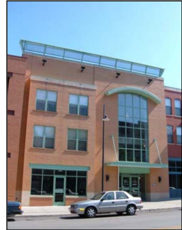
New contemporary construction such as illustrated above should have windows and storefronts in keeping with traditional designs and detailing.
