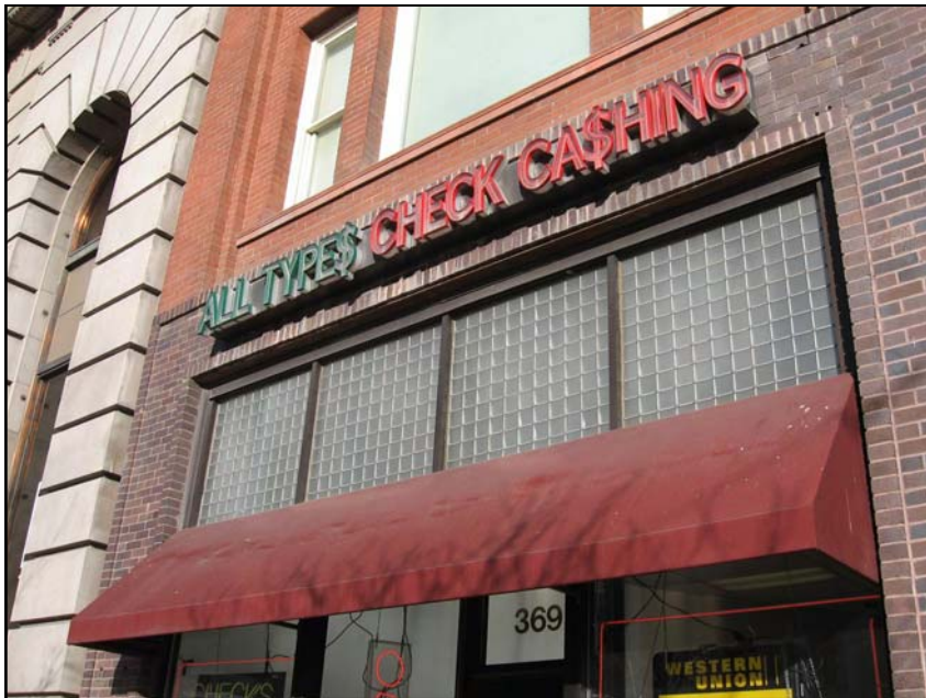
The distinctive Luxfer glass transom on the New Grand Hotel at 369 S Main Street is intact and not concealed.
