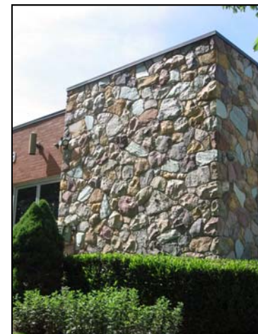
This stone veneer corner bay is at 633 E South Temple Street and was built in 1960.
