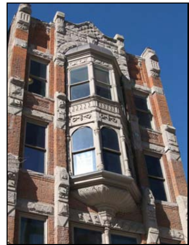
A combination of brick and decorative stone are featured on the upper façade of Daft Block, 128 S Main Street.
