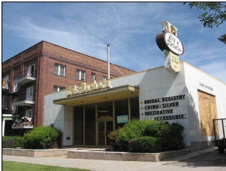
Another example of an enframed window wall plan is the Felt-Buchorn Building at 445 E South Temple Street. Built in 1959, it displays a continuous surround of porcelain steel panels which frame the display windows and entrance.
