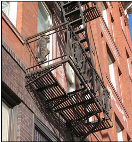
Historic fire escape at 379 S Main Street.
