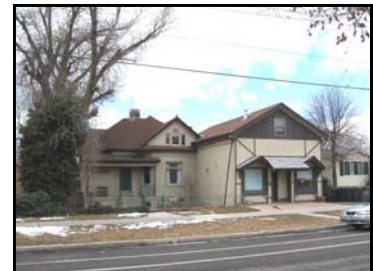
Although the commercial section has been altered, it remains a good example of a house store design (537 N 200 West).
