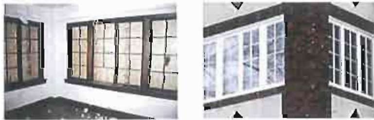
The historic wood windows (left) were repaired and exterior storm windows added (right). This approach meets the Standards for Rehabilitation. Photos: NPS files
