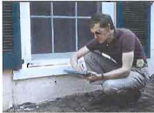
Window condition assessment preceding repair work.
