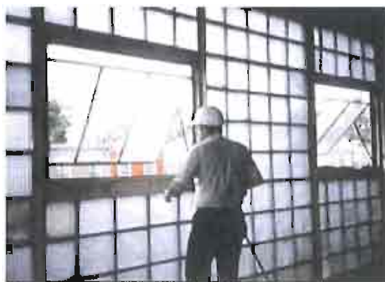
Preparing historic steel windows for repairs and re-finishing.
