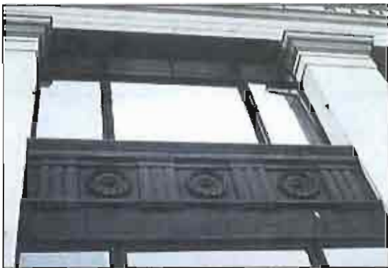
Historic steel sash can be fitted with dual glazing to improve thermal efficiency. Photo: NPS files.
