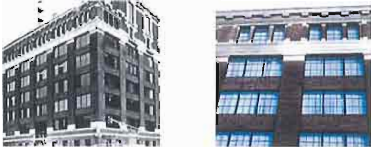
Above: Replacing these existing incompatible replacement windows (left) with similar units would not meet the Standards. New windows installed in a rehabilitation project should be compatible with the historic character of the building. In this case, new windows (right) that convey the general appearance of industrial steel windows that were historically on the building were the appropriate choice for this building. Photos: NPS files
