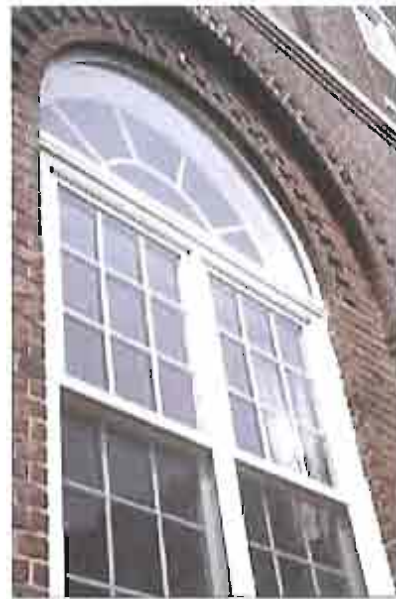
Newly painted double-hung wood windows.
