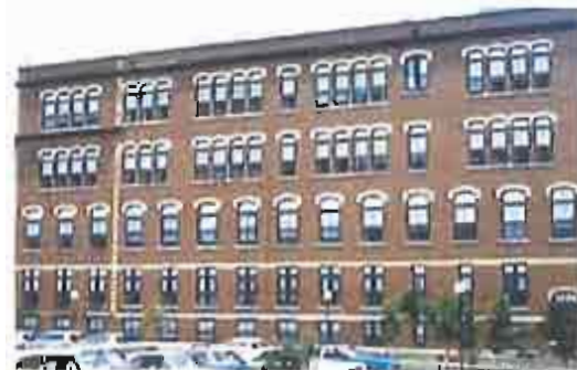
Distinctive window design on 19th century building.
