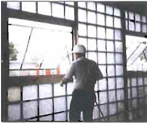
Maintaining historic steel windows for continued use is always recommended. Photo: NPS files.
