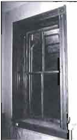
Following the relatively simple repairs, the window is weathertight, like new in appearance, and serviceable for many years to come. Photo: NPS files.
