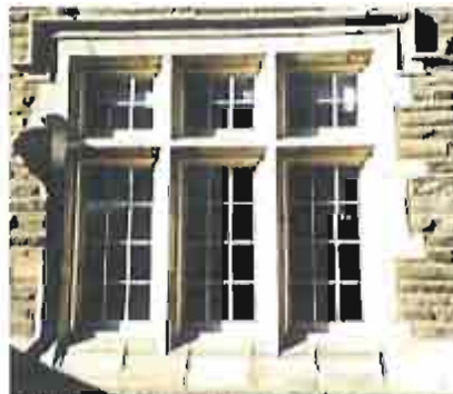
Lower window sash replaced, based on physical documentation.
