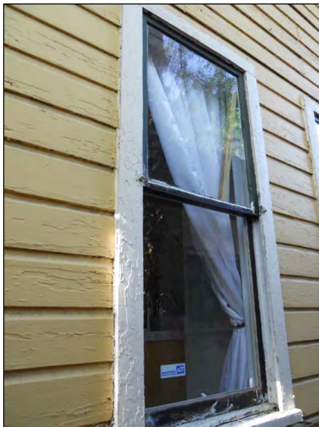
Subject Window #5 (Westernmost Window)
