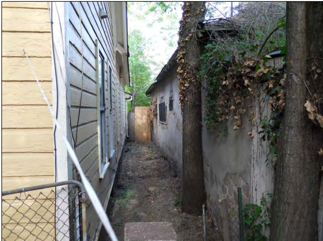
View of Subject Windows from Rear
