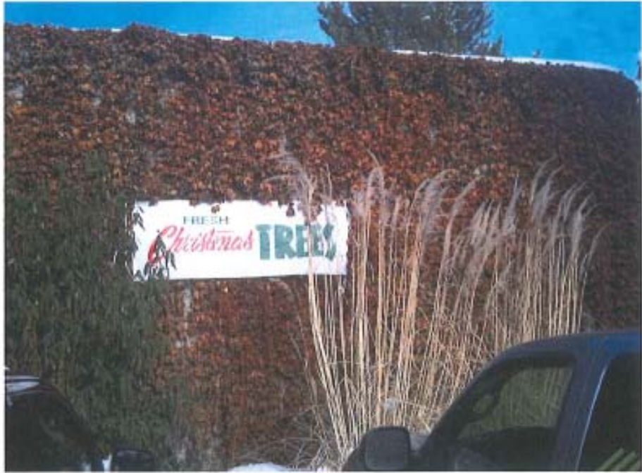
South Elevation Designated as "Reception Center"
