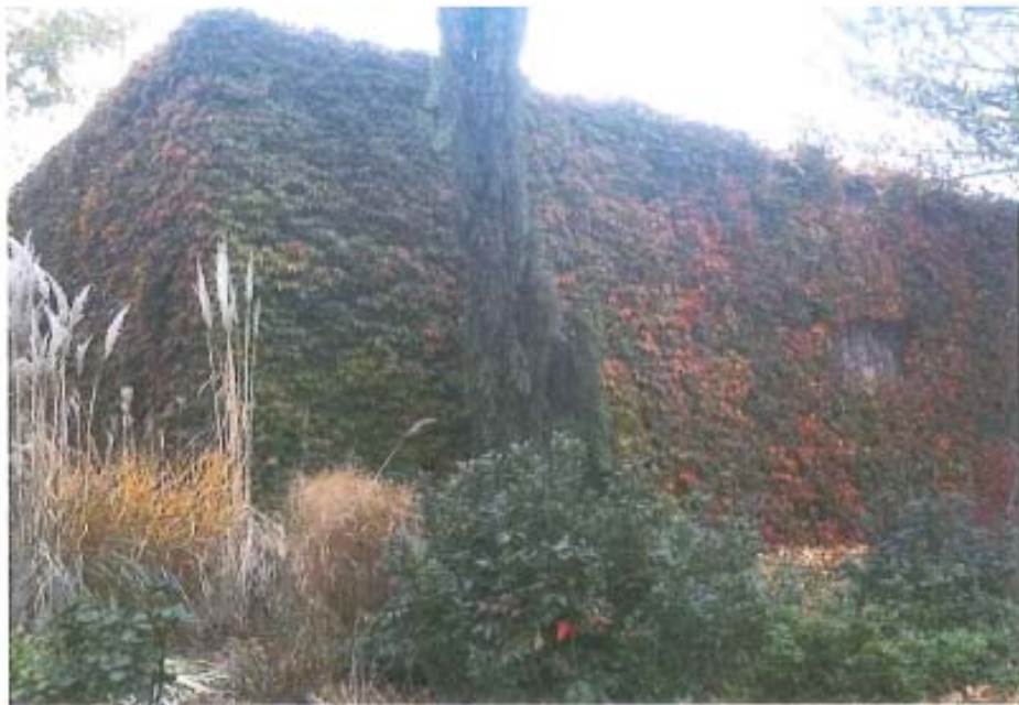
South East Corner of Building Designated as "Reception Center"
