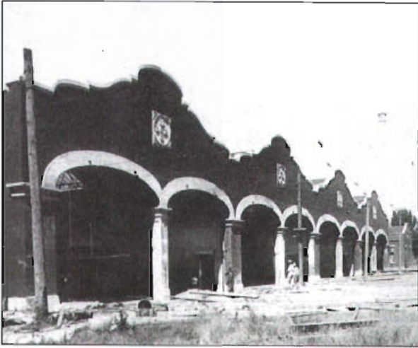
Trolley Square under construction.
