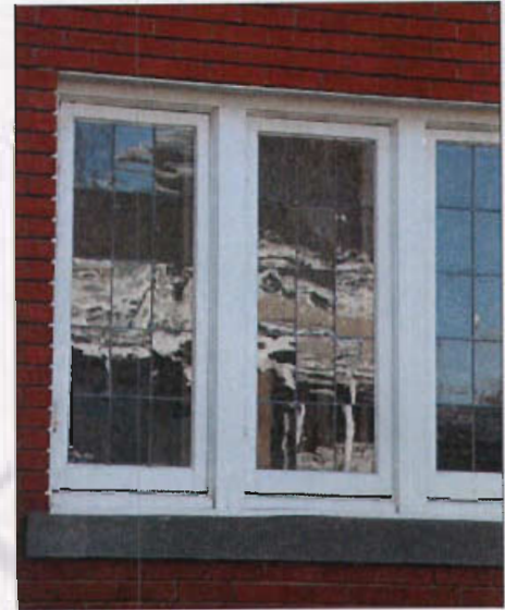
When a window is to be replaced, the new one should match the appearance of the original to the greatest extent possible.
