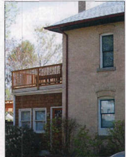
Small rear addition of individual design and materials, though in keeping with the design character and materials of the original building.
