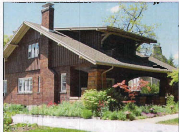
Bungalow porch with battered (tapered) columns.
