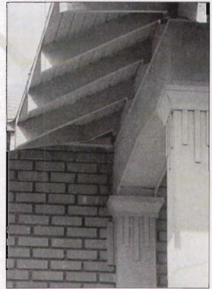
Porch columns with Arts and Crafts details, rafter tails.
