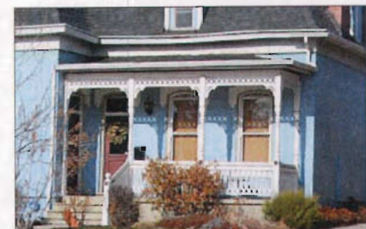
Wood detailing on porches such as this jigsaw ornamentation, or detailed balustrade, should be preserved.
