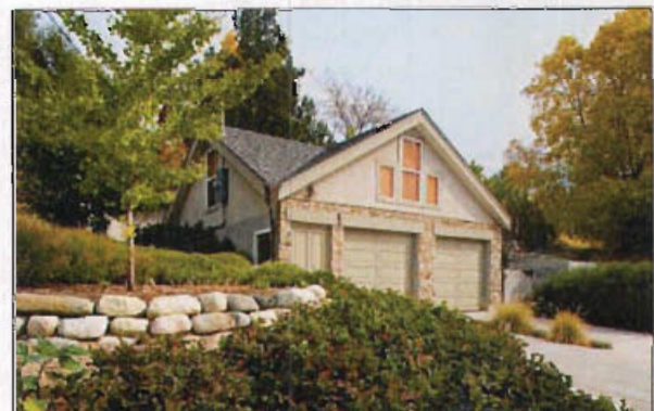
Recent garage with accommodation above designed to reflect scale and character of the context.
