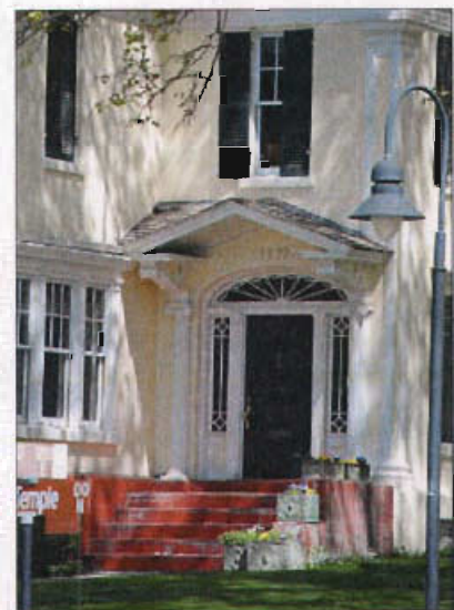
The doorway, the proportions of opening and framework, sidelights and transom/fan lights, porch hood, decorative details, and the design of the door itself, combine to celebrate the entrance.
