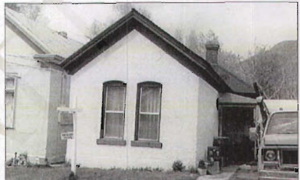
This is an unusual example of a front facing Greek Revival style building in the Capitol Hill Historic District. Despite the rarity of its orientation, its massing, stucco finish, pronounced wood cornices and fascia are clearly in keeping with this style and period.
