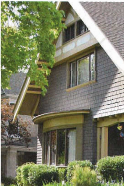
Color can be used to complement the texture and qualities of the materials and detailing.
