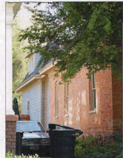
This recent addition reflects the design traditions of the original with a change in material to siding. The change from original to new is emphasized by a break in the wall plane and roof plane.
