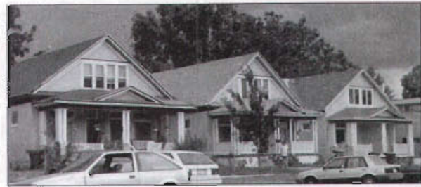
The uniform setback of these vernacular structures provides a sense of alignment and the porches provide a consistent orientation to the street.
