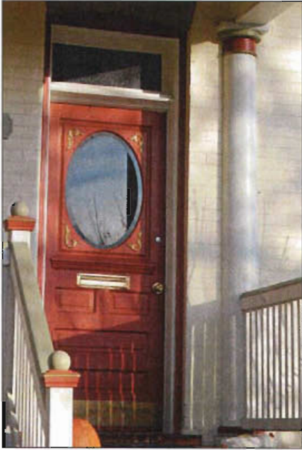
When a historic door or its components are damaged, repair them and maintain their general historic appearance.
