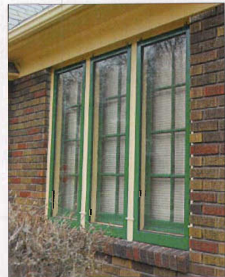
External wood framed storm windows designed to fit the primary framework of the original.
