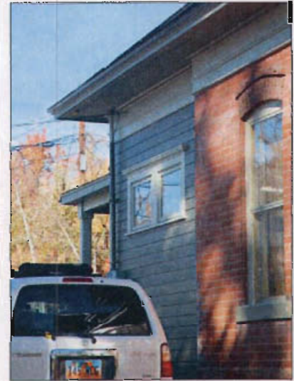
Rear addition reflecting form and scale and distinguished by wall plane, fenestration, detail and materials.
