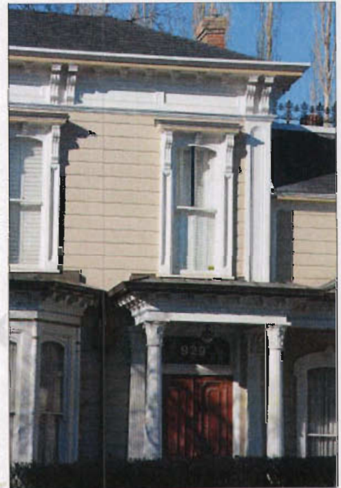
The paneled door of this important Italianate building is framed with intricately detailed full and engaged columns supporting a covered porch.
