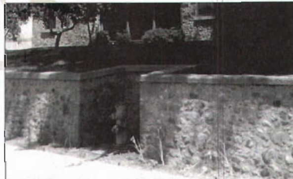
Retaining walls provide visual interest to the street, and serve as distinct character-defining features. This characteristic should be preserved.
