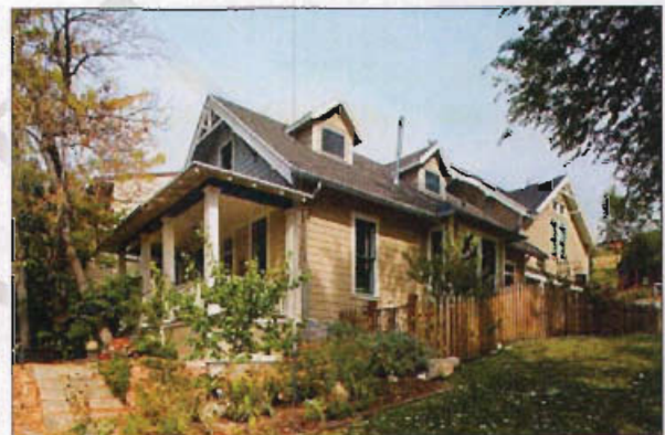
The rear addition steps back from the side facade of the house and integrates two story accommodation in a manner which does not dominate the original building.
