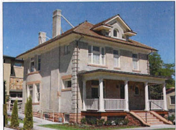
The Stanley F Taylor building, a residence dating to c.1906. was recently seismically upgraded as part of an extensive rehabilitation.
