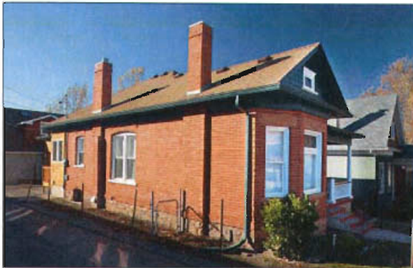
Small staggered rear addition continuing the axis and eavesline of the residence and distinguished by design and materials.
