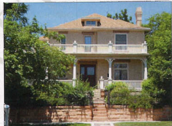
The form, construction, detailing and materials of a retaining wall may complement both the architectural setting and character of the neighborhood.
