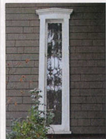
Ornamental trim around historic windows should be preserved.
