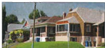
Enclosing a front porch will significantly compromise the architectural integrity of the house.
