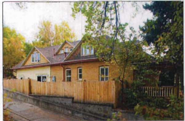
Addition to the rear of this house adopts the scale and design of the original and is clearly identified by a change in materials.
