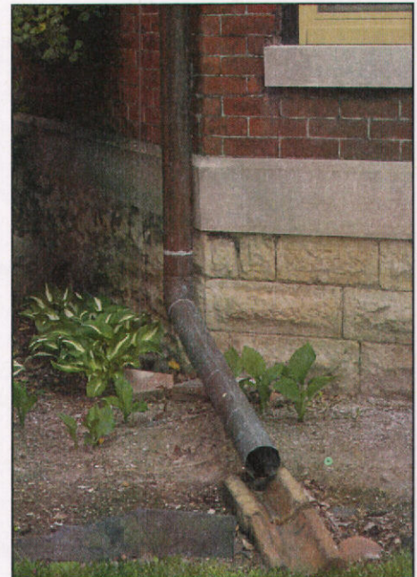
Appropriate downspout and splash block.
