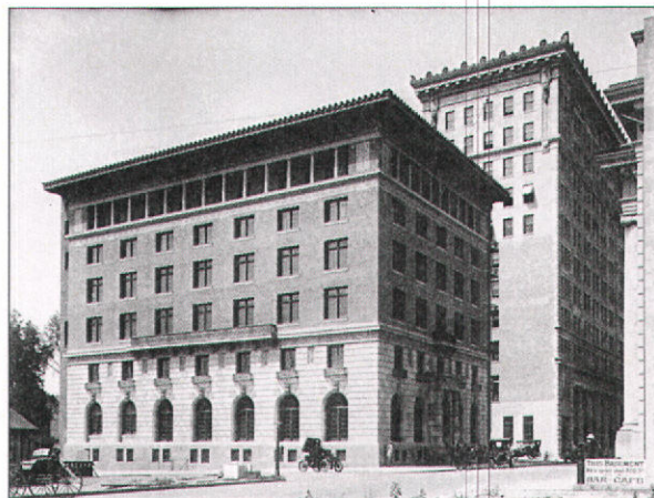
The Commercial Club Building (1908) borrows its architectural detailing and overall style from the Second Renaissance Revival style. (Courtesy Utah State Historical
