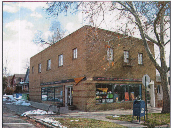
The building at 702 E 3rd Avenue (ca. 1940) was designed with simple detailing and has rectangular steel casement windows and original display windows.
