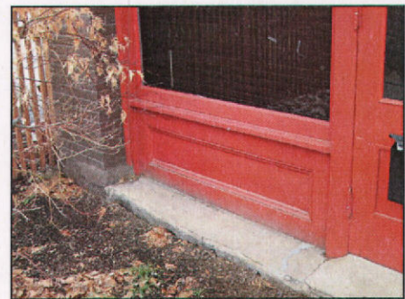
Original wood bulkheads such as those at 361 N Main Street are central elements of historic storefronts.
