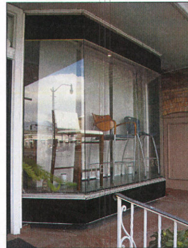
The Carrara glass is a distinctive characteristic of the storefront at 432-434 E South Temple Street.
