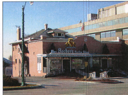
The storefront was an early addition to the building at 434 E South Temple Street.
