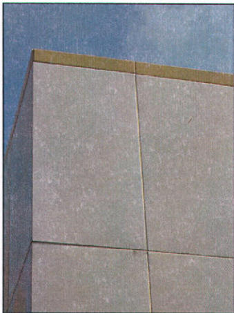
Porcelain panels on the Felt-Buchhorn Building at 445 E South Temple Street.
