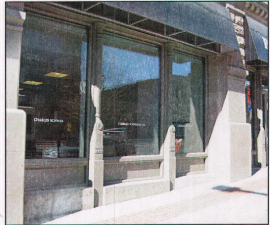
Cast iron columns embellish the window frame on the Brooks Arcade at 268 S State Street.
