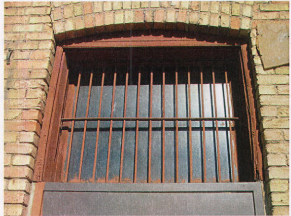
Security bars are more appropriate on side or rear façades.
