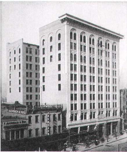
Kearns Building at 130-142 S Main Street. (Courtesy Utah Historical Society)
