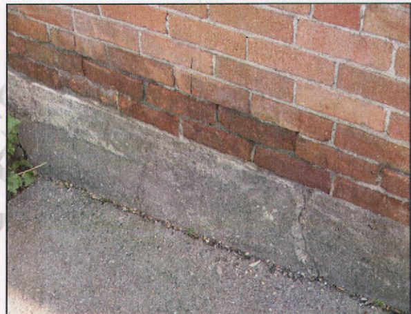
A concrete foundation at 422-426 N 300 West.
