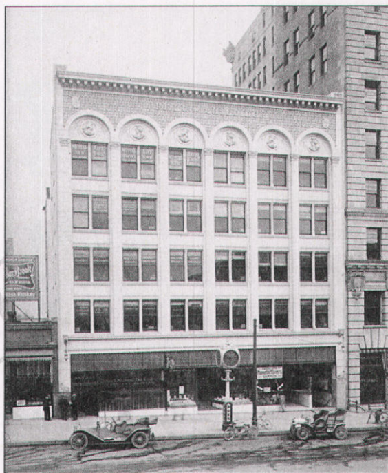
The Felt Building (1910) at 339 S Main Street displays early use of terra cotta as a decorative element. (Courtesy Utah State Historical Society)
