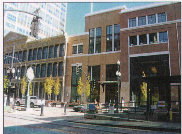
A step back provides a transition between the historic ZCMI storefront and the infill construction.
