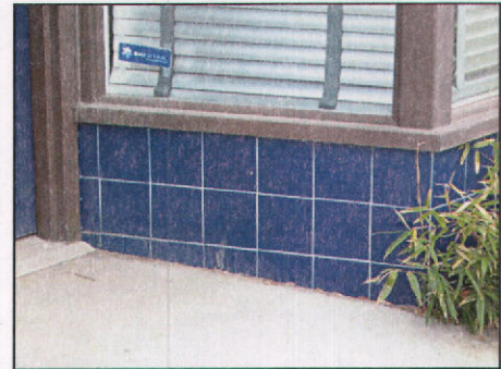
An original tile bulkhead at 422-426 N 300 West.
