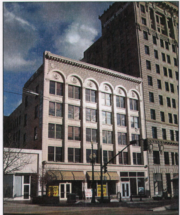
The Felt Building at 335-339 S Main Street (1909) has a separate storefront zone and unified upper façade. The building is distinguished by its glazed terra-cotta and arched panels below the cornice.
