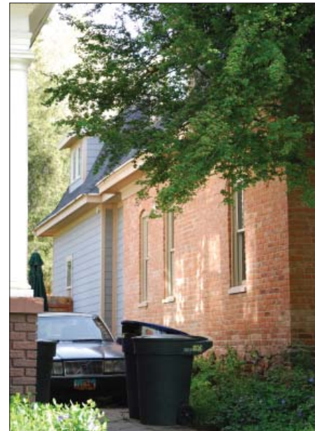
This recent addition reflects the design traditions of the original with a change in material to siding. The change from original to new is emphasized by a break in the wall plane and roof plane.
