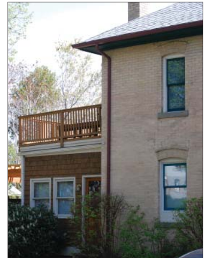
Small rear addition of individual design and materials, though in keeping with the design character and materials of the original building.
