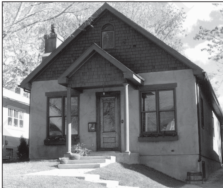
This house, constructed in 1994, blends in well with the traditional Avenues streetscape because of the fenestration pattern, the roofline and the materials. In addition, the porch compliments the design of the house and serves as an important transitional element between the house and the street.
