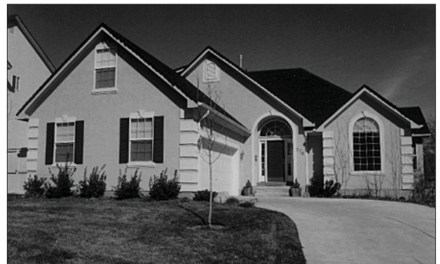
This Avenues house was constructed in 1993. The builders rotated the garage so that the doors would not be a dominating streetscape feature, thus maintaining the traditional “pedestrian-friendly” quality of the street.
