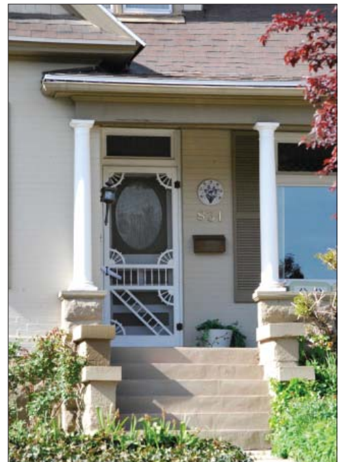
In this case the storm door and screen provide a decorative addition to the original design and detail of the door.
