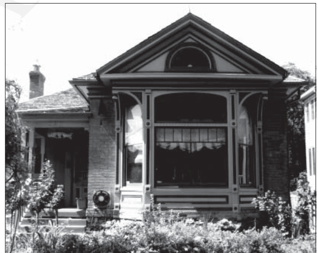
This Victorian Eclectic structure exemplifies the visual and architectural richness of buildings in the Capitol Hill district.
