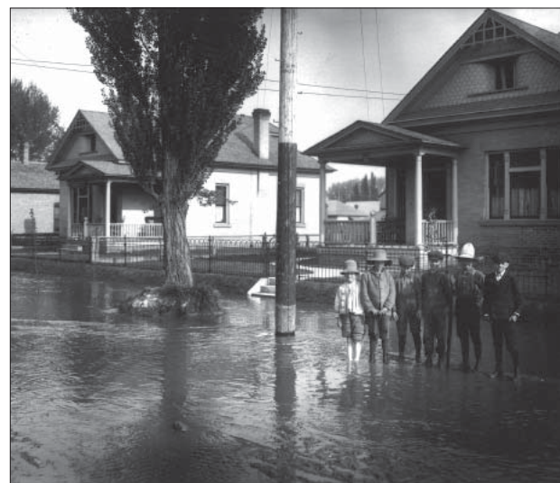
Decorative shingles, window trim and porch detail of the Victorian era.
