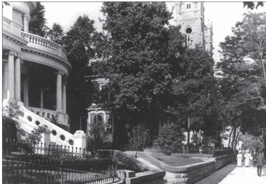
Looking southeast along South Temple from 5th West in 1918: stone retaining walls and cast iron fences define the sidewalk edge. Extensive porch detailing provides a strong sense of orientation to the street.
