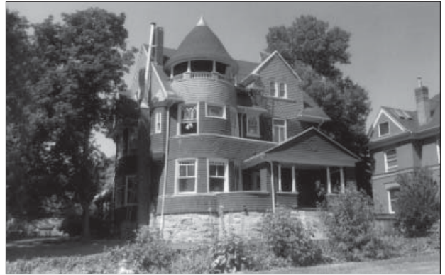
Complex, asymmetrical forms compose many of the Victorian-era structures in the Avenues.
