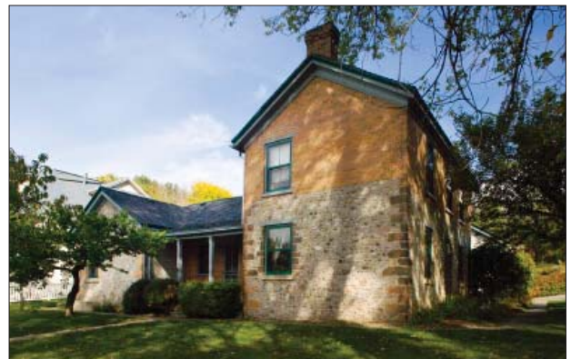
Second story addition to a historic plan form, closely reflecting the original design and identified by a change in materials.
