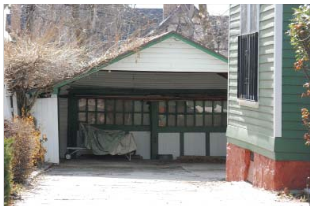
Early garage sliding door arrangement with later alterations.
