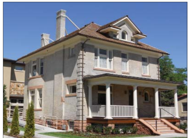
The Stanley F Taylor building, a residence dating to c.1906, was recently seismically upgraded as part of an extensive rehabilitation.
