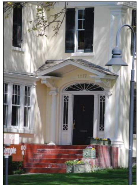
The doorway, the proportions of opening and framework, sidelights and transom/fan lights, porch hood, decorative details, and the design of the door itself, combine to celebrate the entrance.
