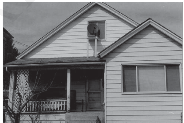
Replacement windows that do not match historic dimensions are inappropriate.
