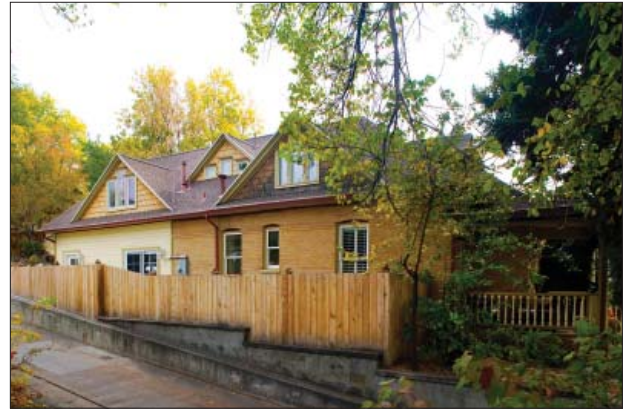
Addition to the rear of this house adopts the scale and design of the original and is clearly identified by a change in materials.
