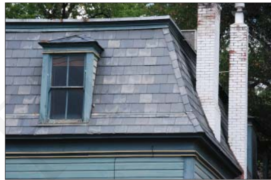
Natural slate is rare in the city and is the most durable of traditional roof materials, usually requiring only piecemeal replacement of damaged individual slates.
