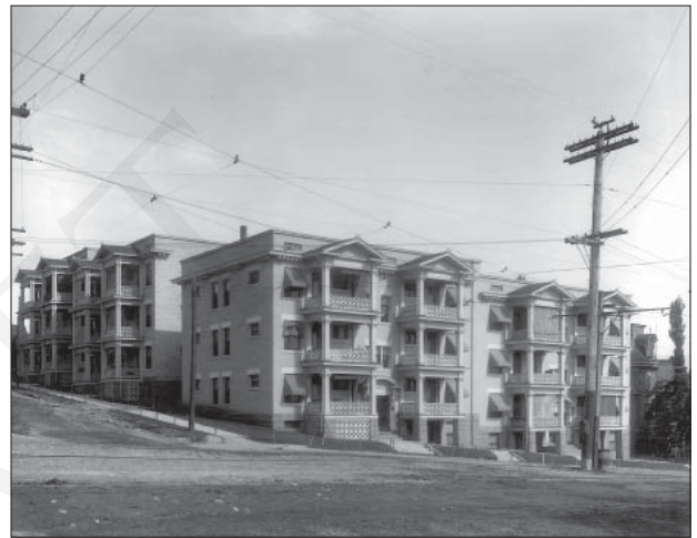
The Kensington Apartements were constructed about 1905, and represent a type of apartement known as a “walk-up.”
