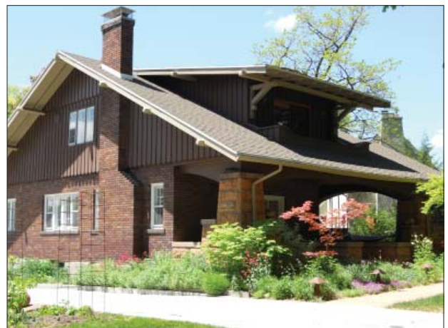
Bungalow porch with battered (tapered) columns.
