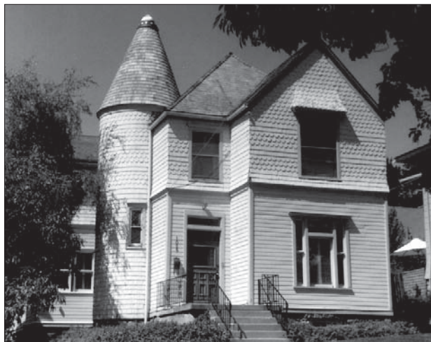
A two story frame structure of the Victorian era. The porch has been altered.
