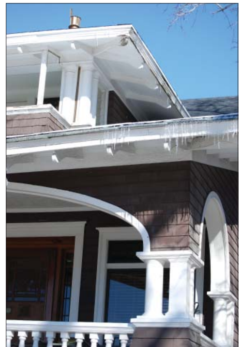
Features such as window hoods, brackets and columns are often associated with particular styles and therefore their preservation is important.
