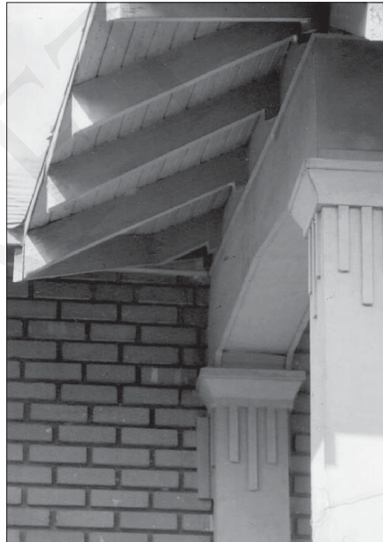
Porch columns with Arts and Crafts details, rafter tails.
