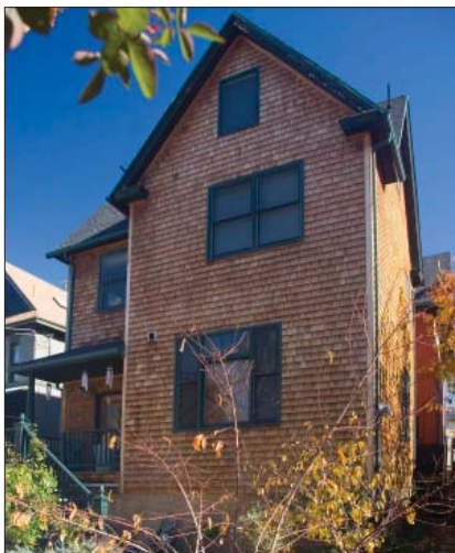
Front and rear views of substantial rear addition adopting original design cues.
