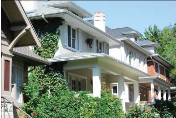
Square columns in various designs create detailed variety and a visual richness in this complementary series of full-width porches.
