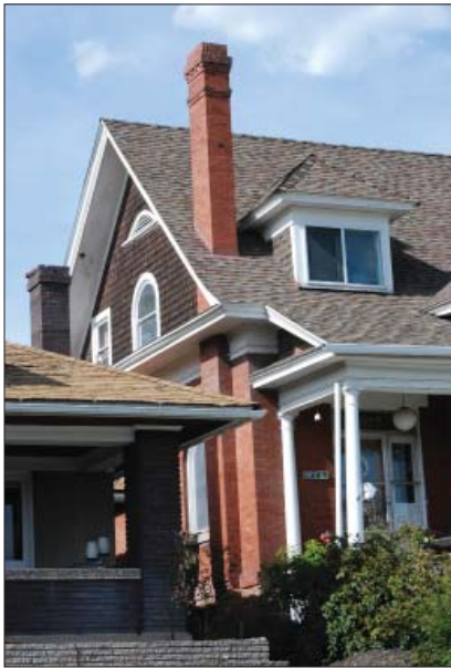
Asphalt Shingles - Appropriate for: All types.
