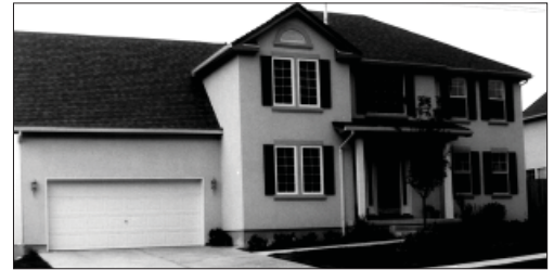
This attached garage is minimized by setting it back several feet from the wall plane of the house.
