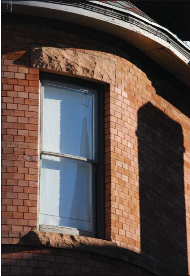
The appearance and integrity of the original masonry can be successfully maintained through appropriate repair.
