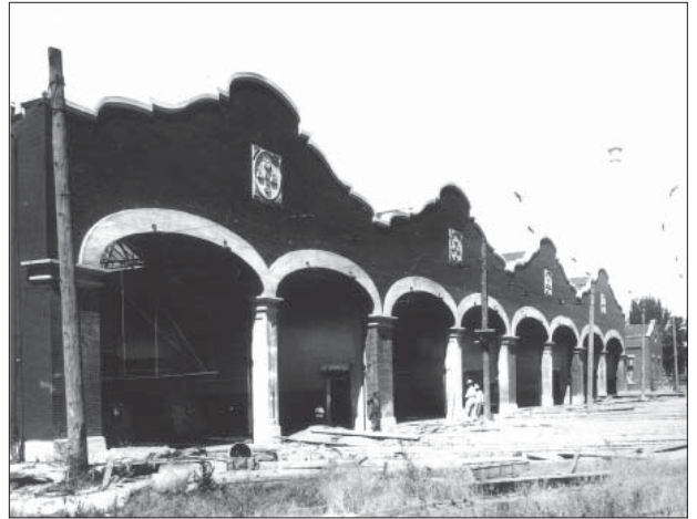
Trolley Square under construction.
