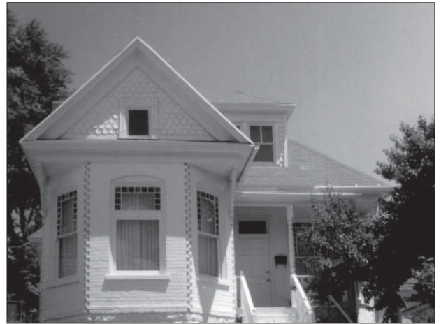
Decorative shingles in the gable, turned posts on the porch and the interlocking brick bay of this house exhibit the high degree of craftsmanship and attention to detail that mark many houses in the neighborhood.
