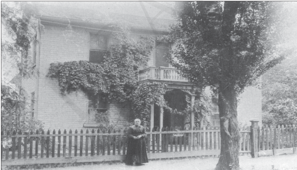
Sarah Hancock Beesley in front of the home of Ebenezer Beesley on 200 North Street. Italianate posts support a railing with turned balusters for a second floor porch in the background. Also note the wooden picket fence.
