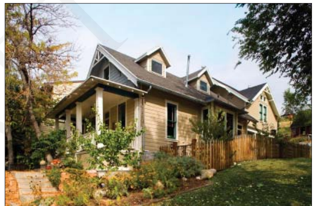
The rear addition steps back from the side facade of the house and integrates two story accommodation in a manner which does not dominate the original building.
