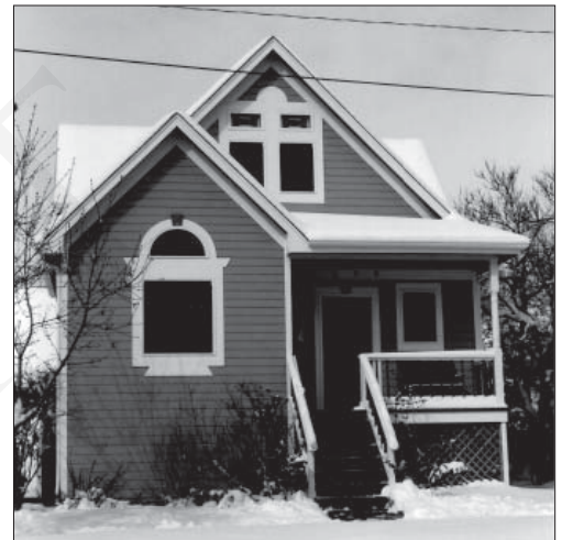
The proportions of window and door opening should be similar to those of historic buildings in the area.
