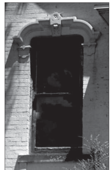
Ornamental trim around historic windows should be preserved.
