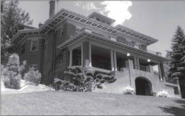
The “Woodruff-Riter-Stewart Home” at 93 East Second North Street is an example of the variety of architectural styles that can be found in the Capitol Hill Historic District.
