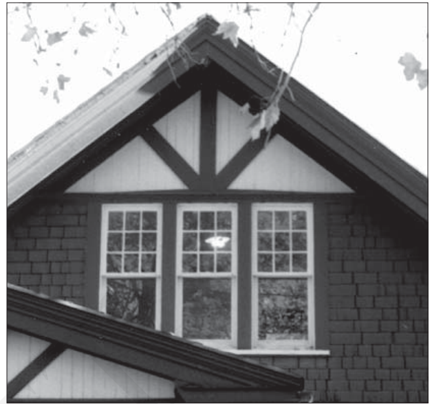
When a window is to be replaced, the new one should match the appearance of the original to the greatest extent possible.
