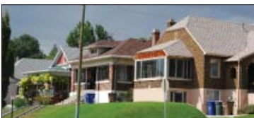
Enclosing a front porch will significantly compromise the architectural integrity of the house.
