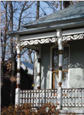
This porch reconstruction closely followed photographs of the original.
