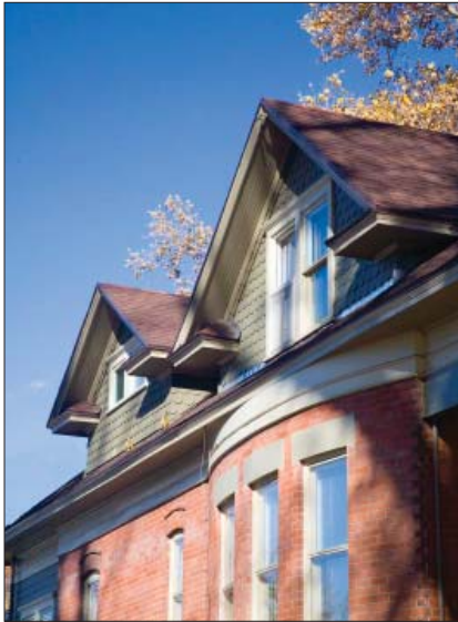
Rear addition with second story space above designed to complement and be distinguished from the original house.
