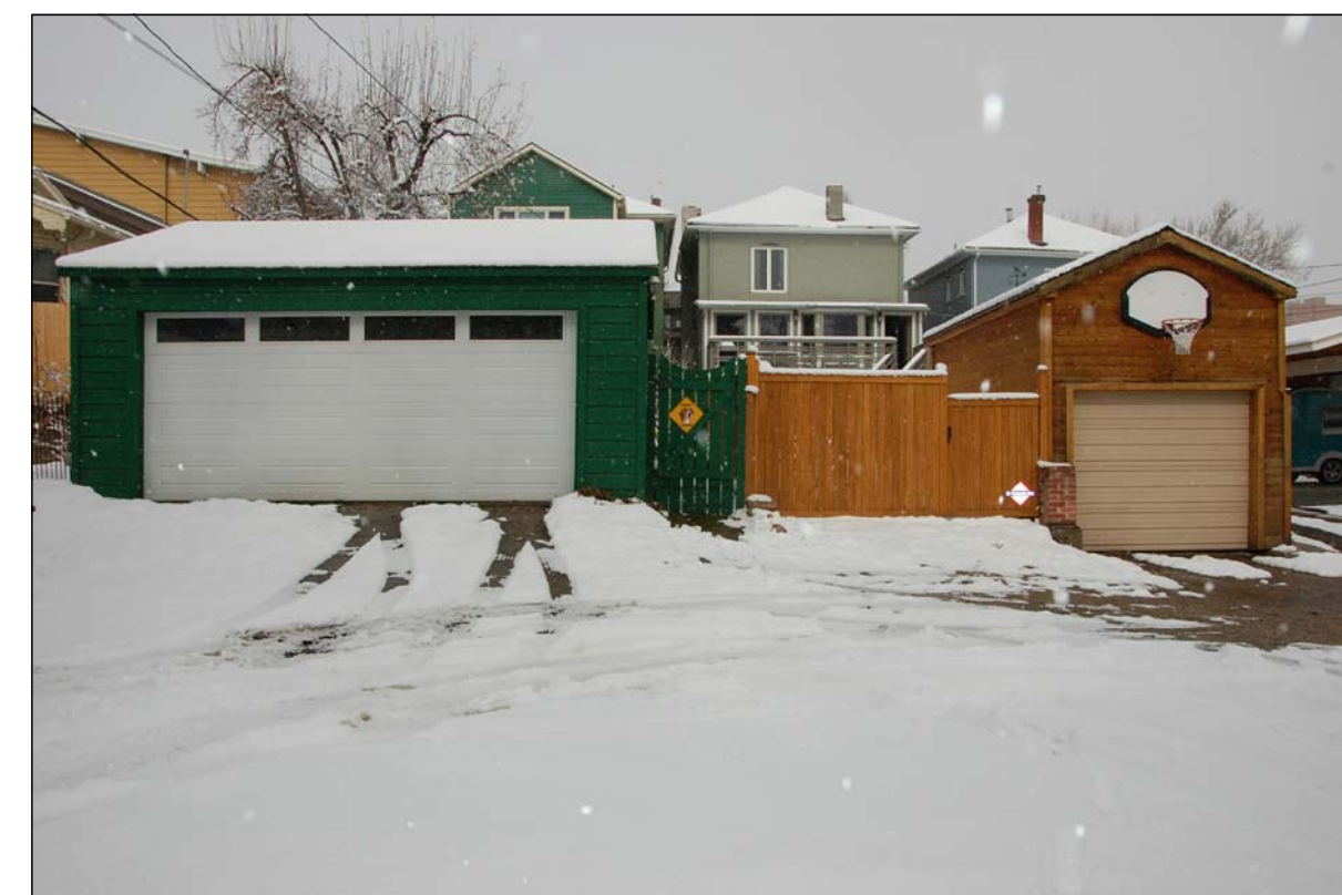
NORTH ELEVATION OF RIGHT OF WAY
