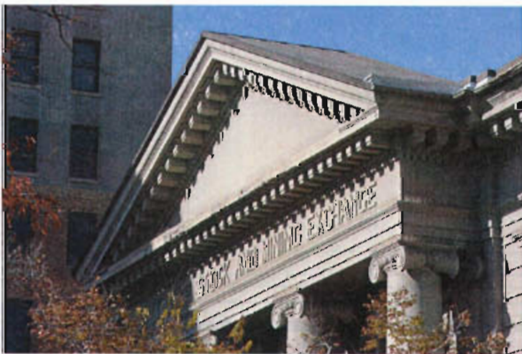
Classical detailing at 39 Exchange Place.
