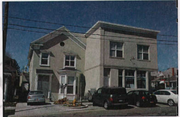
The building (ca. 1906) at 187 N 'E' Street is a good example of a house store.
