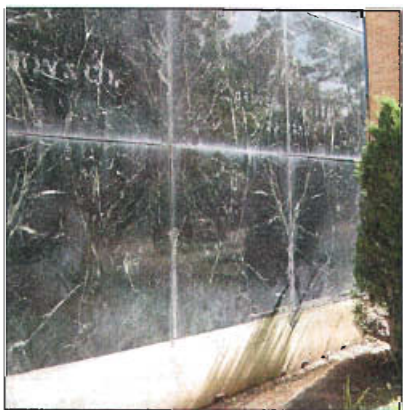
Marble paneled veneer on the main façade at 641-645 E South Temple Street.
