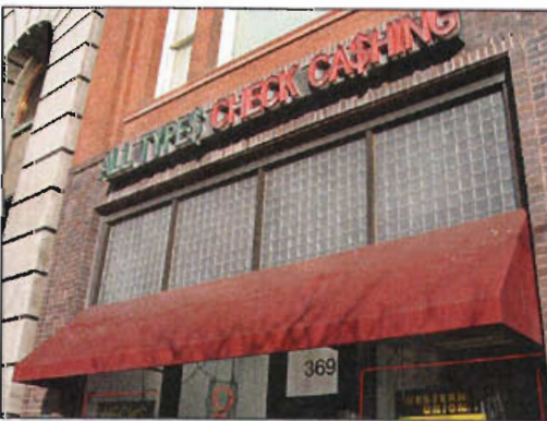
The distinctive Luxfer glass transom on the New Grand Hotel at 369-379 S Main Street is intact and not concealed.
