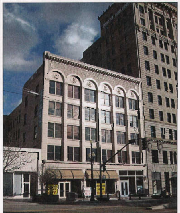
The Felt Building at 335-339 S Main Street (1909) has a separate storefront zone and unified upper façade. The building is distinguished by its glazed terra-cotta and arched panels below the cornice.
