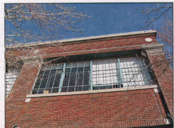
Steel frames with multiple lights are characteristic of many historic buildings.
