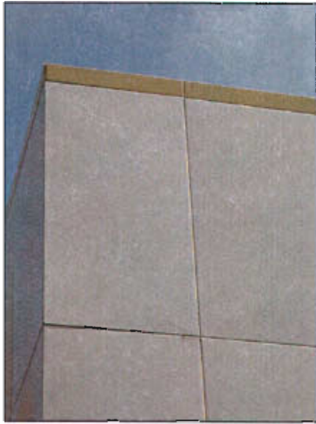
Porcelain panels on the Felt-Buchorn Building at 445 E South Temple Street.
