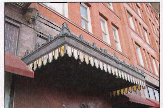
The distinctive canopy on the New Grand Hotel at 369-379 S Main Street defines an entrance and provides cover.
