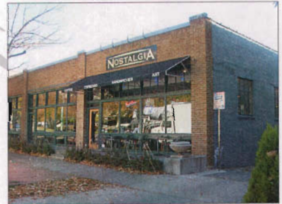
Most historic commercial buildings were designed with flat or sloping roofs.
