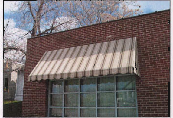
This shed awning provides façade detailing to the building at 736 N 300 West.
