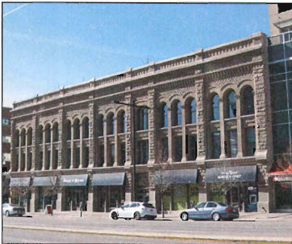
Rounded arches and textured masonry are common features of the Richardsonian Romanesque style.
