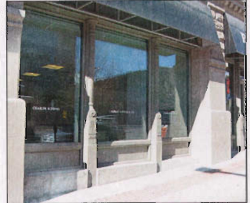
Cast iron columns embellish the window frame on the Brooks Arcade at 268 S State Street.
