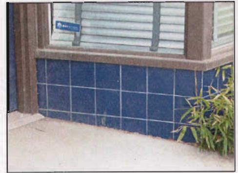
An original tile bulkhead at 422-426 N 300 West.
