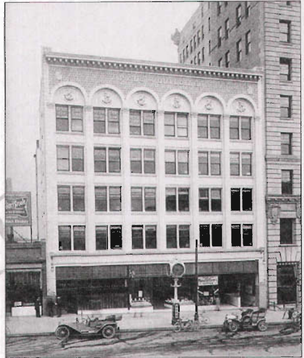
The Felt Building (1910) at 339 S Main Street displays early use of terra cotta as a decorative element. (Courtesy Utah State Historical Society)
