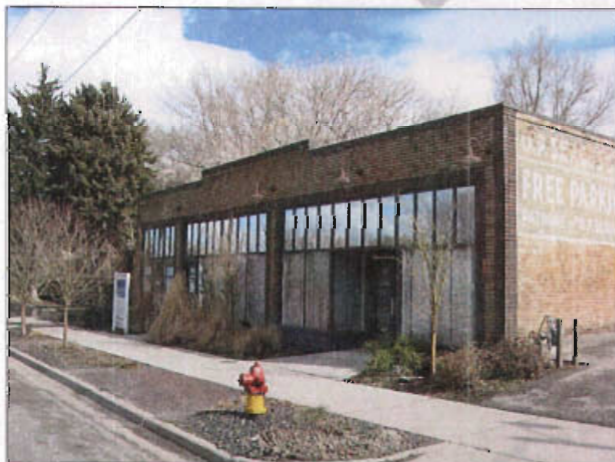
The O. P. Skaggs building at 422-426 N 300 West (1926) is a good example of the type of commercial buildings built along 300 West.
