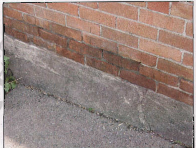
A concrete foundation at 422-426 N 300 West.
