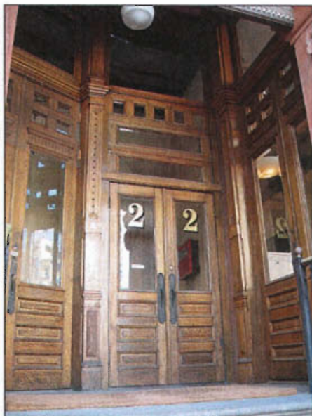
Wood doors on Utah Commercial & Savings Bank Building at 22 E 100 South.
