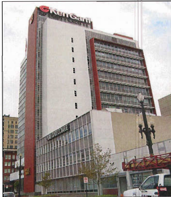
The First Security Bank Building at 405 S Main Street (1955) features an exterior curtain wall of glass, aluminum, and enameled porcelain panels.
