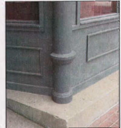
Decorative metal detailing is a significant characteristic of the street façade at 68 N 'K' Street.
