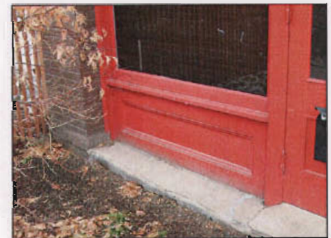
Original wood bulkheads such as those at 361 N Main Street are central elements of historic storefronts.
