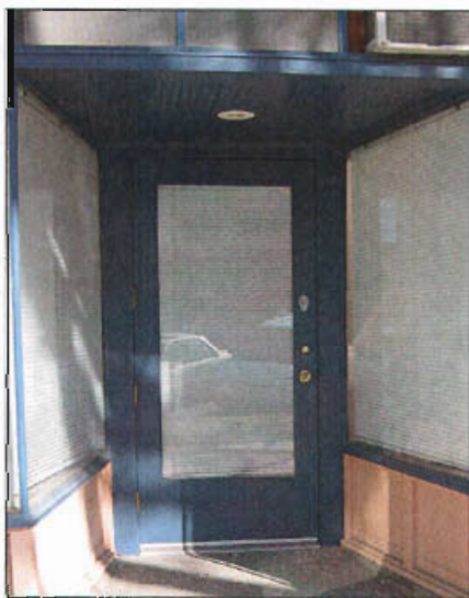
Salt Lake City's commercial buildings have a variety of doors and entrances.
