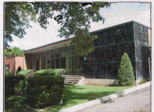
The building at 641-645 E South Temple Street (1957) displays black marble panels and a sleek exterior.
