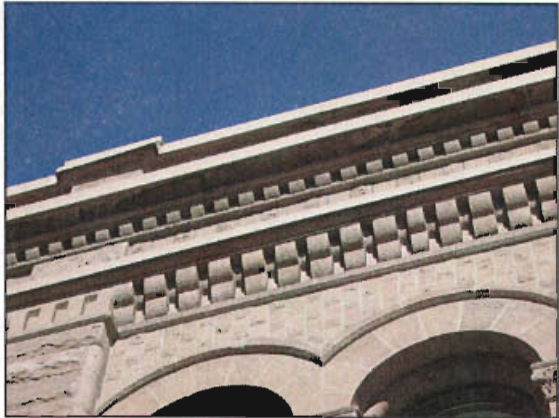
A stone cornice on the Brooks Arcade at 268 S State Street.
