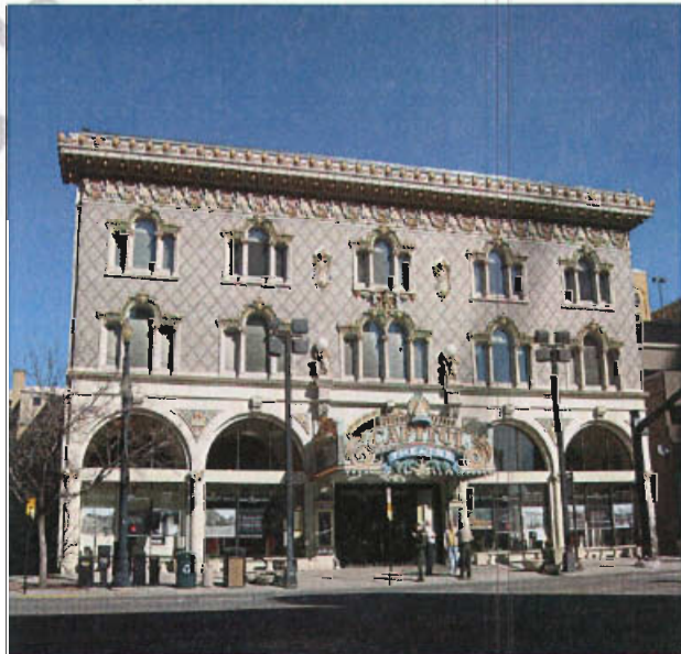
The Orpheum (Capitol) Theatre (1913) reflects the arcaded block building type and Renaissance Revival architectural style. The building displays terra cotta on the main façade and has been restored into a multi-use theater building.
