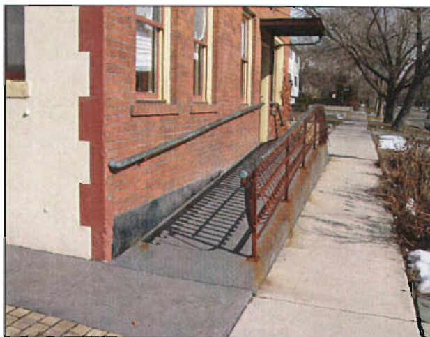
This accessibility ramp is compatible with the historic building both in scale and materials.
