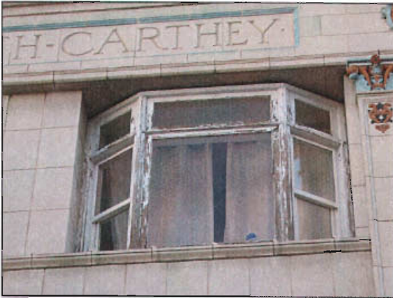
Regular maintenance will improve the longevity of a historic window.
