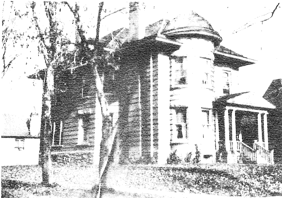
Figure 2: Main structure circa 1915 showing fences have deteriorated and been removed. Not the brick detail which will be carried onto the addition. Trees on the property are more mature and some have been removed since 1905.
