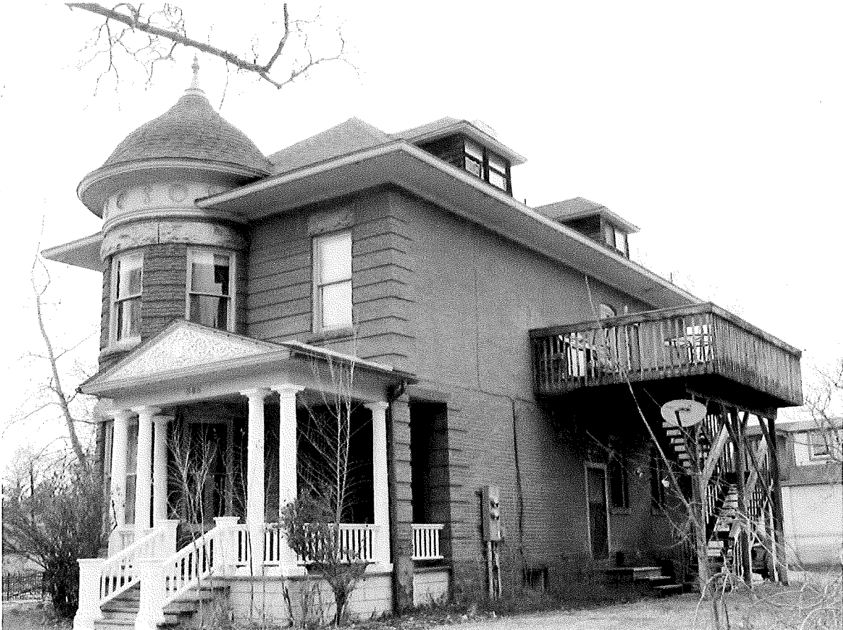
Figure 7: Existing front porch (left) restored to original character present in 1905. This design will be used to replace the 1960's era two story deck, with the exception that the second story will be flat deck space.
