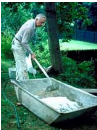
The dry materials must be mixed thoroughly before adding water to make the stucco. Photo: NPS files.
