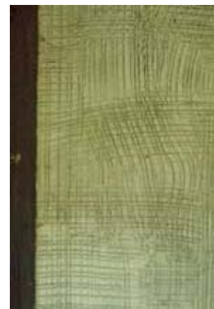
The final finish coat will be applied to this scratch coat. Photo: NPS files.
